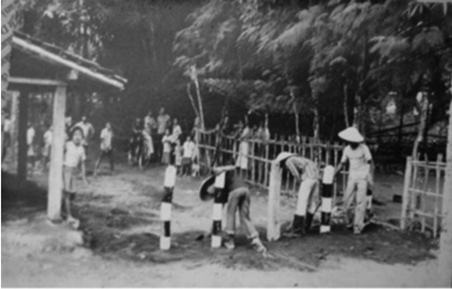
Fig. 3.2 Concrete blockages setting (source: Sucoro)
