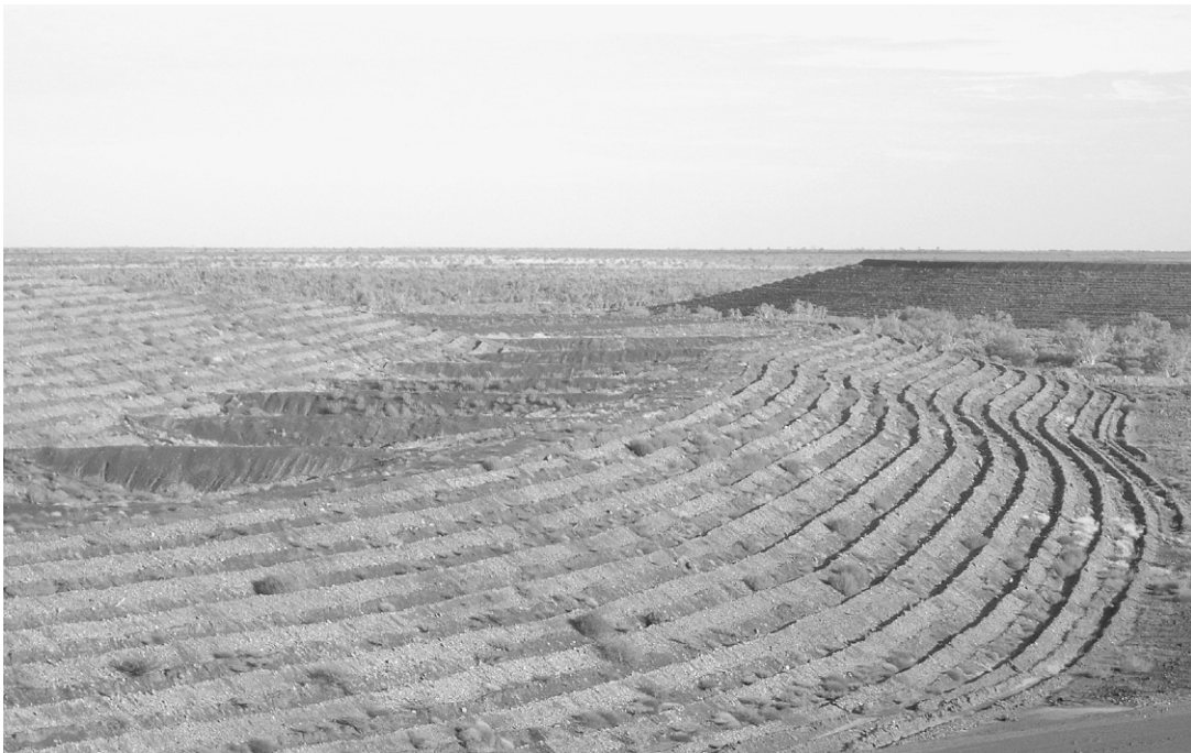
FIGURE 7.5. An example of a bank-and-trough system constructed on a low-angled TSF wall. Natural landforms can be seen in the background. Photograph courtesy of Roger Potts.
