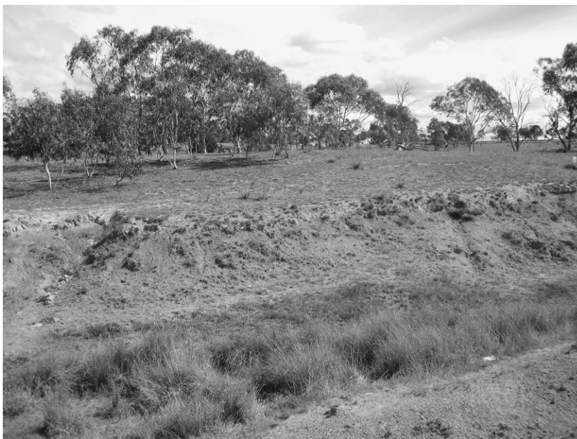
FIGURE 15.2. A channelized ephemeral drainage line on a hillslope shows signs of rapid over-bank flow (bare side-walls) but a stabilizing grassy floor. This implies that the restoration solution involves reducing flow rates from the hillslope above the channel, rather than within the channel itself.
