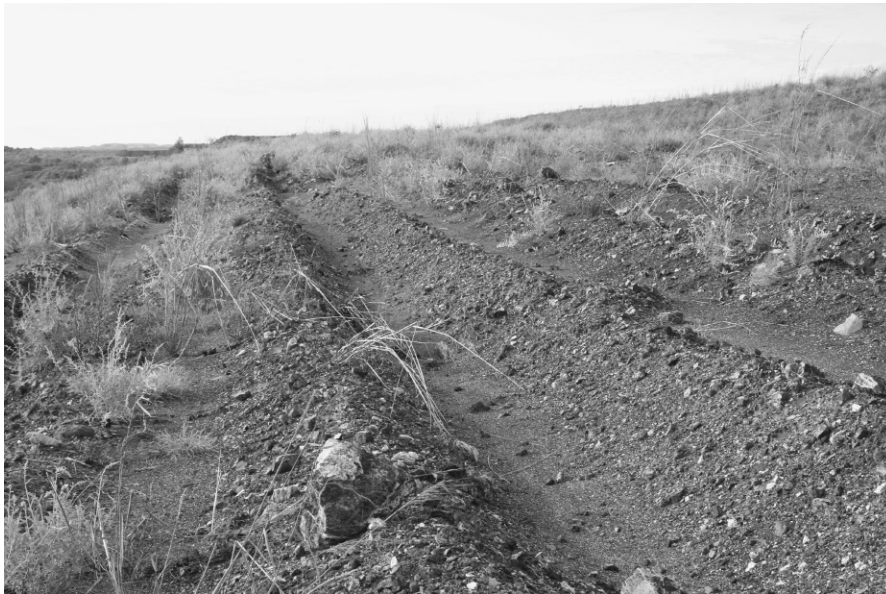
FIGURE 3.2. A landscape where piles of waste rock were reshaped to have minimum slopes. The reshaped surface was then deep-ripped to create banks and troughs.
