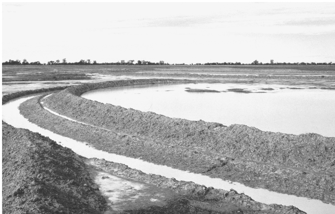
FIGURE 5.13. An example of a water-ponding bank constructed on a scald. The bank is successfully retaining water after a rain event. Photograph courtesy David Eldridge.
