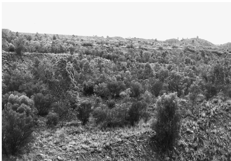
FIGURE 8.11. An example of a landscape reformed into small catchments (about 50 m from rim to rim) from spoil heaps produced by open-cut coal mining.
