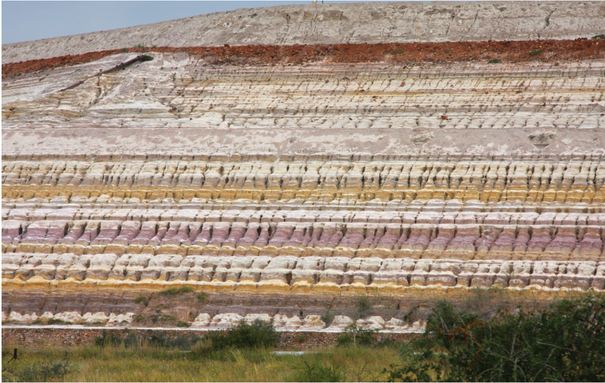
PLATE 7.2. Wall of a tailings storage facility with distinctive bands of different tailing materials.
