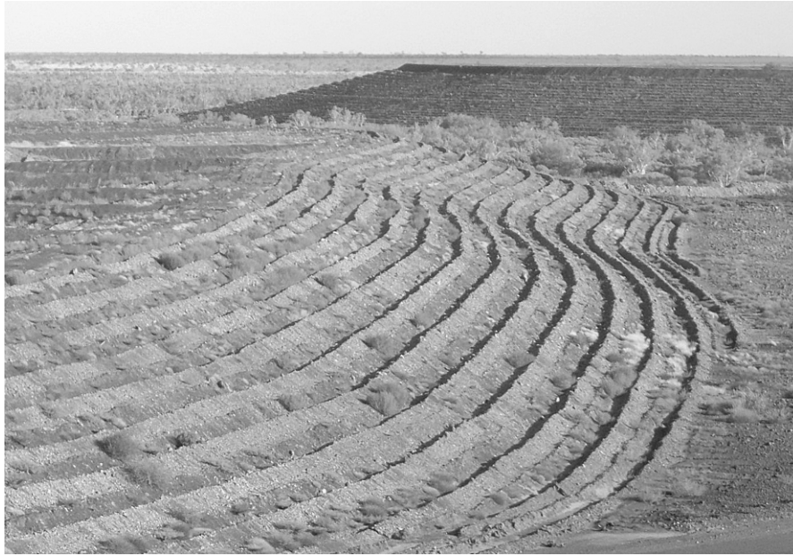
FIGURE 3.3. A landscape reformed from piles of waste rock into one with sloping sides and a series of banks and troughs shaped along slope contours.
