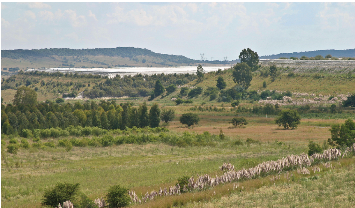
PLATE 7.3. Plantations located at the base of tailings storage facilities.
