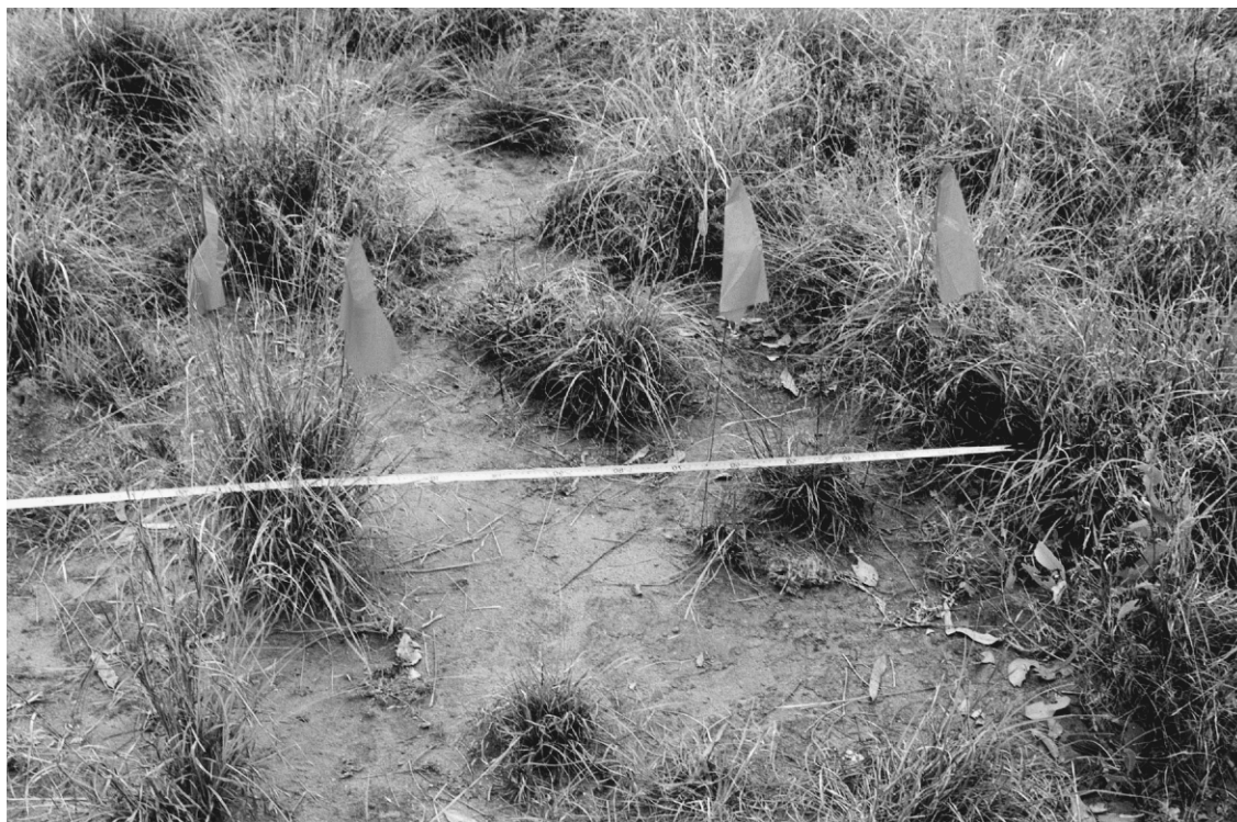
FIGURE 7.8. Signs of surface erosion and compact physical crusts are evident between grass clumps along a transect being monitored on the walls of a rehabilitated TSF.
