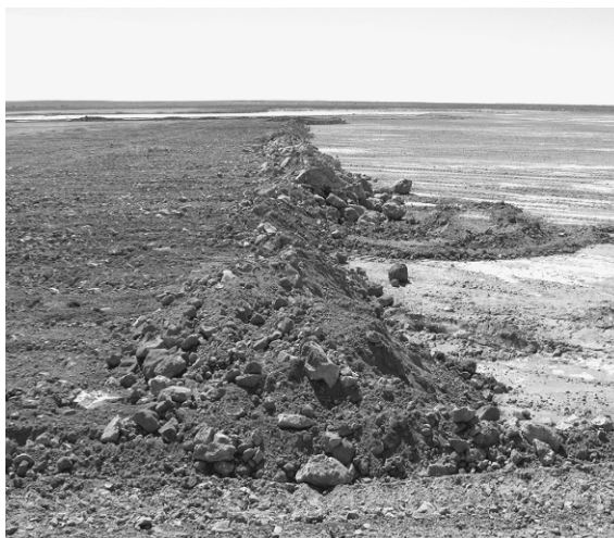
FIGURE 7.3. The entire top of a TSF is being covered with earth and waste rock. Photograph courtesy of Harley Lacy.
