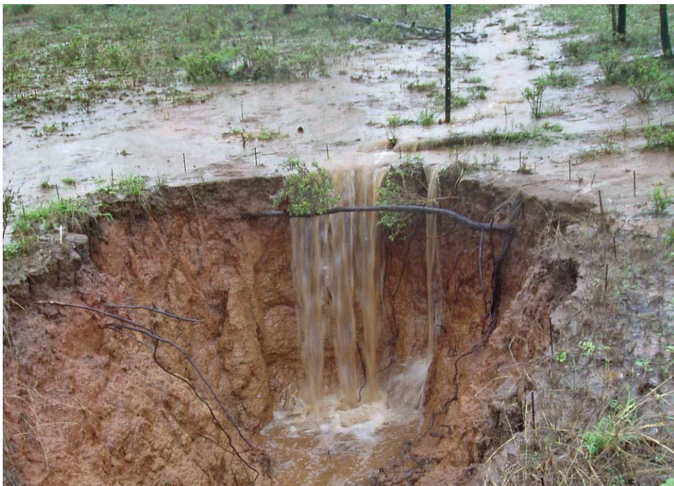
PLATE 2.2. Landscape where runoff is cutting a gully. Photograph courtesy of Aaron Hawdon.
