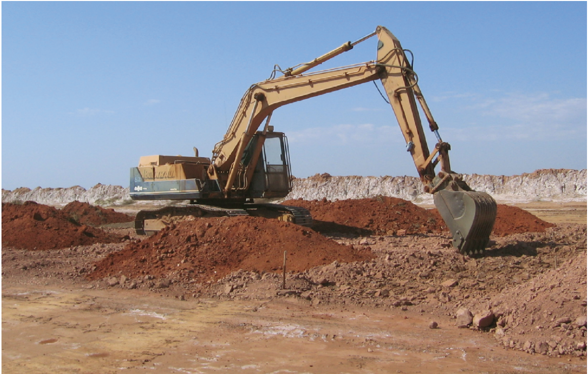
PLATE 7.1. The top of a tailings storage facility being covered with topsoil after capping with coarser materials. Photograph courtesy of Harley Lacy.
