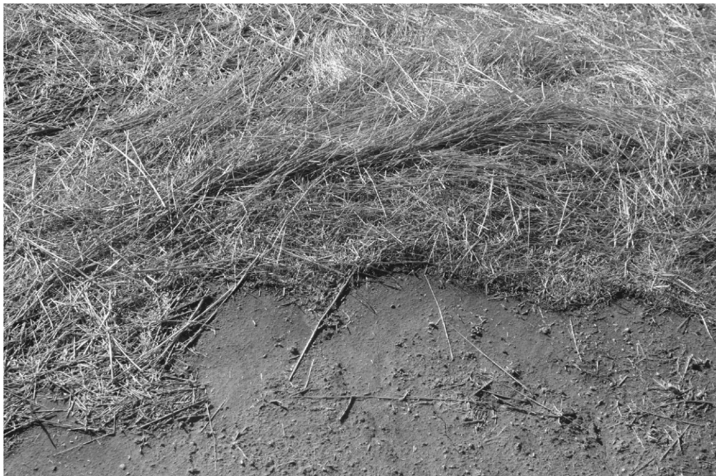
FIGURE 6.9. An example of the application of hay mulch to trap sediments on an eroding slope (see figure 6.8). All sediments were being trapped in the upper 40 cm of the applied mulch.
