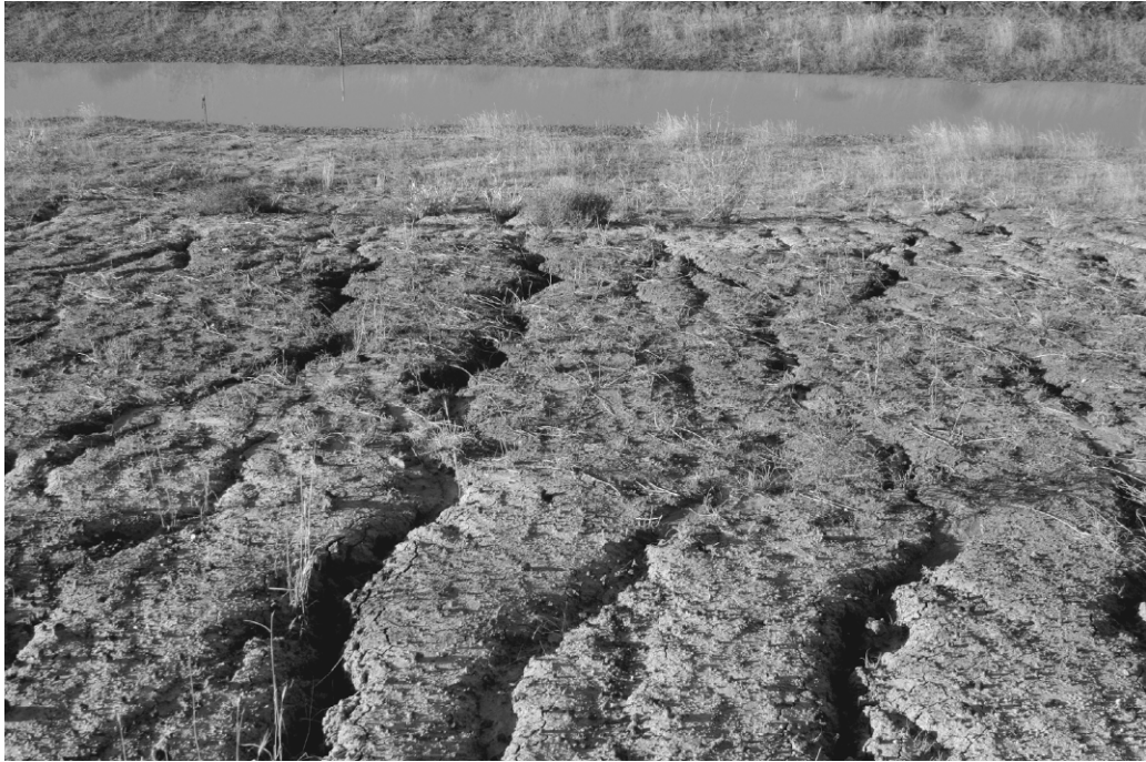
FIGURE 6.8. An example of a slope that has eroded into rills, with water ponding at the base of the slope rather than infiltrating into the slope to benefit plants.
