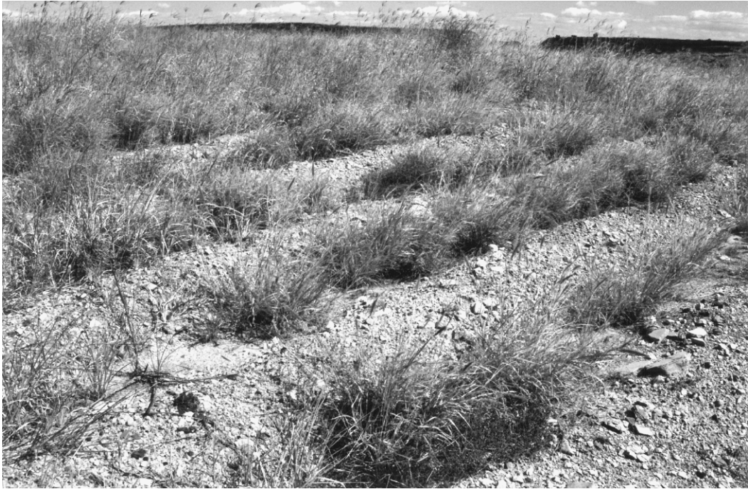
FIGURE 7.4. An example of vegetation established on a gently sloping TSF wall covered with earth and waste rock in a semiarid environment.
