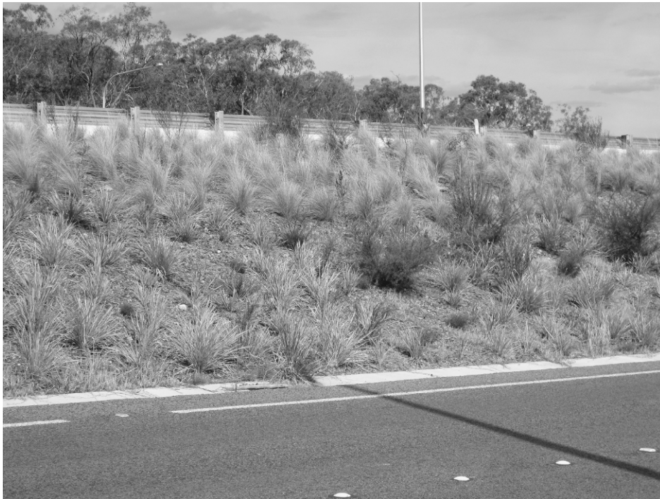
FIGURE 12.1. A road verge where native grasses, mat rushes, and shrubs have successfully established and are providing an attractive and protective roadside covering. After rainfall events, no sediments accumulate at the foot of this embankment.
