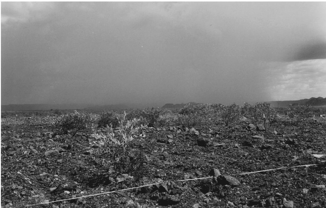
FIGURE 6.2. An example of a waste-rock dump that has been shaped into a plateau-like landscape and covered with coarse regolith materials. Note the approaching rainstorm.
