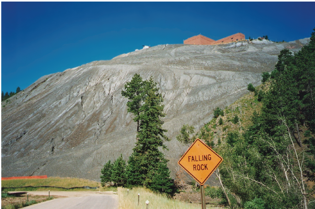
PLATE 3.1. Forest landscape has been buried by waste materials (spoil) created by mining. Gullies are cutting into the steep slopes, but this has not deterred someone from building a house on top of this mine-spoil heap.
