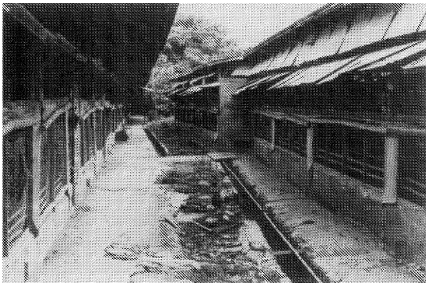
Fig. 2. A typical New Territories chicken farm. Note the proximity of the buildings, also the fold-down shutters and roll-down blinds to adjust ventilation.
