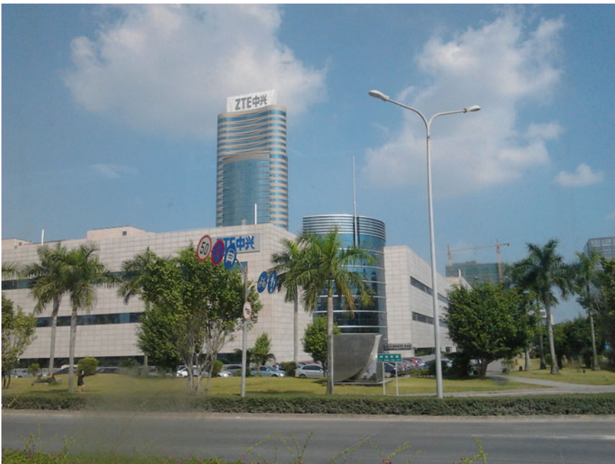
Fig. 3.7 ZTE Corporation, a leading Chinese multinational telecommunications equipment and systems company in Shenzhen (taken by the authors in December 2012)
