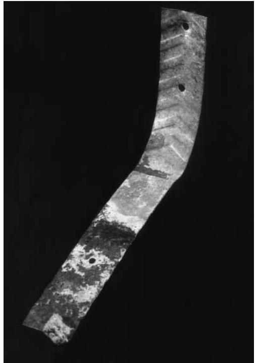
FIGURE 33.2 Corroded timber frame masonry wall tie showing both white rust ( ZnO ) and red rust ( Fe_2O_3 \cdot H_2O ).
