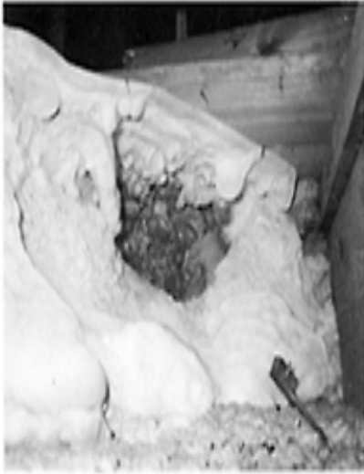
Serpula lacrymans (dry rot) fruiting body and mycelium filling a void.
