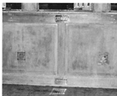
Ventilation of the wall void (via wood panelling).
