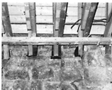
Joist ends isolated from masonry on a DPC membrane.
