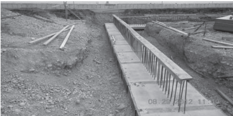
Covers—high in labor, handling and fabrication hazards, then, protection removed during worker activity
