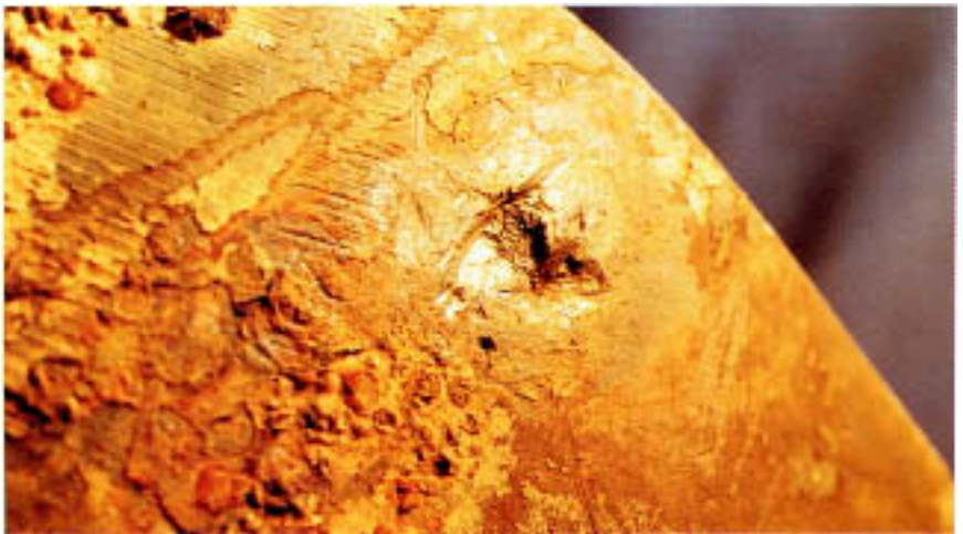
Figure 17.12 Corroded area beneath a tubercle on the external surface. The shiny black corrosion product has been partially removed to reveal the depth of penetration.
