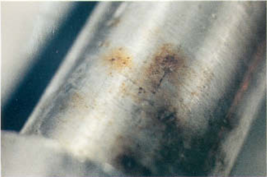
Figure 4.13 Rust patches surround small pits on a stainless steel shaft. The rust is formed by oxidation of ejected ferrous ion from the tiny pits. Pits were initiated by chloride and sulfate ions concentrated by evaporation.
