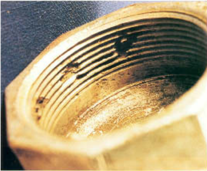
Figure 2.17 Pitting at a free-machining austenitic stainless steel threaded valve throat. The valve controlled flow of a chlorine-containing, low-pH biocide.
