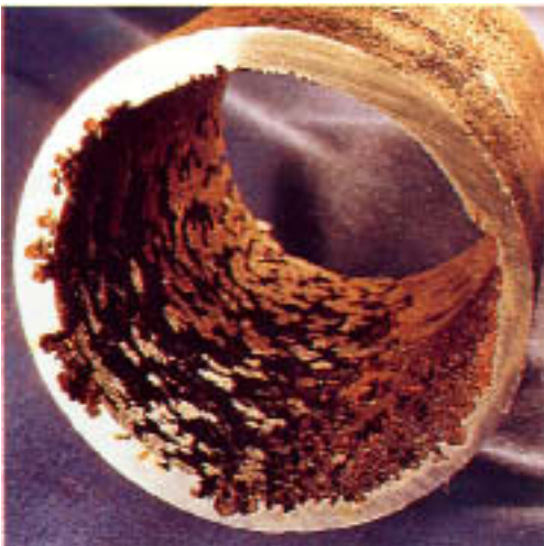
Figure 7.2 Carbon steel pipe attacked by a strong mineral acid.
