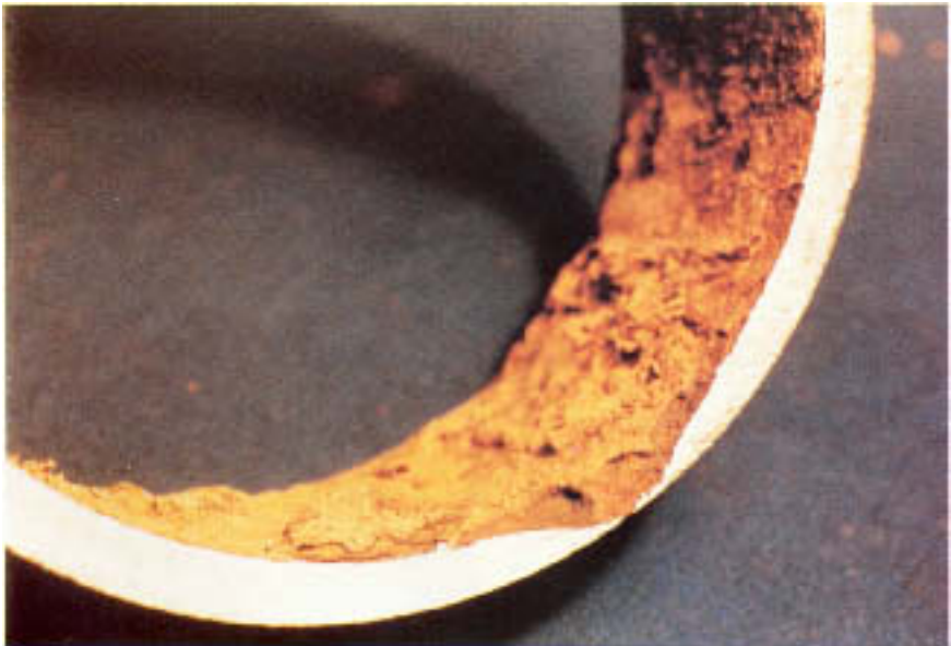
Figure 3.23 Perforation at a dish-shaped depression on the internal surface of a large-diameter steel pipe. A large tubercle capped the depression but was dislodged during tube sectioning. (Courtesy of National Association of Corrosion Engineers, Corrosion '89 Paper No. 197 by H. M. Herro.)
