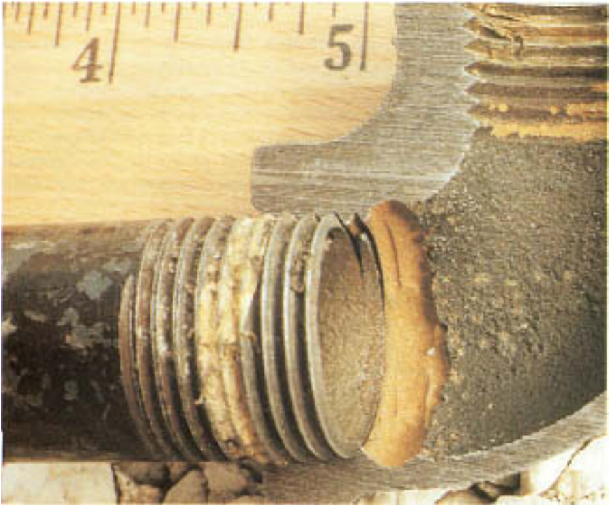
Figure 7.17 Locally wasted region at an inlet pipe. See Fig. 7.18. Note the severe attack at the discharge end of the straight pipe.
