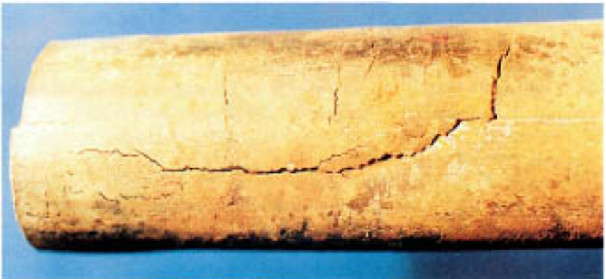
Figure 9.4 Both longitudinal and transverse stress-corrosion cracks on a brass heat exchanger tube that had been exposed to ammonia. Note the branching of the cracks.
