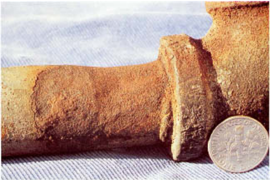
Figure 5.12 Severely corroded galvanized steel pipe supplying water to a cooling tower fan-bearing system. Where the galvanized metal has been consumed, only a brown rust patch is visible.
