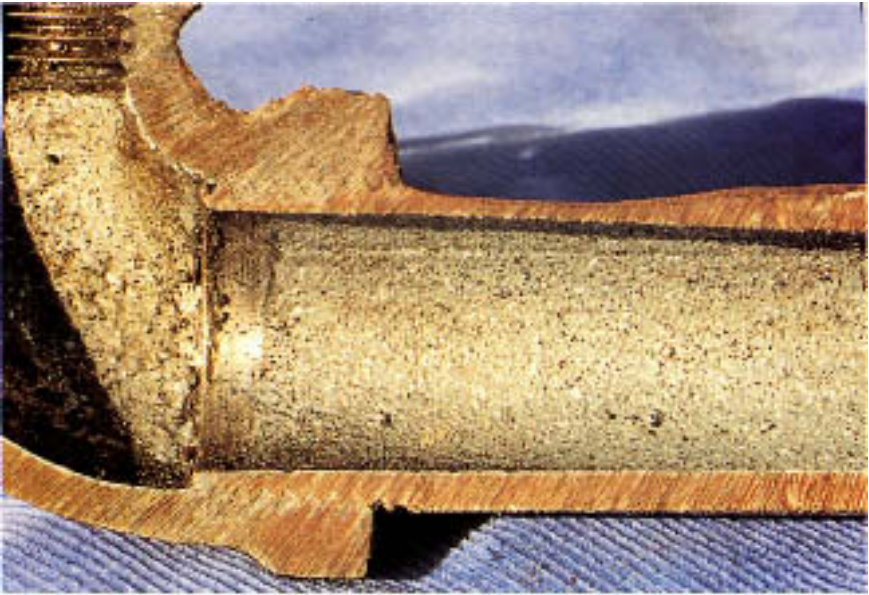
Figure 5.13 As in Fig. 5.12 but with pipe in cross section, showing severe wastage where the galvanized layer is absent.
