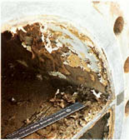
Figure 6.13 A dried slime layer peeling off water box surfaces on a small heat exchanger.
