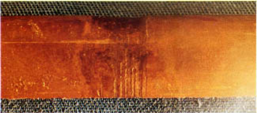
Figure 2.10 Wastage in a circumferential region where a 90:10 cupronickel main condenser tube passed through a baffle. In places, metal loss was greater than 25% of the nominal wall thickness.
