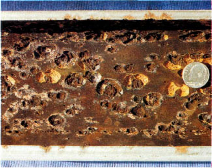
Figure 5.8 Heavily pitted surface of a mild steel cooling water return line. Note the deep localized metal loss surrounded by aureoles of rust. Pitting is common when oxygen concentration varies greatly over time.
