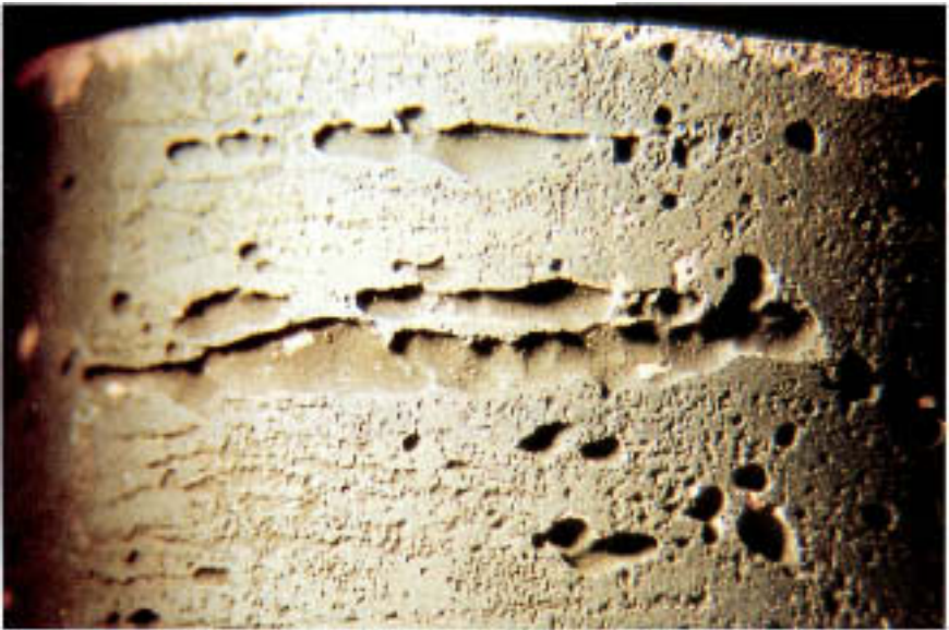
Figure 7.24 Deep groove in region of localized metal loss on a copper tube. Grooving was caused by carbonic acid containing high concentrations of dissolved oxygen.
