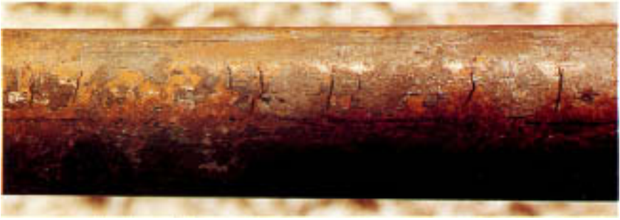
Figure 10.2 A family of short, transverse corrosion-fatigue cracks originating on the external surface.
