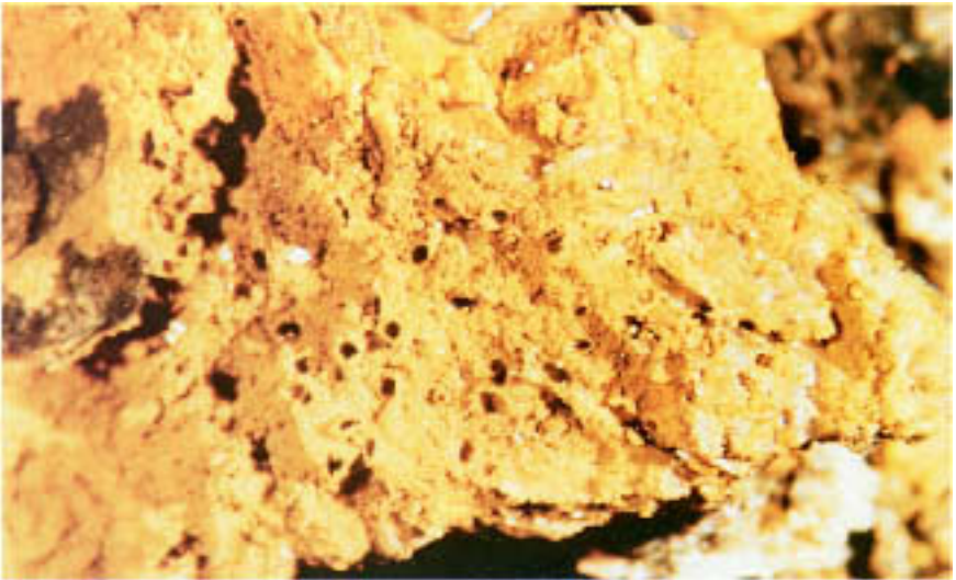
Figure 6.17A A corrosion-product and deposit mound on a mild steel service water pipe honeycombed by small tubelike organisms. Each hole is approximately 0.01 in. (0.025 cm) in diameter.
