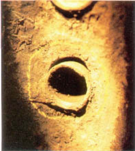
Figure 2.9 Severely attacked crevice between rolled brass heat exchanger tube and mild steel tube sheet.
