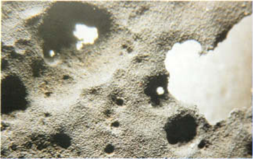
Figure 7.20 Close-up of general wastage on a carbon steel bracket subjected to low-pH (<2) mill coolant.
