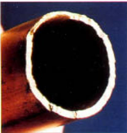
Figure 10.3 Blunt fracture edges typical of corrosion-fatigue cracks.
