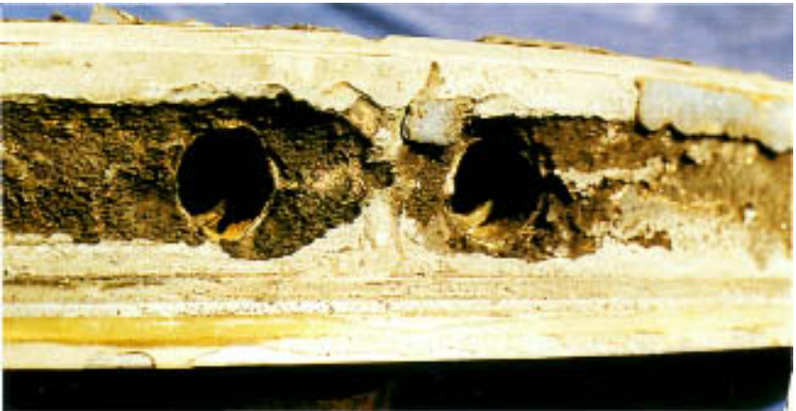
Figure 16.5 Severe deterioration adjacent to nozzle holes where brass nozzles had been inserted.
