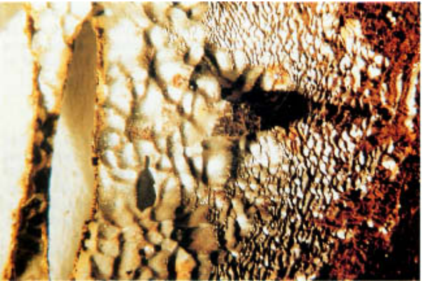
Figure 11.3 Sand dunelike erosion-corrosion patterns on the inlet end of a steel heat exchanger tube. (Magnification: 7 \times .)
