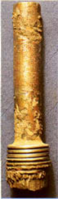
Figure 6.22 A thermocouple housing showing localized wastage. Small fibers containing high concentrations of salt were found in corroded areas.
