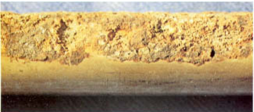
Figure 4.12 As in Fig. 4.11. Note how abruptly corrosion terminates at deposit edge.
