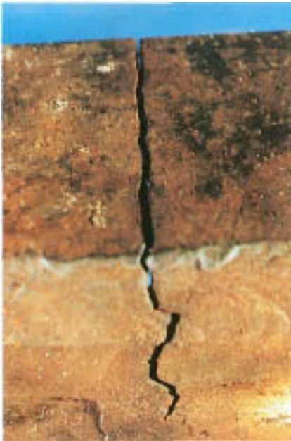
Figure 15.25 Appearance of fracture along the external surface.
