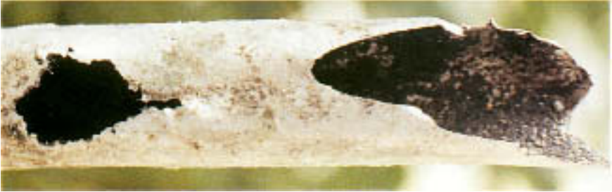
Figure 7.21 Austenitic stainless steel pipe that carried sulfuric acid. Failure was caused by severe general wastage from internal surfaces.
