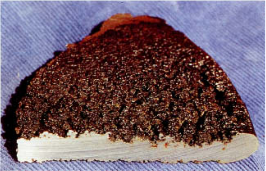
Figure 17.15 Section of a cast iron pump impeller that has suffered graphitic corrosion followed by cavitation damage.
