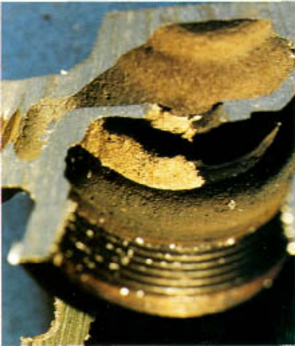
Figure 11.29 Erosion-corrosion of a valve seat (bright metal in center of photograph).
