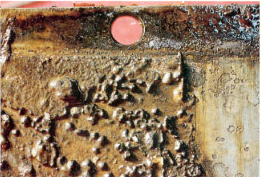
Figure 4.27B As in Fig. 4.27A but with deposits removed to show corrosion beneath.
