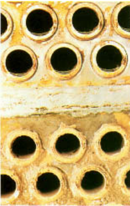
Figure 6.12B As in Fig. 6.12A, but split above and below the water box to show the clean outlet sheet (top) and the slimed inlet sheet (bottom).
