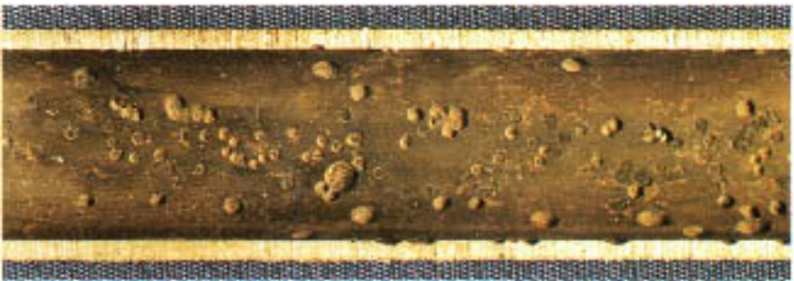
Figure 6.3 Pitting on the waterside surface of a Carpenter 20 heat exchanger tube caused by sulfate reducers.
