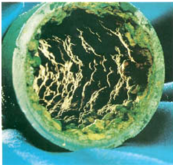
Figure 3.12 Heavily tuberculated 3-in. (7.6-cm) outer diameter steel mill water supply line.
