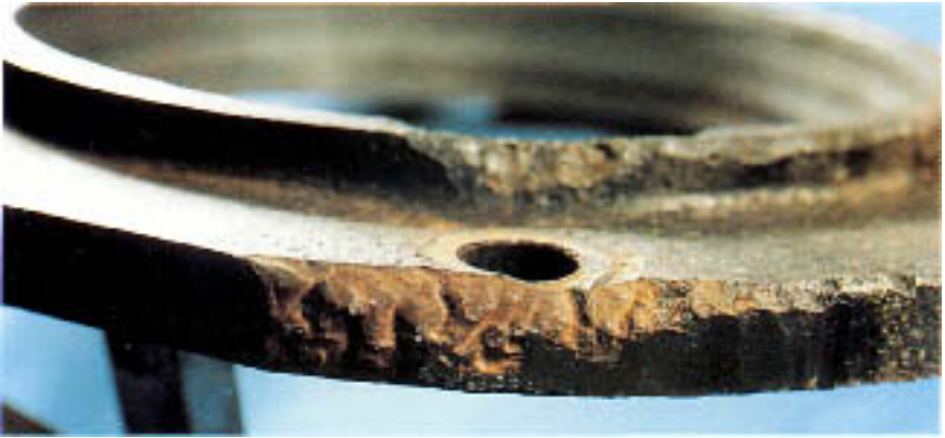
Figure 11.31 Severe metal loss on the retainer plate at a bolt hole (see Fig. 11.32).
