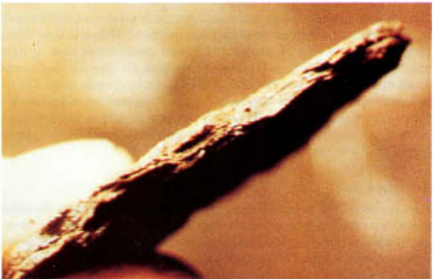
Figure 5.7 Rust chip as in Fig. 5.6.
