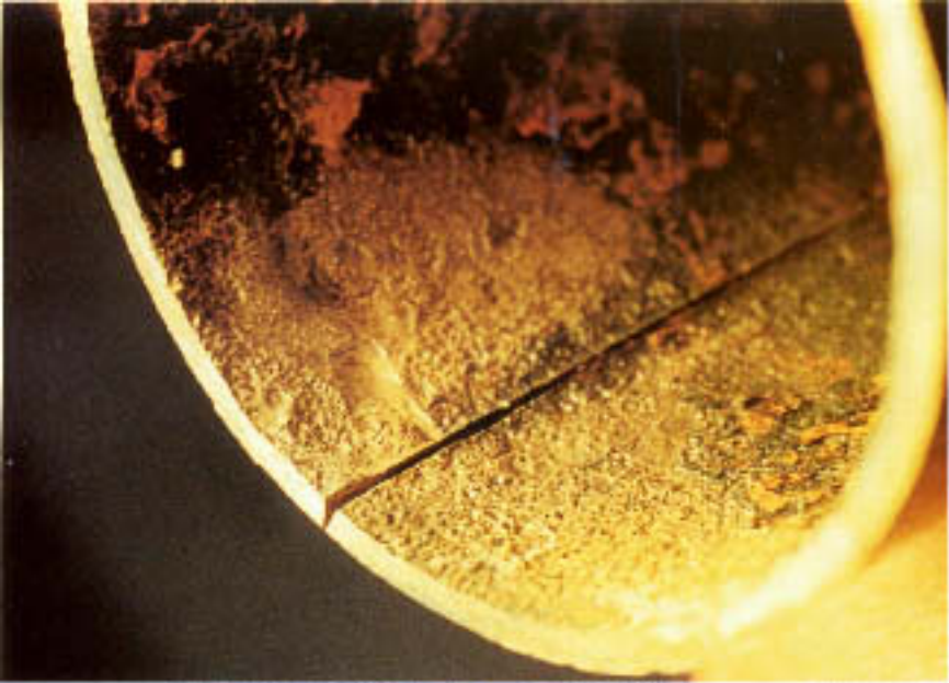
Figure 14.5 Severe seam defect apparent after acid cleaning of the internal surface.
