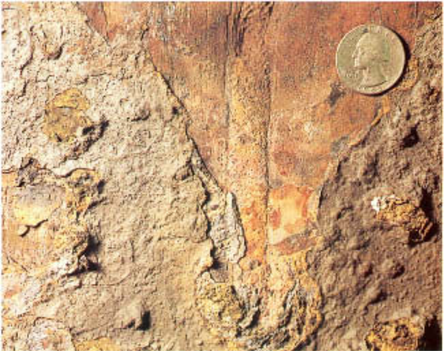
Figure 3.26 Typical internal surface of heavily tuberculated mill water supply line about 16 hours after removal from system. Surface resembled Figs. 3.19 and 3.20 immediately after removal. Note the weld where corrosion product and deposit were removed.
