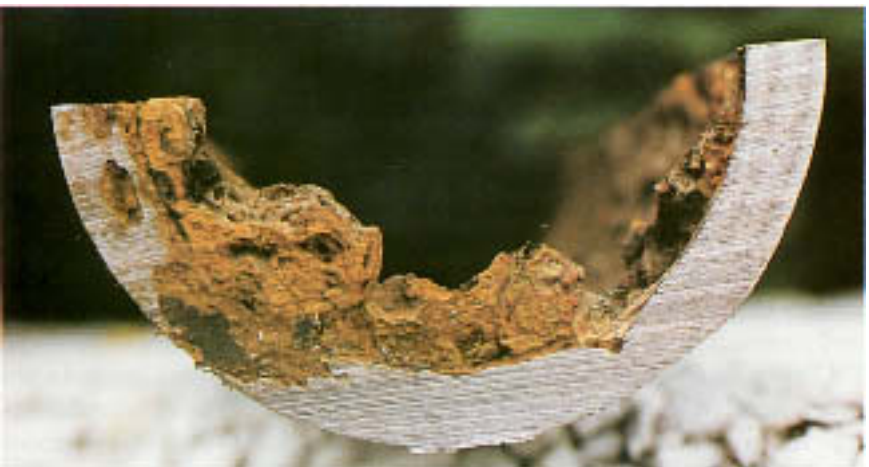
Figure 6.10 A perforated carbon steel pipe at a weld-backing ring. The gaping pit was caused by sulfate-reducing bacteria (see Case History 6.1).
