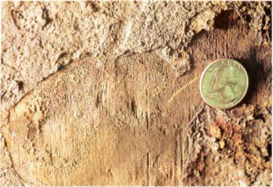
Figure 3.24 Striated, corroded depressions are revealed on a large-diameter pipe after tubercles were removed. Striated surfaces are caused by preferential corrosion along microstructural irregularities in the steel. Such attack can be caused by low pH conditions.
