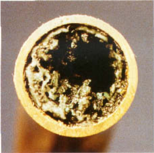
Figure 4.30A Brass cooler tube almost plugged by deposits.
