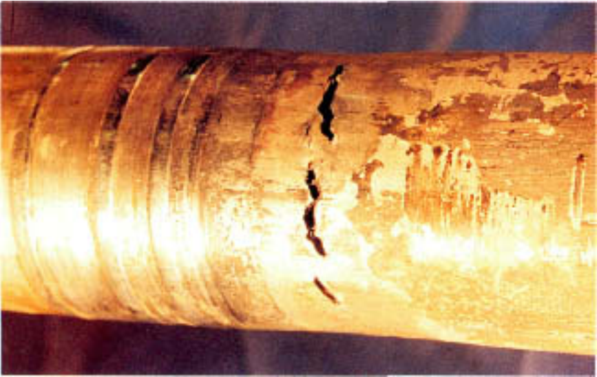
Figure 9.19 Circumferential cracks along one side of the heat exchanger tube. Note proximity of cracks to the plane of the tube sheet, as indicated by the tube sheet grooves (left). Expansion of the cracks may have occurred during removal of the tube from the exchanger.
