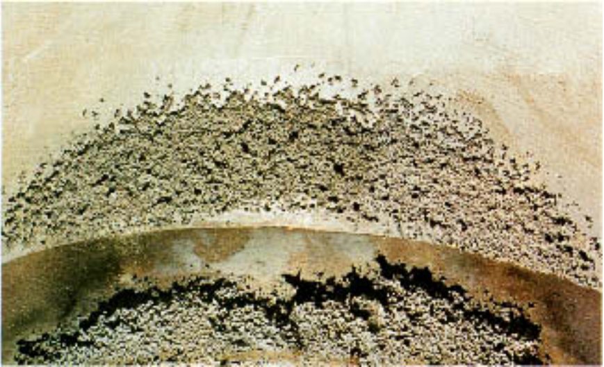
Figure 12.17 Metal loss downstream of flange wall expansion.
