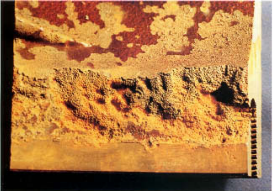
Figure 17.13 Severe metal loss along an internal surface.
