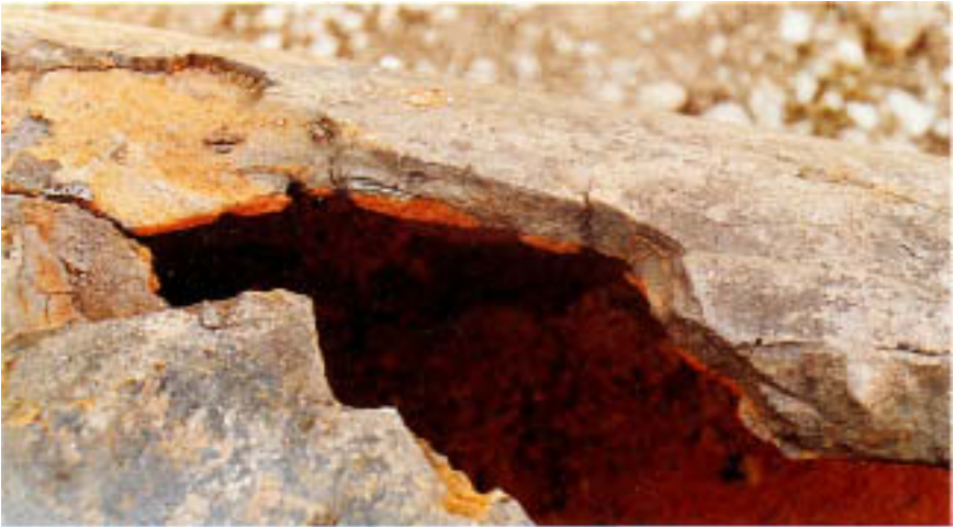
Figure 17.5 Brittle fracture through pipe. The gray material is graphitically corroded cast iron. Unaffected pipe wall metal is orange from normal rust.
