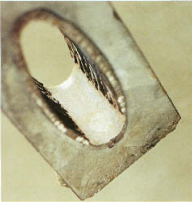
Figure 7.15 General thinning along the bottom of a steel conduit carrying carbonic acid-laden water.
