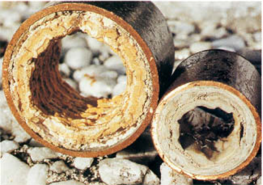
Figure 4.16 Thick calcium carbonate deposits on condenser tube and copper transfer pipe. Note the stratification.
