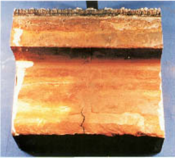
Figure 15.24 Section of cracked door frame.
