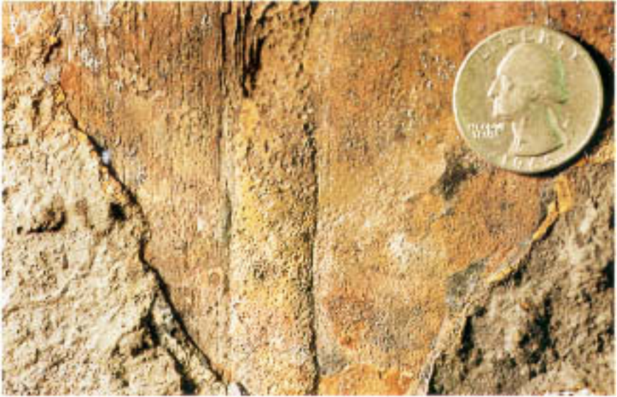
Figure 3.27 As in Fig. 3.26, showing preferential weld attack.
