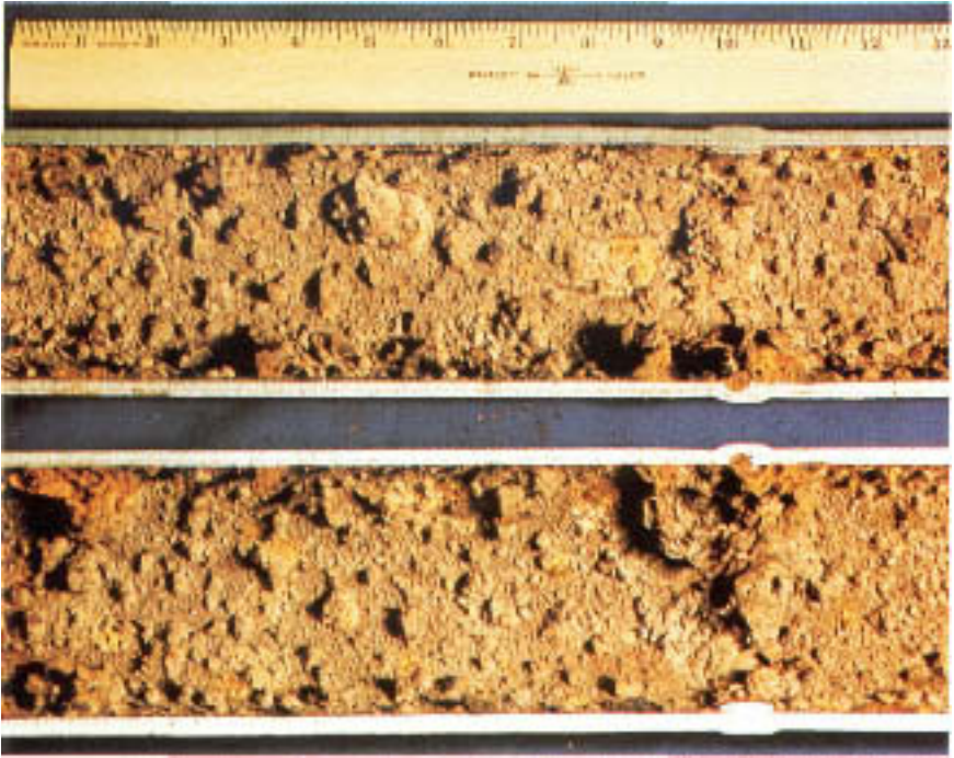
Figure 3.13 Emergency supply line shows moderate tuberculation.
