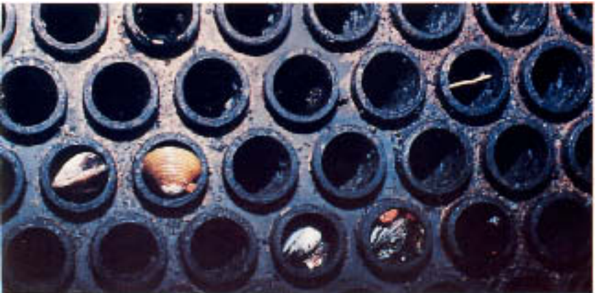
Figure 6.16 Small clams lodged in heat exchanger tube inlet ends. (Courtesy of Rick Ruckstuhl, Nalco Chemical Company.)
