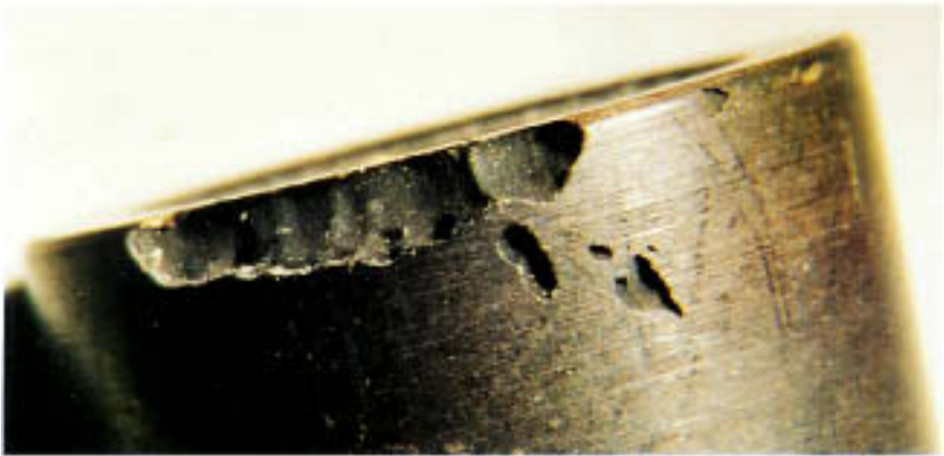
Figure 11.30 Metal loss by erosion-corrosion at edges of a throttling nut. (Magnification: 7 \times .)
