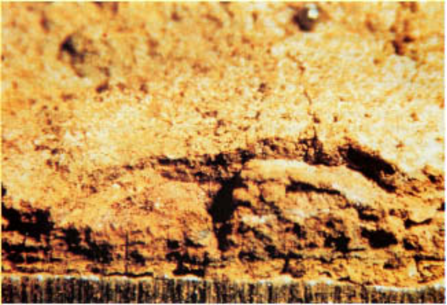
Figure 5.14 Stratified corrosion products and deposits on the internal surface of a tube. (Magnification: 7.5 \times .)
