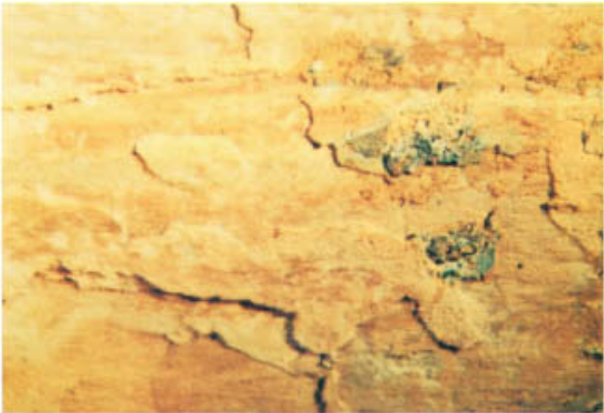
Figure 4.14 Silt layer on the internal surface of a 90:10 cupronickel condenser tube.
