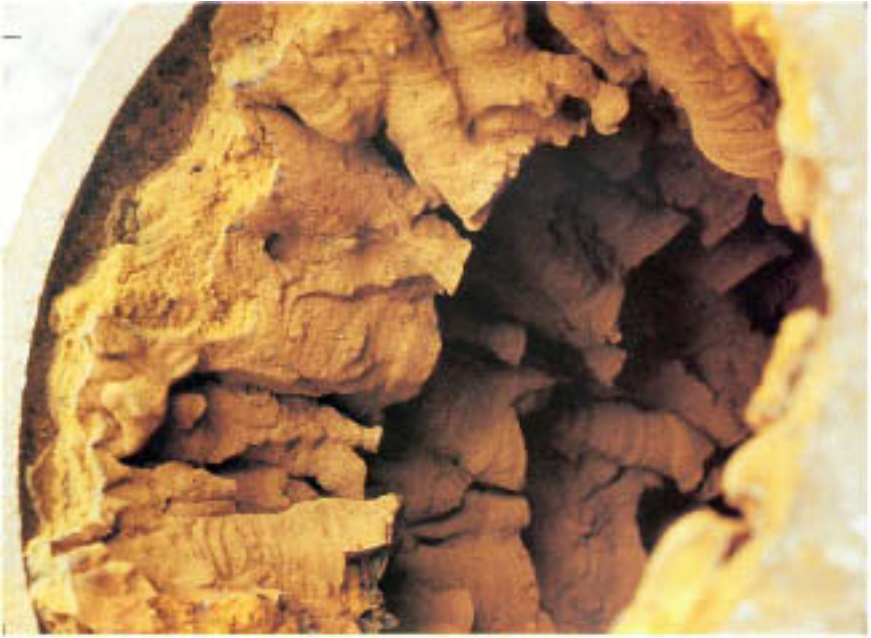
Figure 3.11 Tubercles elongated by flow in a mill water supply line.
