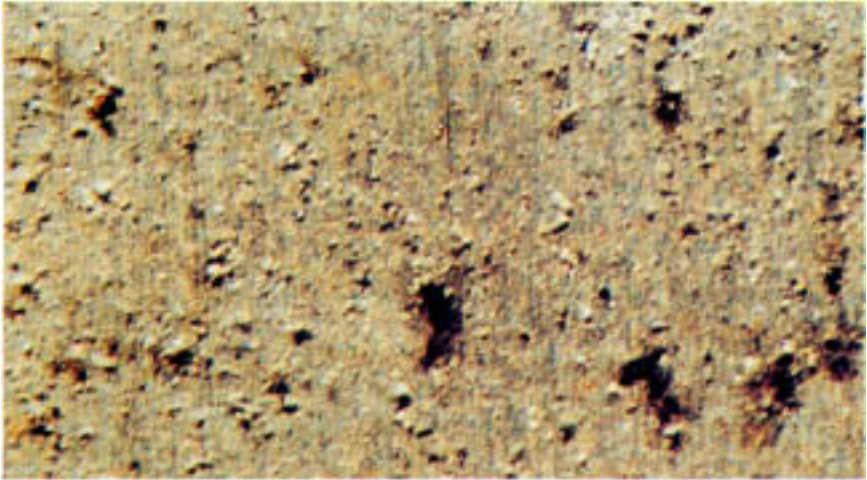
Figure 7.22 Pitting on a 304 stainless steel coupon caused by acidic, chloride-containing water condensating and evaporating. High chloride concentrations were produced locally.
