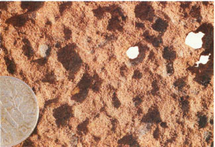
Figure 5.10 Generally corroded steel surface.
