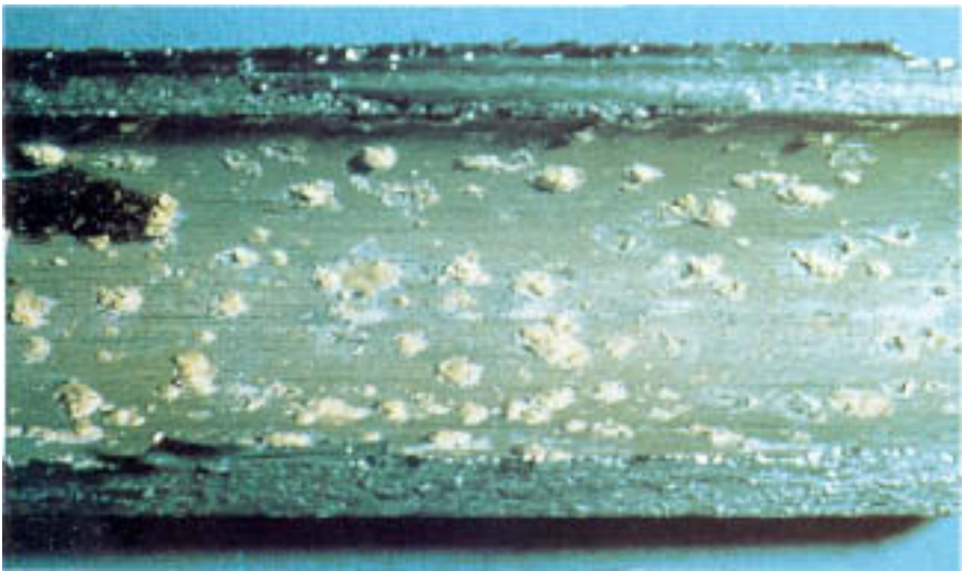
Figure 4.4 Corrosion product mounds covering localized areas of metal loss on an aluminum heat exchanger tube. Attack initiated beneath a thin deposit layer.
