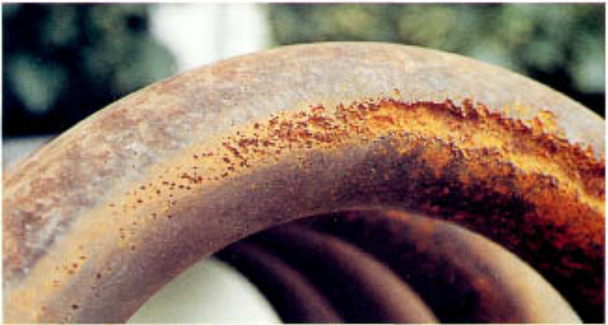
Figure 7.14 As in Fig. 7.13. Note the presence of orange iron oxides and carbonate. Also note how attack starts as small pits due to dropwise condensation.
