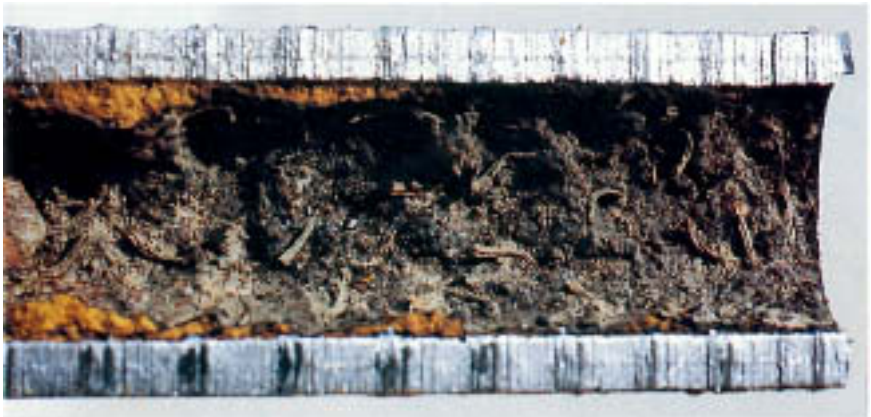
Figure 6.20A A 1 in. (2.5 cm) diameter mild steel service water pipe containing many small cone-shaped organisms.
