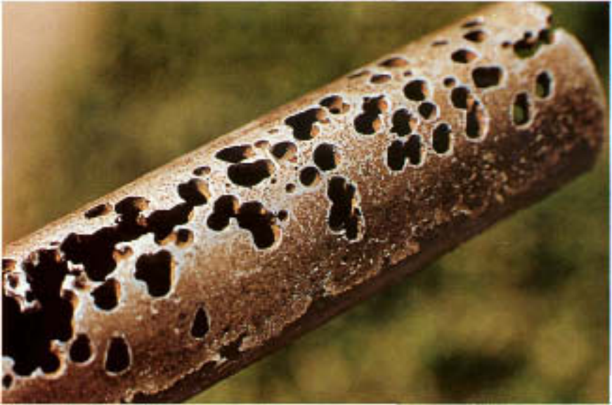
Figure 6.2 Severely pitted aluminum heat exchanger tube. Pits were caused by sulfate-reducing bacteria beneath a slime layer. The edge of the slime layer is just visible as a ragged border between the light-colored aluminum and the darker, uncoated metal below.
