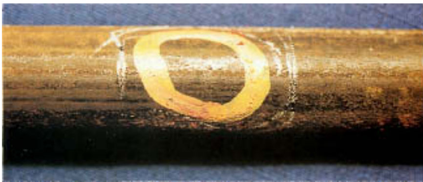
Figure 14.1 Pinhole perforation in a steel heat exchanger tube, viewed from the external surface.
