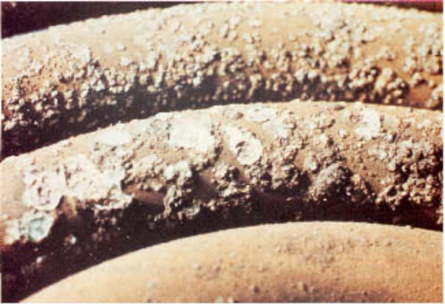
Figure 4.17 Corroded copper tubes from a heating coil. Cooling water contacted the visible surface. The mounds consist of copper carbonate (see Fig. 4.18).
