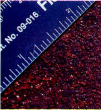
Figure 6.14 A generally corroded carbon steel surface after the slime layer was removed.
