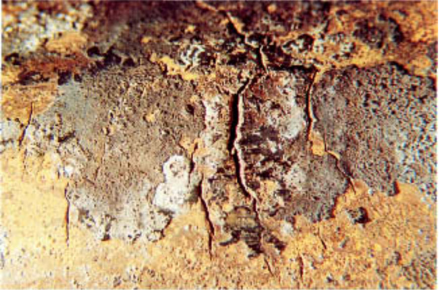
Figure 10.9 Close-up of cracks. (Magnification: 7.5×.)
