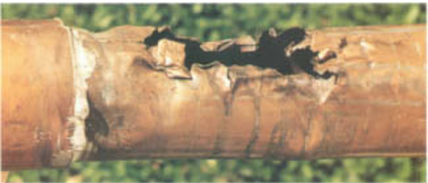
Figure 8.10 A large, ragged perforation in a region of severe internal wastage on a copper pipe. Corrosion was caused by ammonia-containing condensate.
