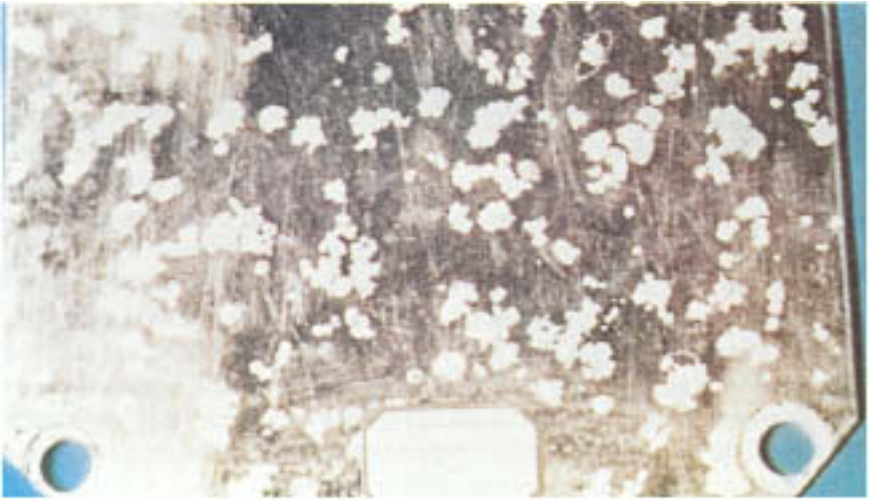
Figure 4.3 A 304 stainless steel plate from a storage tank floor, which pitted beneath a deposit layer.
