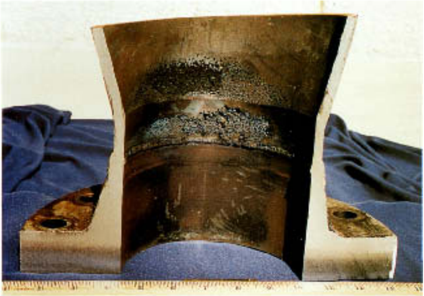
Figure 12.15 Damage to the internal surface of a supply line.
