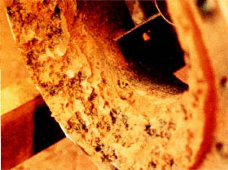
Figure 17.10 Appearance of the graphitically corroded throat of a pump housing.
