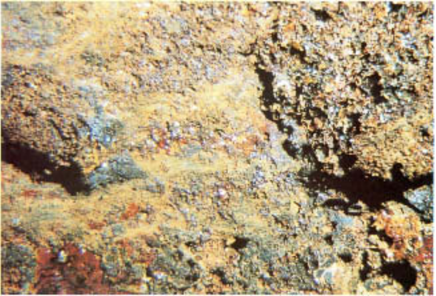
Figure 4.21 Internal surface (waterside) of alloy steel heat exchanger. Corrosion products and deposits partially cover pits. (Magnification: 7.5 \times .)
