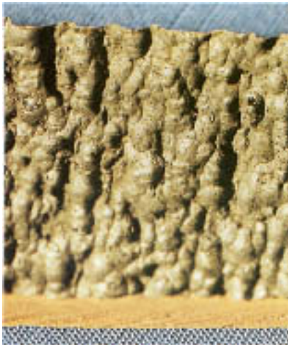
Figure 7.16 Carbon steel corroded by organic acid on a cast iron pipe elbow.
