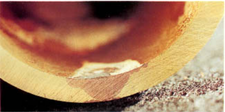
Figure 13.4 A large plug of dezincified metal beneath a deposit. Plugs often form on the bottom of horizontal pipes, beneath deposits.
