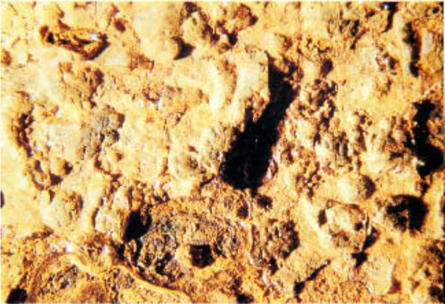
Figure 5.16 Delaminated, phenolic epoxy resin coating on an internal surface. (Magnification: 7.5 \times .)
