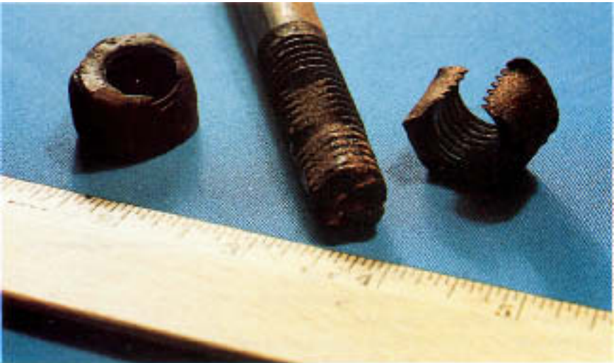
Figure 11.32 Severe localized metal loss on bolt threads and on nuts.
