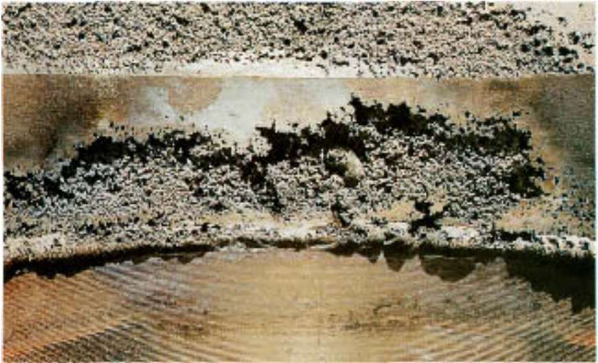
Figure 12.16 Jagged metal loss downstream of protruding weld bead.
