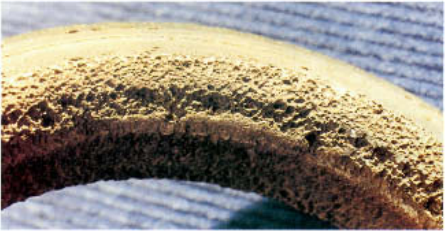
Figure 8.5 As in Fig. 8.4 but at greater enlargement. Note the intersection of pitlike depressions to form more general metal loss.
