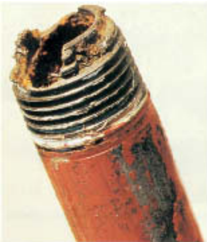
Figure 2.18 Wasted threads on small-diameter mild steel pipe.
