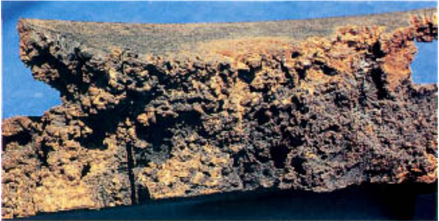
Figure 12.14 Typical appearance of severe cavitation damage in cast iron.
