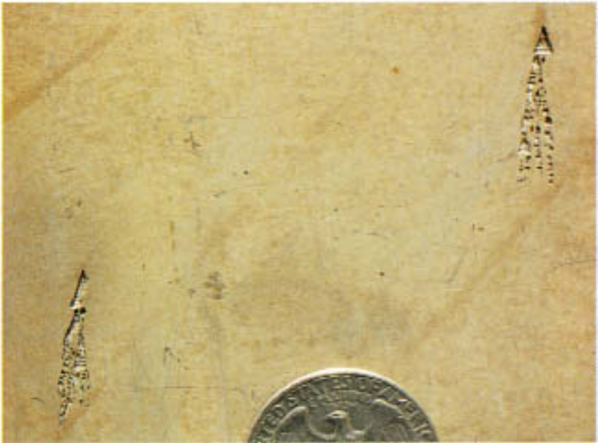
Figure 7.5 Pits on a large-diameter austenitic stainless steel pipe. Note the grooves formed by leakage of pit contents down the pipe wall in the direction of gravity. (Pipe wall was vertical in service.)
