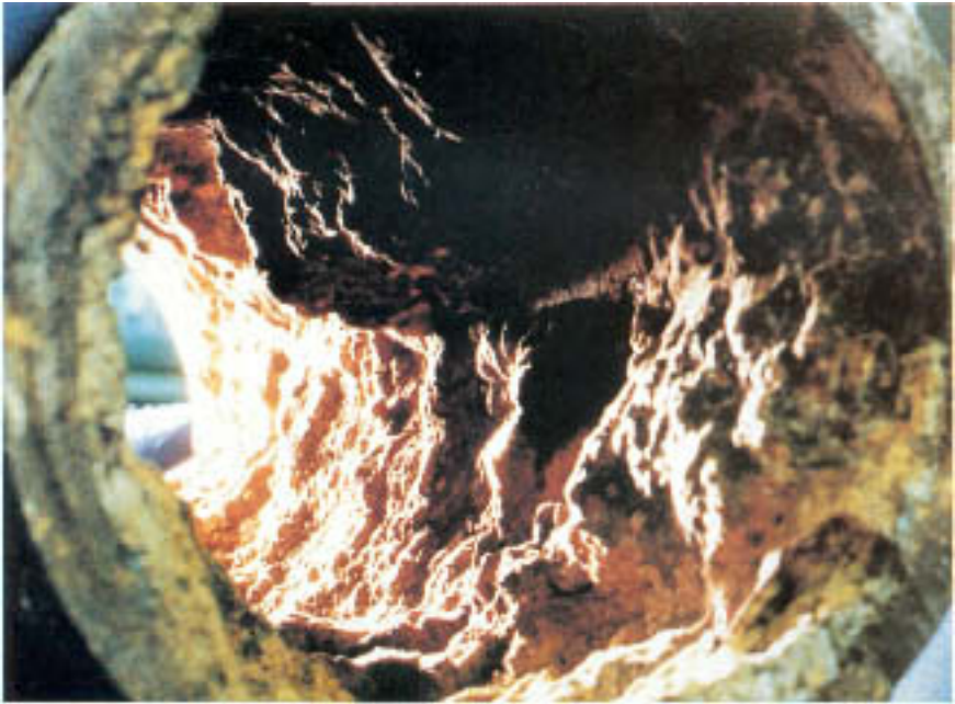
Figure 3.1 Utility service water system pipe almost plugged by heavy tuberculation.
