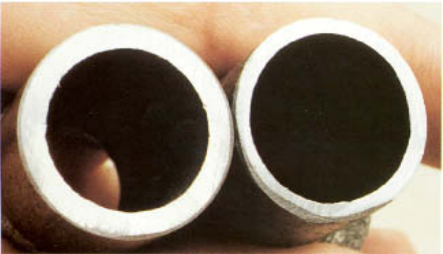
Figure 7.18 Generally wasted pipe (to the viewer's right) and new pipe. Wastage was general near a pump discharge due to high flow.
