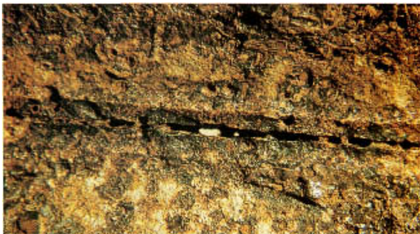
Figure 14.3 Close-up of the internal surface following acid cleaning. Note the perforation in the tube wall along the weld seam.
