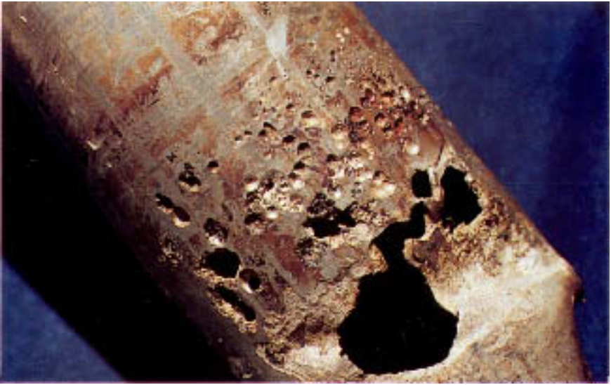
Figure 6.5 Many small hemispherical pits on a 304 stainless steel heat exchanger tube end. The heat exchanger was removed from service and stored vertically for an extended period. Deposit accumulated at the lower tube ends where sulfate reducers flourished.
