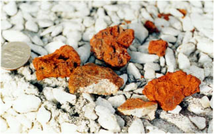
Figure 11.24 Concrete chips covered with orange iron oxide that were removed from the tube ends.
