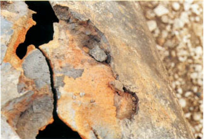
Figure 17.8 The black outer covering is corrosion product; the reddish-brown surface is coated with air-formed iron oxide.
