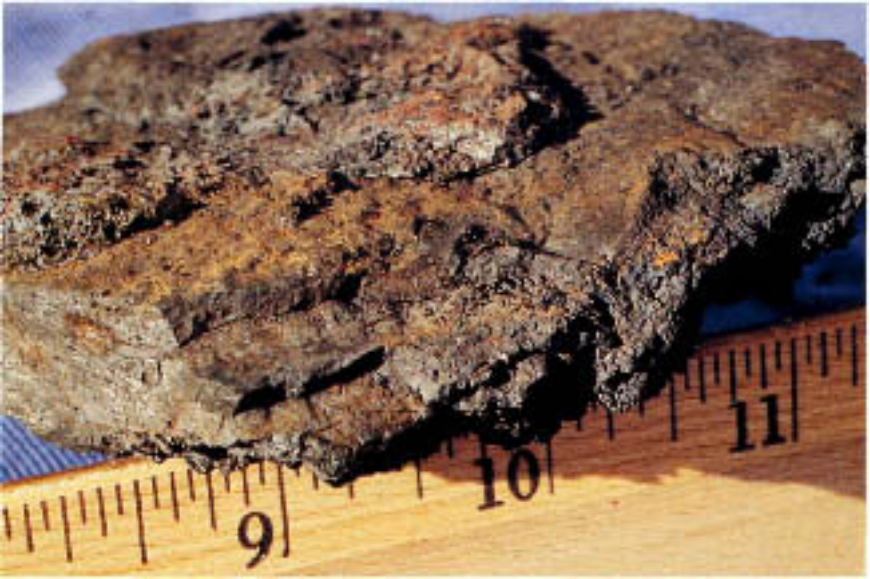
Figure 5.9 Wall of steel tank, originally \frac{1}{2} in. (1.3 cm) thick, that was entirely converted to oxide. It was continually exposed to oxygenated water mist at about 180^{\circ}\text{F} ( 82^{\circ}\text{C} ).
