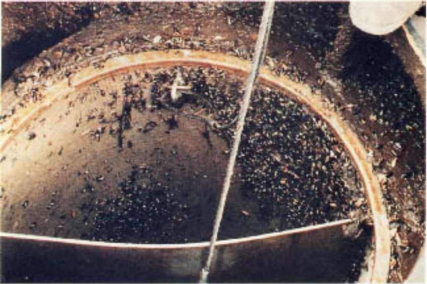
Figure 6.15 A main mill water-strainer basket caked with clams.
