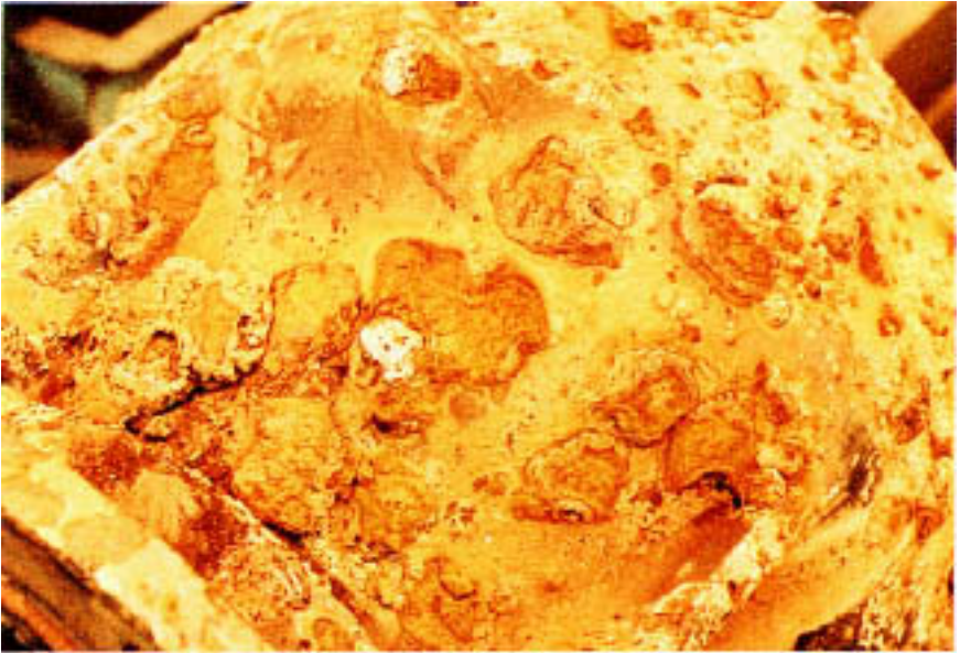
Figure 17.11 External surface of a pump housing showing tubercles capping sites of graphitic corrosion.
