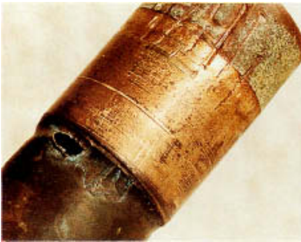
Figure 8.6 Severe grooving by ammonia-containing condensate on an admiralty brass condenser tube. Condensate flowed down the tube sheet and collected at the tube end, cutting an annular groove. Note the perforation just outside the tube roll.
