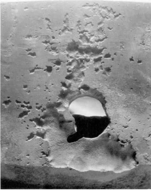
Figure 17.18 Close-up of the perforation in Fig. 17.16 viewed from the external surface. Graphitic corrosion of the external surface permitted erosion by turbulent water escaping through the perforation.
