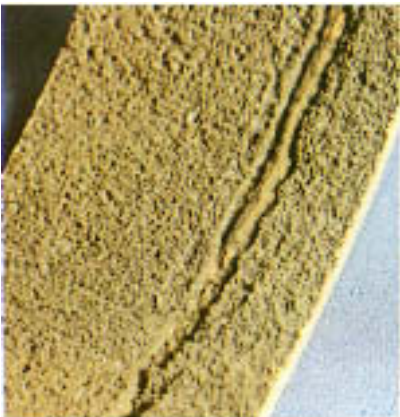
Figure 7.10 Severely attacked weld on a large-diameter steel pipe by an acid upset.
