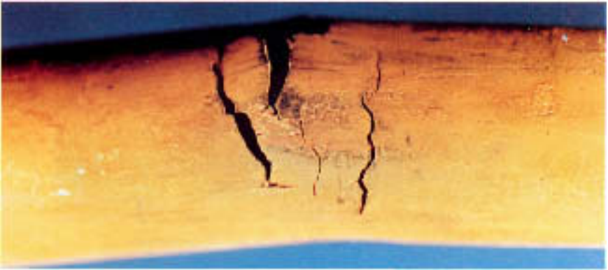
Figure 9.3 Transverse stress-corrosion cracks in a condenser tube; the presence of the cracks along just one side indicates that a bending moment provided the stress.
