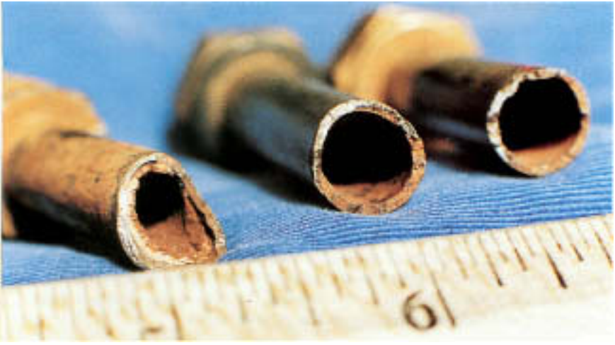
Figure 9.18 Cracked connectors; note brittle, thick-walled character of the cracked faces and the accumulation of alkaline deposits on the internal surface of the connector on the left.
