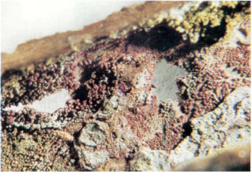
Figure 4.29 Corroded internal surface of a copper chiller tube. The light-colored deposits are primarily iron oxides and silicates; reddish material is cuprous oxide.
