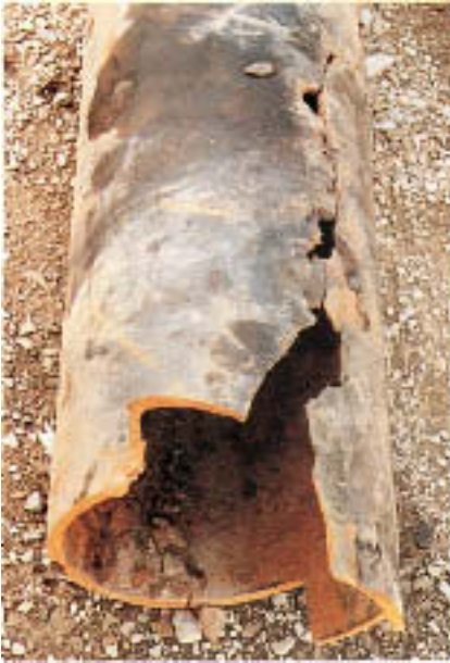
Figure 17.7 Section of longitudinally fractured subterranean cooling water line. Note that the crack runs the entire length of the line.
