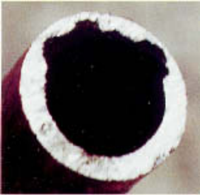
Figure 6.7 A small-diameter carbon steel service water pipe perforated by sulfate-reducer corrosion.
