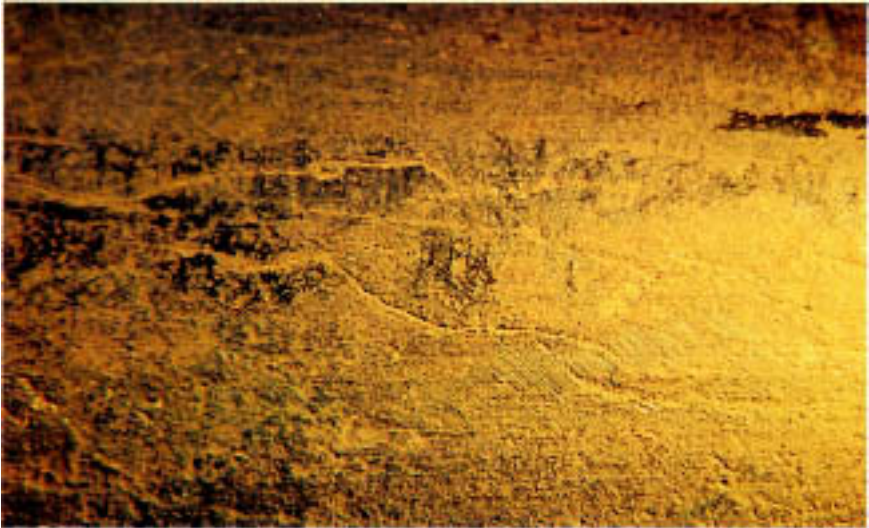
Figure 9.11 A network of longitudinal cracks along the external surface. (Magnification: 7.5 \times .)
