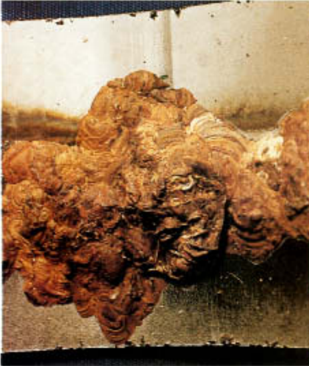
Figure 6.9A Irregular deposit and corrosion-product mounds containing concentrations of sulfate-reducing bacteria on the internal surface of a 316 stainless steel transfer line carrying a starch-clay mixture used to coat paper material. Attack only occurred along incompletely closed weld seams, with many perforations. Note the heat tint, partially obscured by the deposit mounds, along the circumferential weld.
