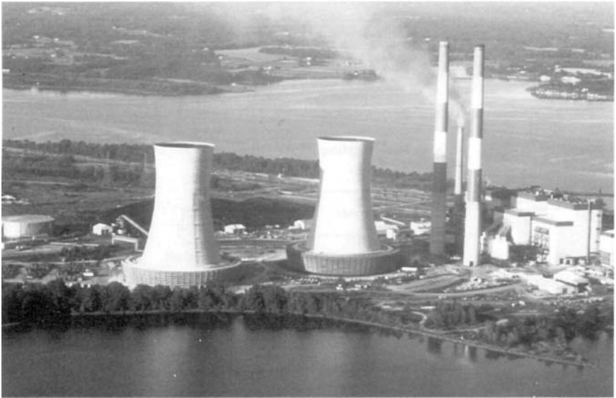
Figure 1.5 Hyperbolic towers cooling condenser water in a utility station. [Fig. 38.10, The Nalco Water Handbook, 1st ed. (1979) , reprinted with permission from McGraw-Hill, Inc., Courtesy of The Marley Company.]
