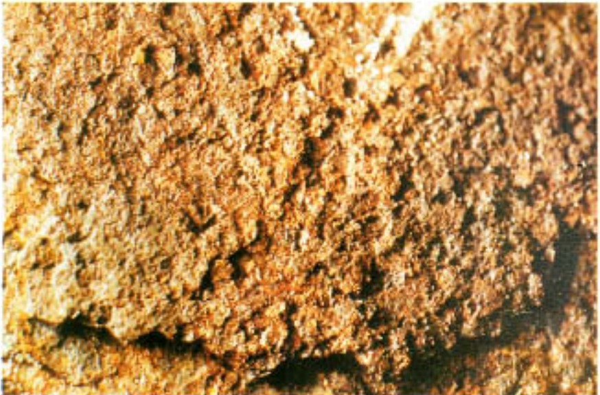
Figure 5.6 Rust layer on carbon steel mill water supply pipe. Note the partially exfoliated region at the bottom of the photo.
