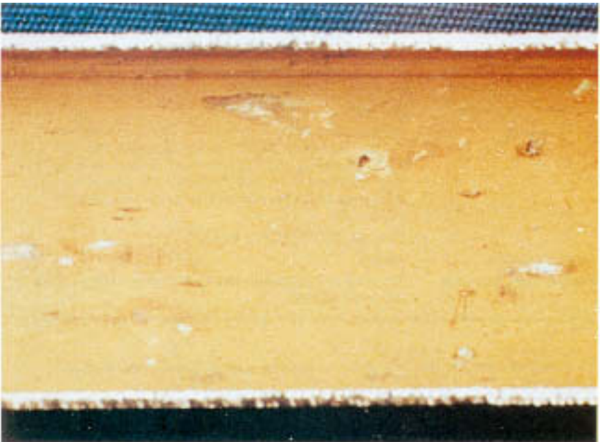
Figure 4.24 Internal surface of condenser tube as shown in Fig. 4.23.
