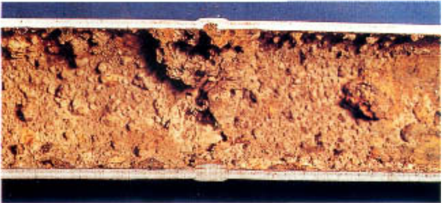
Figure 6.21 A longitudinally split carbon steel emergency service water pipe, as in Fig. 6.10. Note the circumferential weld-backing ring, which is consumed on one side.
