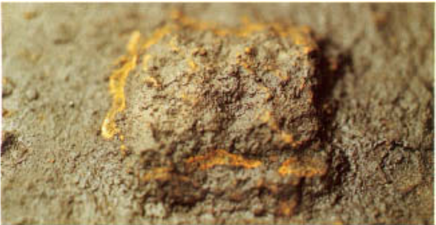
Figure 3.19 Tubercle only a few minutes after removal from a water-filled pipe.
