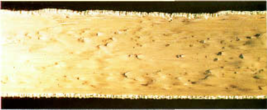
Figure 11.18 Erosion-corrosion in its mature form. Note the horseshoe-shaped depressions aligned with flow direction.
