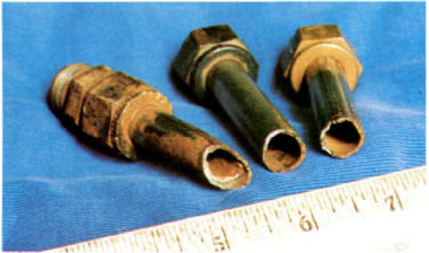
Figure 9.17 Stainless steel connectors showing circumferential fractures.
