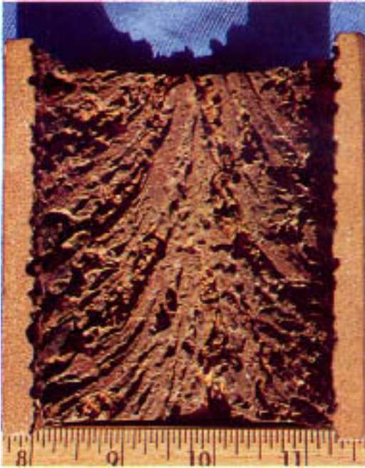
Figure 7.12 Jagged fir-tree pattern of metal loss caused by condensing steam with high concentrations of carbon dioxide and oxygen.
