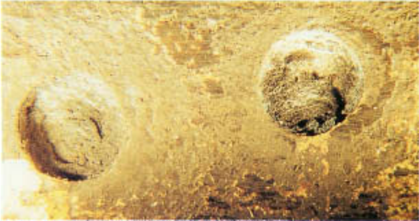
Figure 13.11A Deep, hemispherical “depressions” on the external surface of an overhead condenser due to severe dezincification from internal surfaces (see Fig. 13.11B).
