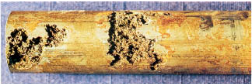
Figure 4.2 Severe localized wastage on a 316 stainless steel heat exchanger tube. Attack occurred beneath deposits, which were removed to show wastage.
