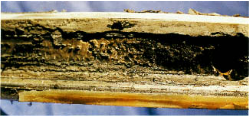
Figure 16.4 Appearance of corrosion along circumference of ring.
