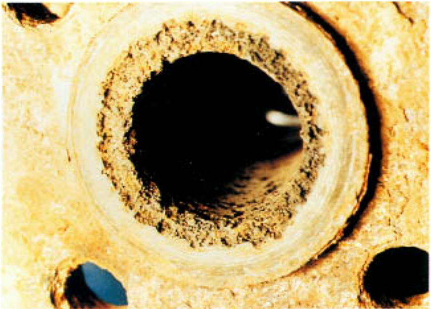
Figure 12.6 Cavitation damage on the discharge side of a regulating valve.
