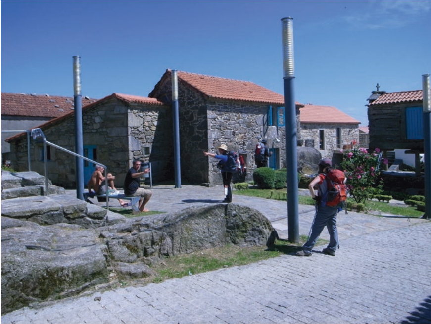
Fig. 6.12 Group of houses restored for the municipal hostel. Source Paula Ballesteros-Arias and Cristina Sánchez-Carretero
