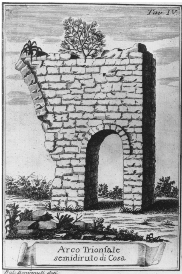
FIG. 47. Fornices, SW half, standing in A.D. 1793
