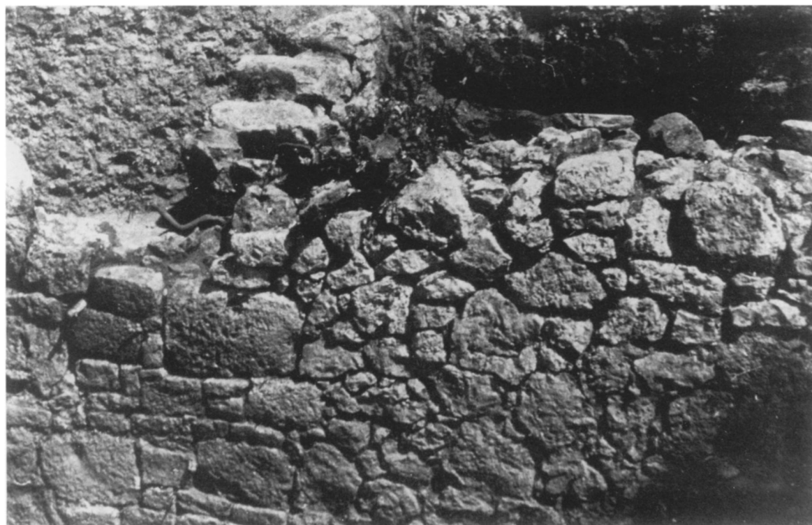
PLATE 100. NW end of SW retaining wall along Street 7, looking SE
