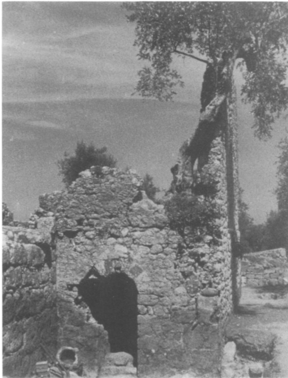
PLATE 229. Basilica, tribunal and vault, looking WNW
