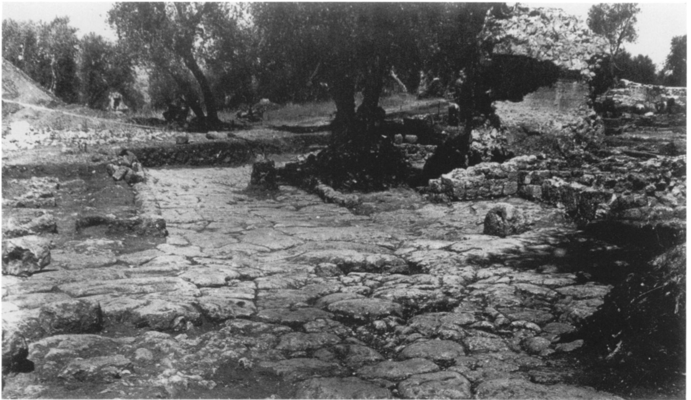
PLATE 87. Streets O and 6, looking NE
