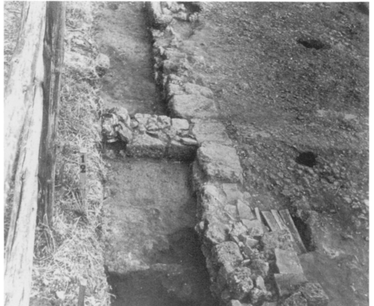
PLATE 62. AB III/IV, party wall and quoins, looking NW
