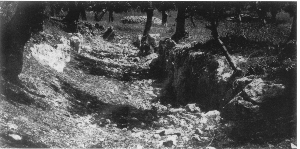
PLATE 2. NW cistern on SW side
