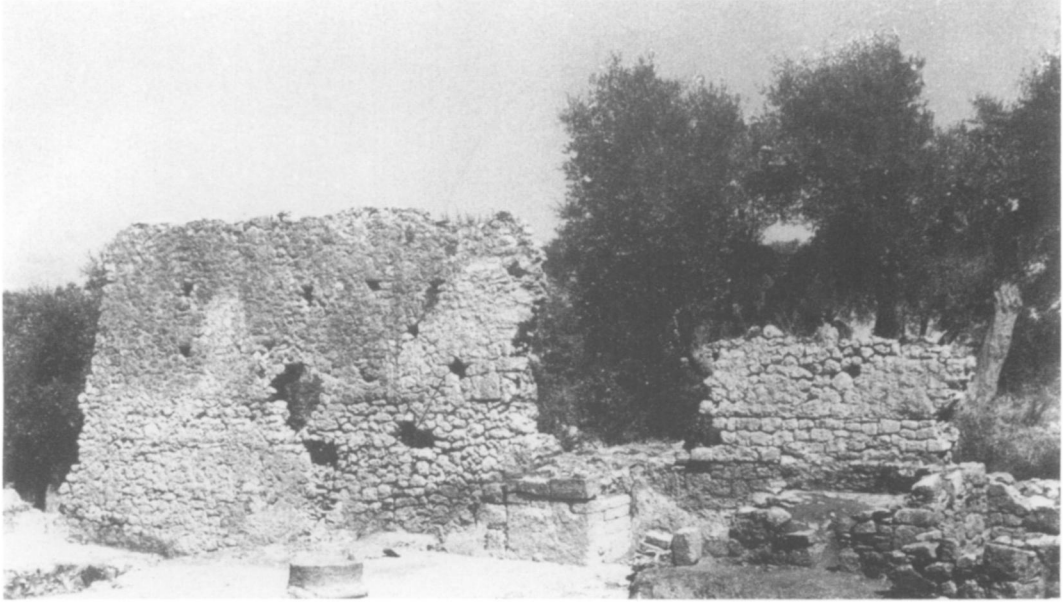
PLATE 231. Basilica, SE wall with putlog holes, looking ESE
