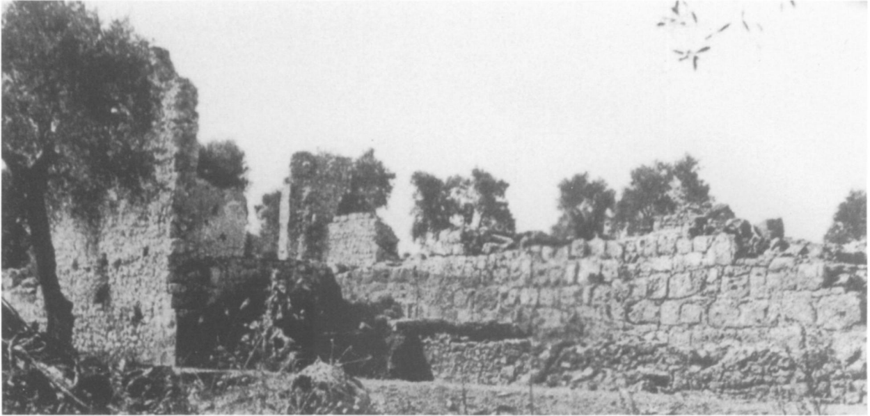
PLATE 228. Basilica, NE foundations and tribunal, looking S
