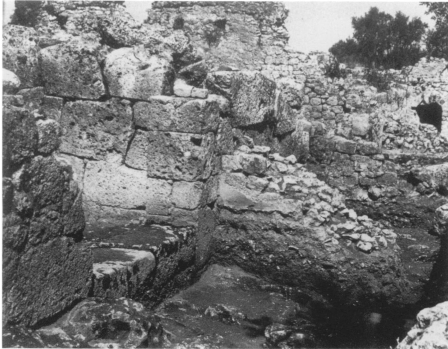
PLATE 103. Curia III, NE wall with buttresses, view looking NW
