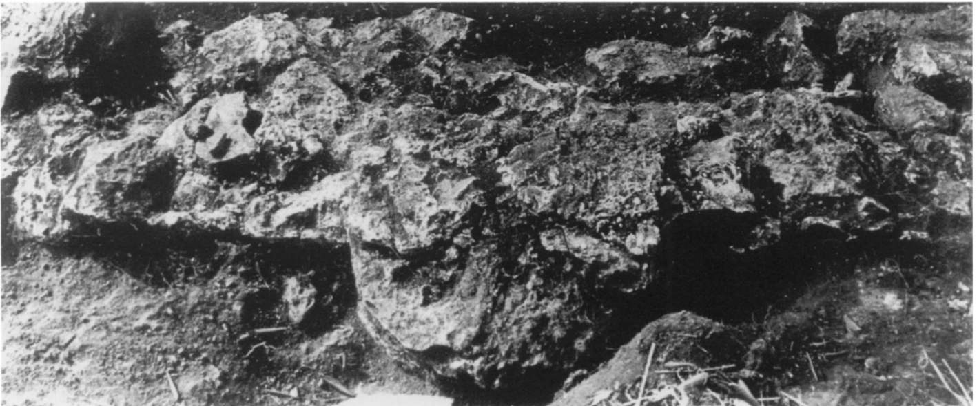
PLATE 70. AB VI, SE wall, engaged half-column, looking SE
