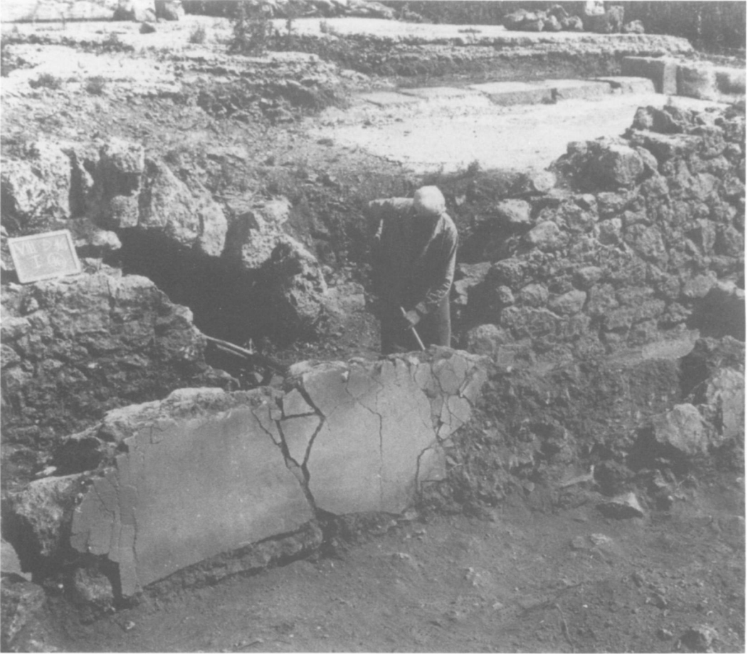
PLATE 248. Basilica, collapsed NW wall
