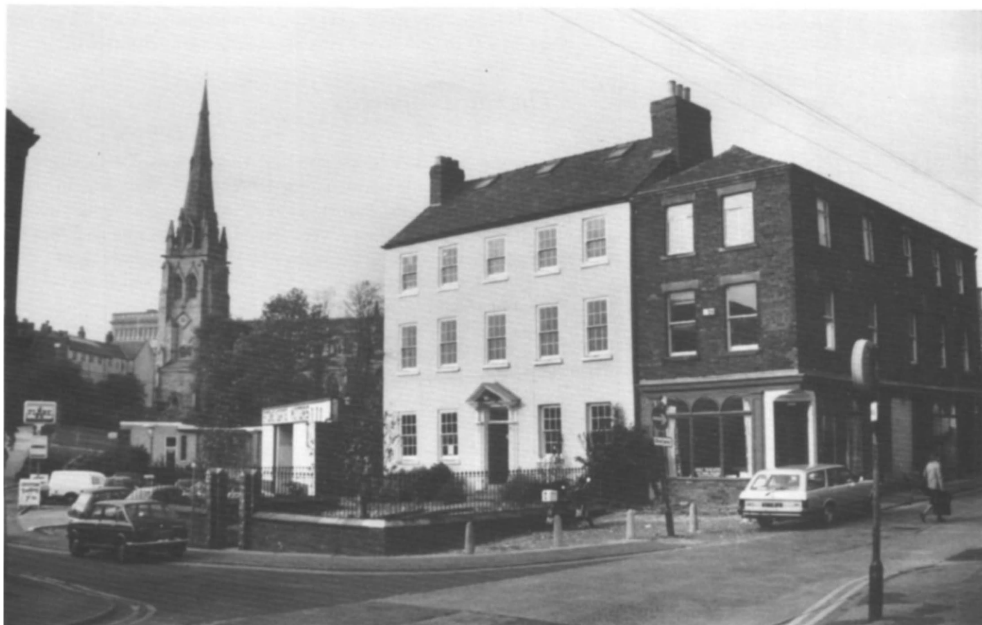
Fig 59 Arkwright House, Preston: rehabilitation completed in 1981; by 1987 the local authority had begun to upgrade the area between the house and the church (photo: Architectural Heritage Fund)
