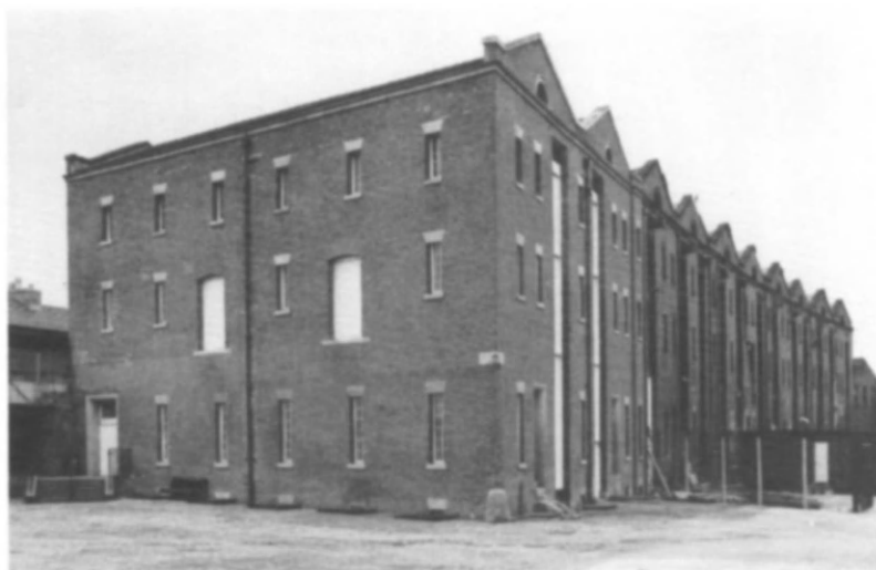
Fig 94 Warehouse, Liverpool Road Station, Manchester: the first two gables, seen in 1988 from yard level, indicate the east bay which was converted for the National Electricity Gallery in 1984 (photo: English Heritage)
