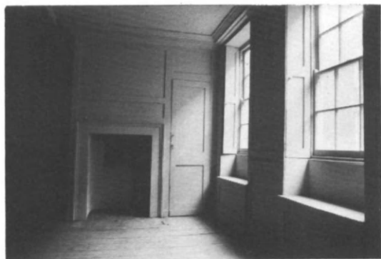
Fig 50 5-7 Elder Street, Spitalfields: repaired panelling (photo: Julian Harrap Architects)
