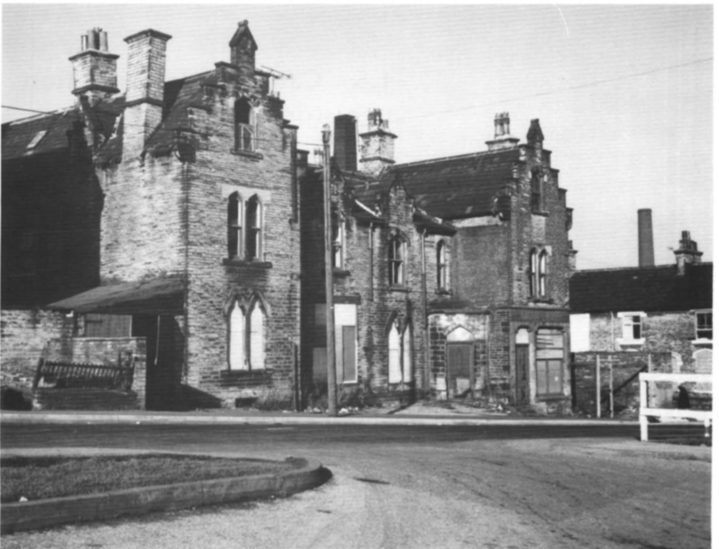
Fig 2 Preston Street, Bradford, bought for demolition and subsequently listed as an early example of cluster block houses
