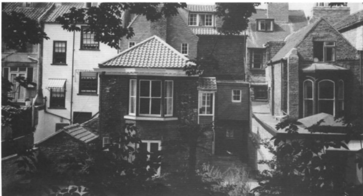
Fig 74 Gillygate, York: a view from the city wall in 1984 after repairs (photo: York City Council)
