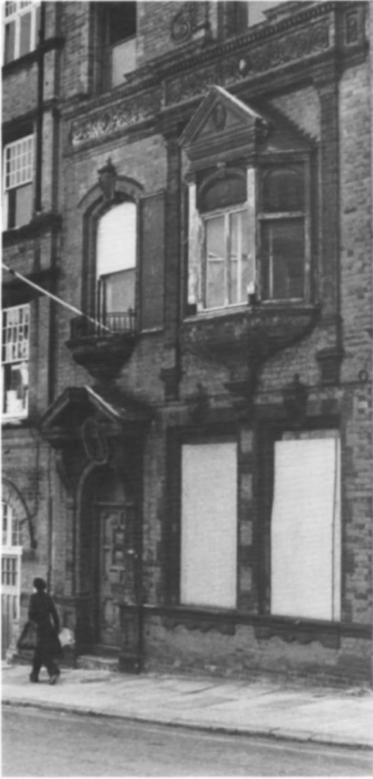
Fig 137 32 Heathcoat Street, Nottingham, before emergency repair; with its fine brickwork concealed by 95 years of grime it blended into a drab streetscape and offered no appeal to prospective users (photo: Nottingham City Council Planning Department)
