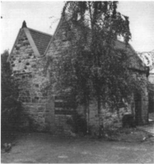
Fig 106 Brandling Station, Felling: the entrance side in 1987 with the side window shuttered and padlocked; beside the entrance door stood the bold and heavy finial which together with its missing partner should have crowned the rear roof
