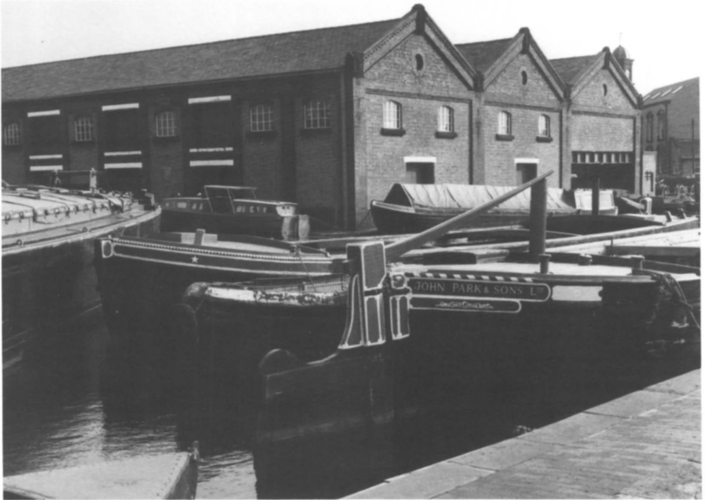
Fig 123 Island Warehouse, Ellesmere Port: the warehouse from the north in 1988
