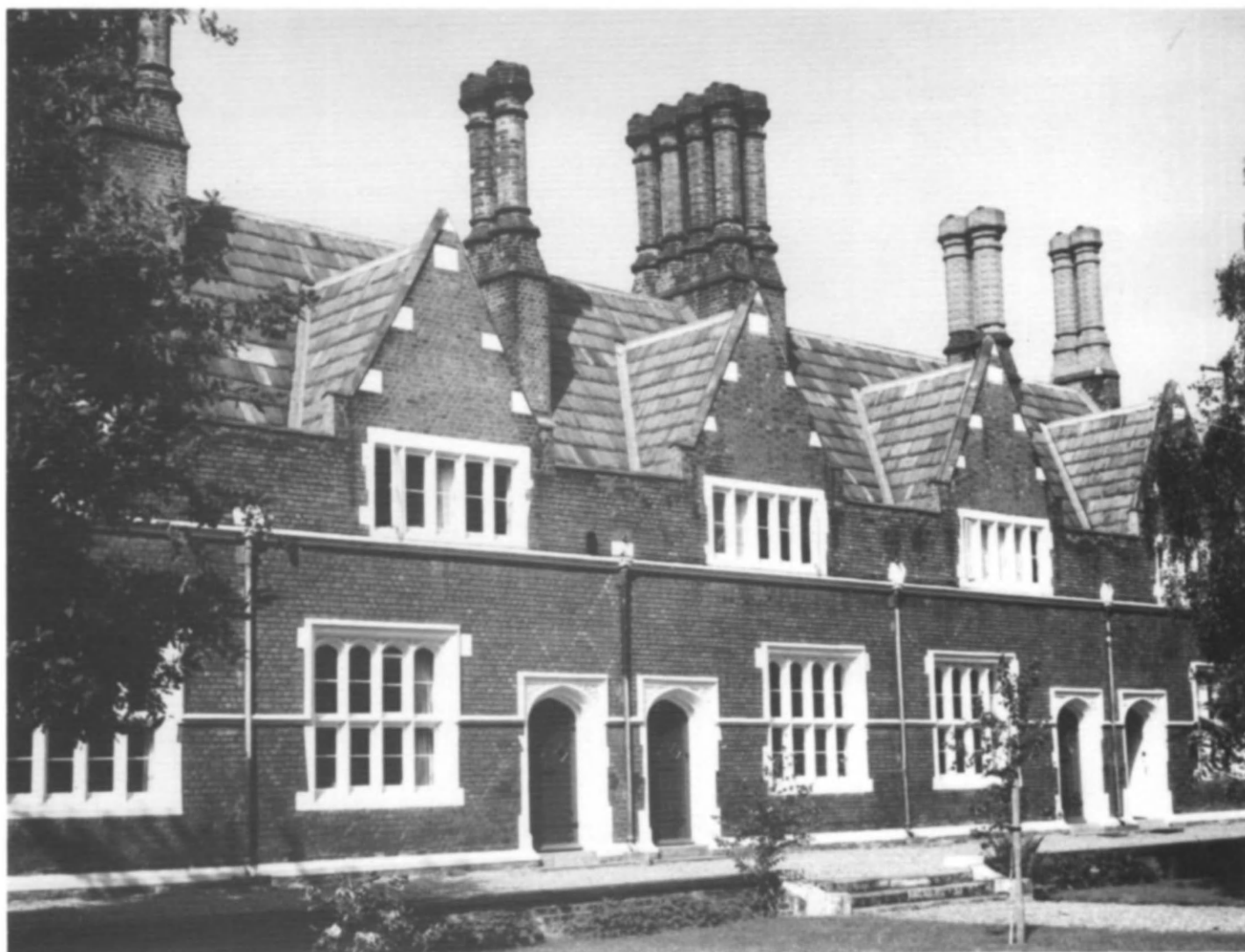
Fig 115 King William IV Gardens, Penge: the central block in 1987, wholly repaired and completely unchanged; the two rebuilt chimney stacks can be seen on the right
