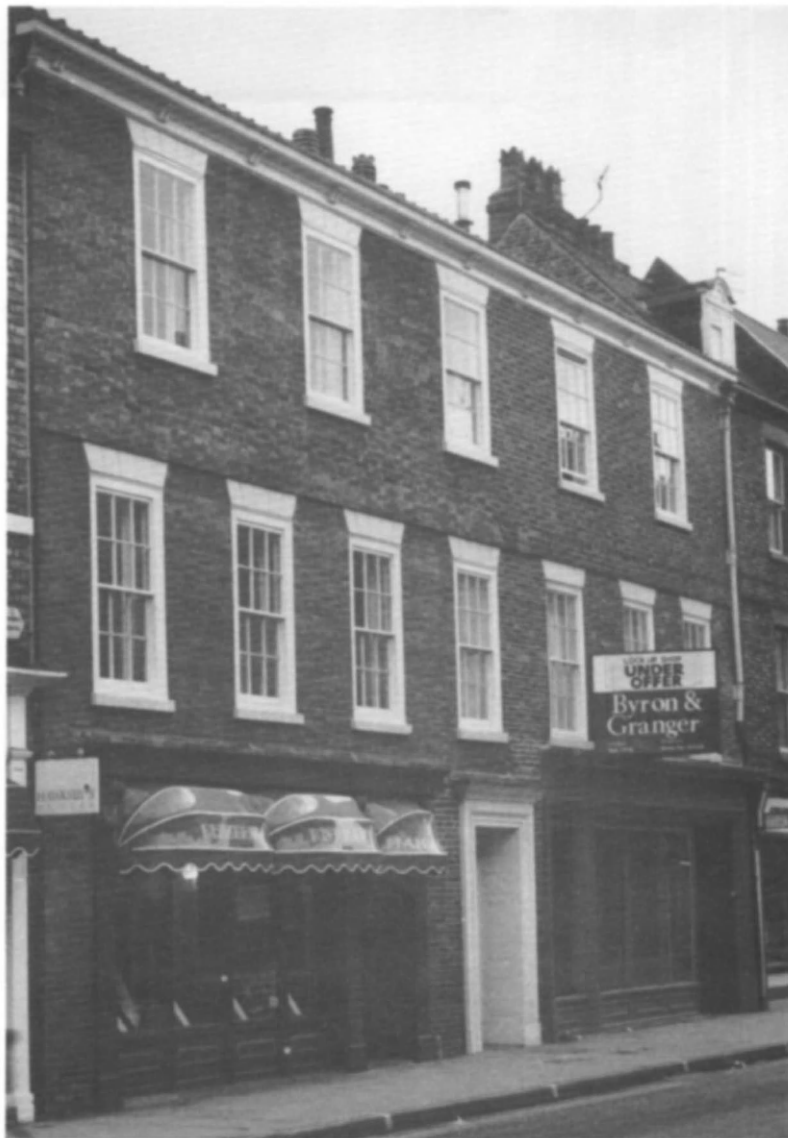
Fig 73 Gillygate, York: numbers 16–20 in 1987, with the seven first floor windows showing the extent of the original early eighteenth-century house
