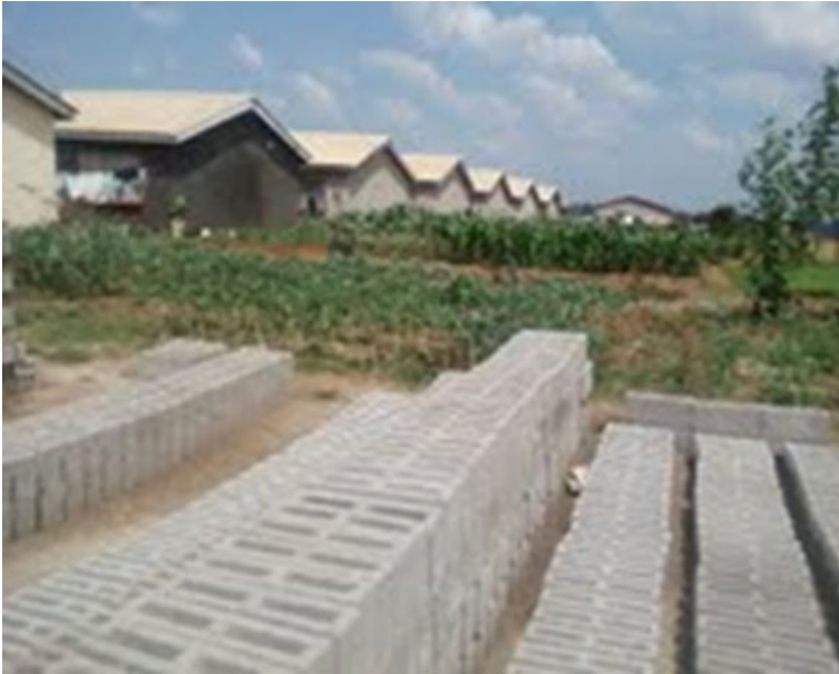
Plate. 4.6 In-situ cement block making for house building ( Source Fieldwork 2012)
