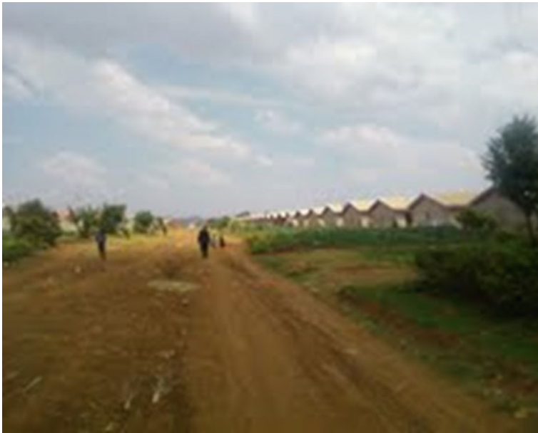
Plate. 4.4 Unpaved access roads—muddy in the rainy season and dusty in the dry season ( Source Fieldwork 2012)
