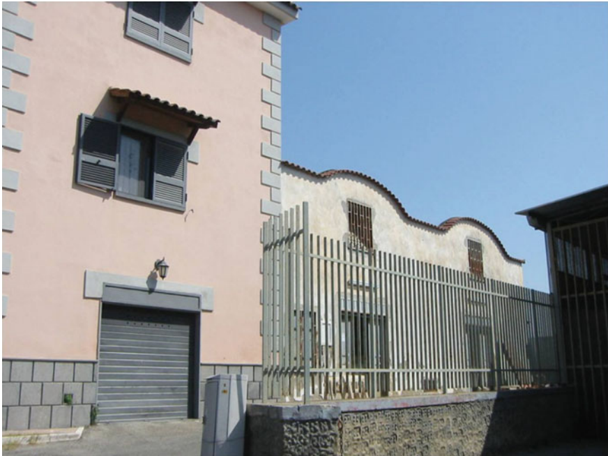
Pozzuoli. A farmhouse after the “restoration” works
