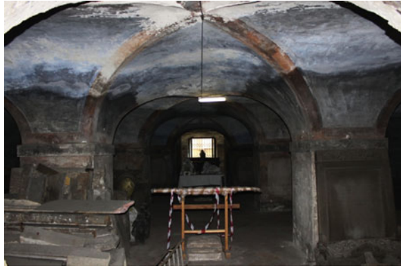
Fig. 5 The central part of the crypt (the “sacello”) before the intervention
