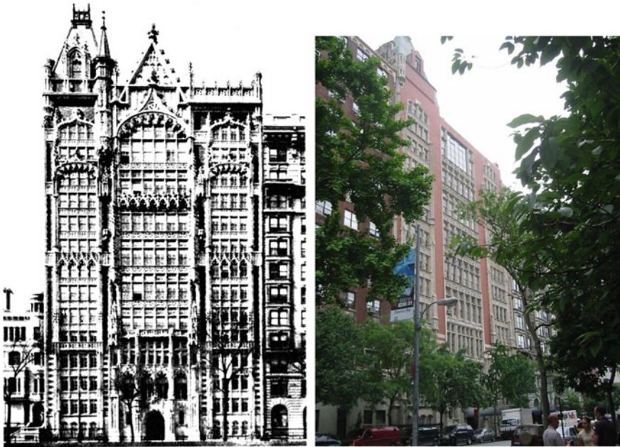
Fig. 1 The upper west side building façade before the majority of the terra-cotta decoration ( left ) was removed in the 1950s and how it looks today after the repair campaign ( right )
