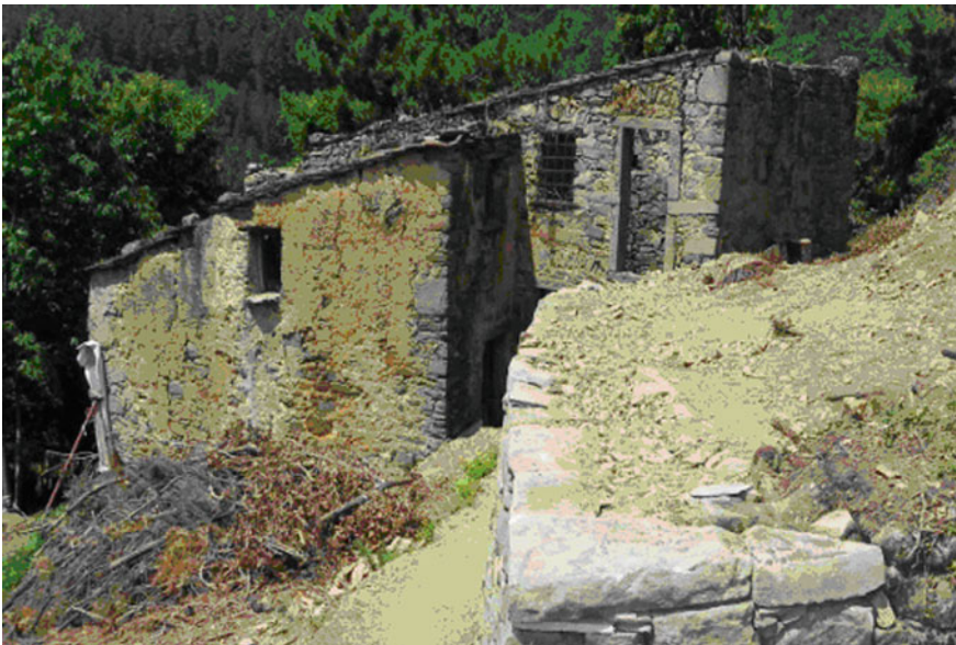
Fig. 2 Case study n. 1 located in Cacinagora. View of the double-cellular building
