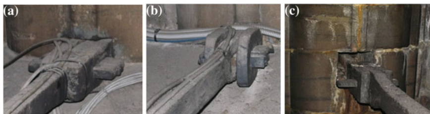
Fig. 2 Typical appearance of ties in the Cathedral of Milano
