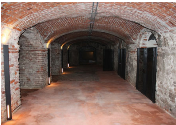
Fig. 6 The “navazzone”, below the narthex, after the intervention, with the “totems” for the lights, the new gates, and the new cocchiopesto pavement
