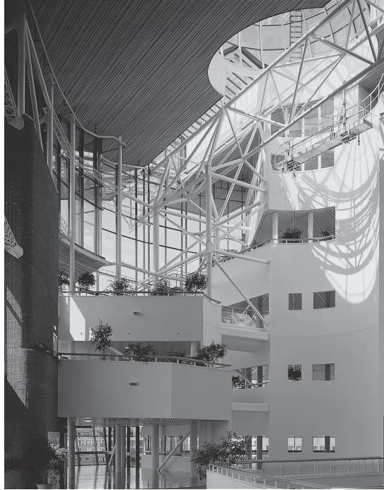
The Ark – interior view: the atrium (copyright Chris Gascoigne/Arcaid)
