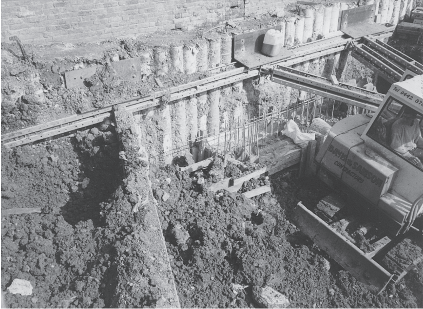
Argent House — groundworks
