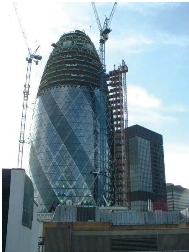
Fig. 3.14 30 St Mary Axe, London. Photo from Structurae: International Database for Structural Engineering, courtesy of Wilhelm Ernst & Sohn Verlag.
