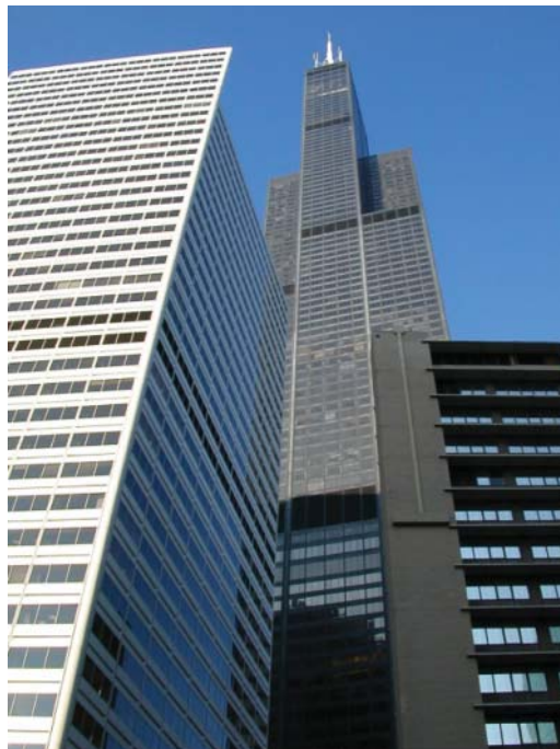
Fig. 3.8 The Willis Towers.
