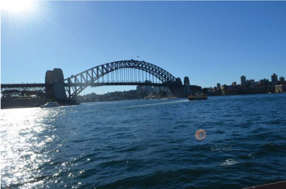
Fig. 9.2 Sydney Harbour Bridge.
