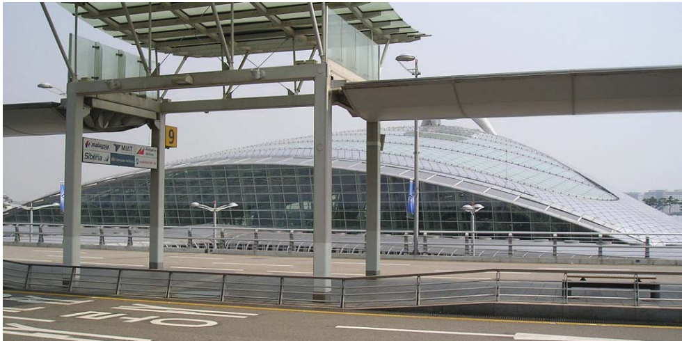
Fig. 8.3 Latticed shell structures: Incheon airport Korea.
