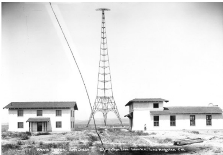
Fig. 7.5 Chollas Heights Naval Radio Transmitting Facility, San Diego, California. Constructed during the Modernization Era in 1917, the Chollas facility was the largest and most powerful radio transmitter in North America. It included three 600-foot tall towers with a copper antenna suspended mid-way between the towers. The facility was the first in the development of long-range transmitter stations between Arlington, Virginia; Pearl Harbor, Hawaii and Cavite, Philippine Islands (U.S. Navy)
