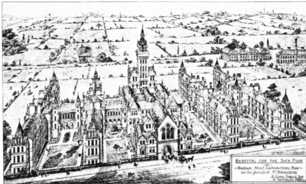
2.5 Aerial view of St Marylebone Workhouse Infirmary, 1879–81, drawn and published by the architect, H.S. Snell, in his ‘Charitable and Parochial Establishments’, 1882, and ‘Hospital Construction and Management’, 1883.
