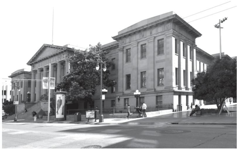
Fig. 2.11 The 1963 demolition of San Francisco's Fox Theater is remembered annually in the city even today, however its destruction can be said to have saved structures such as the Old Mint, illustrated here, and the Presidio, discussed in Chapter 5. (Author's photograph)
