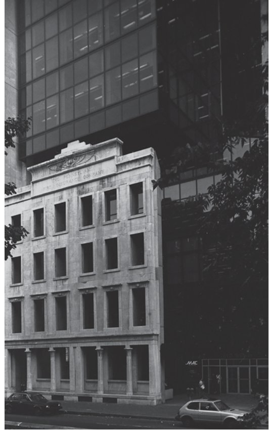
Fig. 7.6 All but the Egyptian Revival front of the Pennsylvania Fire Insurance Company was removed to make way for the Penn Mutual Life tower, a 21 story office building erected in 1971–1974. It serves as a four-story, freestanding sculpture defining the new building's entrance plaza. (Author's photograph)
