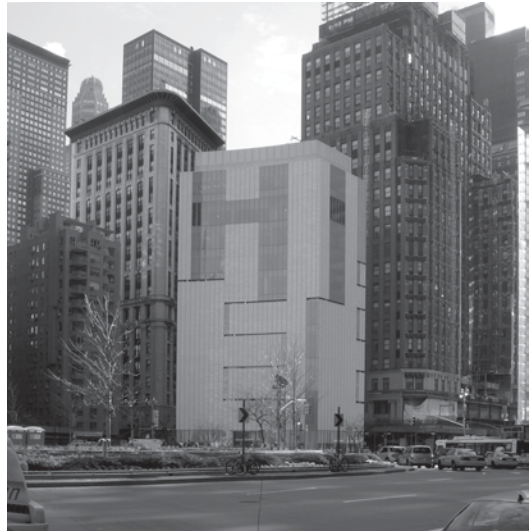
Fig. 7.12 The famed “Lollipop Building” on Columbus Circle could not be landmarked because the New York City administration blocked the Landmarks Commission from holding a hearing, despite the appeals of local preservation organizations. (Author’s photograph)
