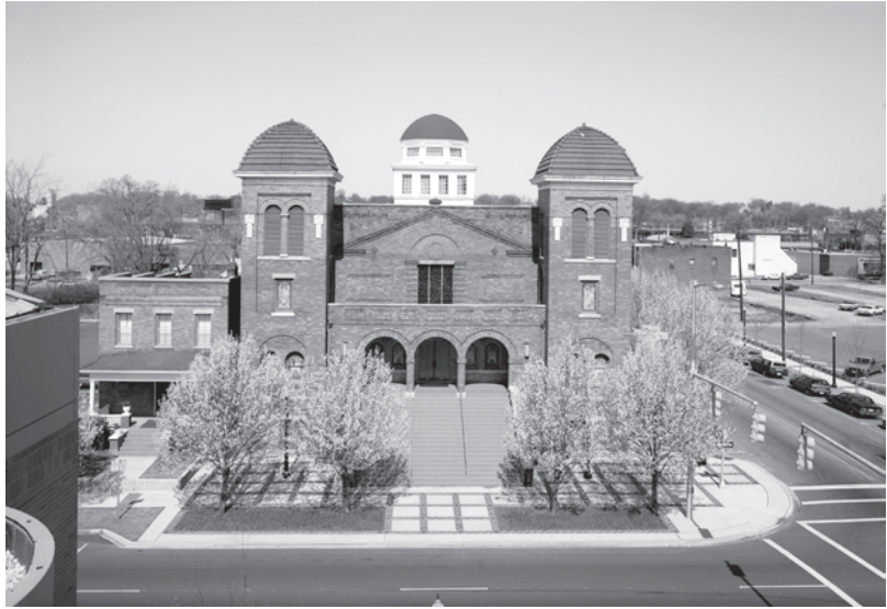
Fig. 3.4 The Sixteenth Street Baptist Church in Birmingham is one of two locations intimately associated with Dr. Martin Luther King, easily recognized for the historical associations with the Civil Rights movement. (Historic American Buildings Survey, Library of Congress)
