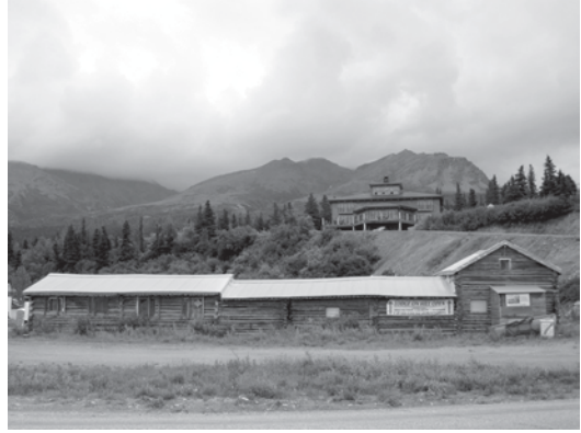
Fig. 6.2 The Rapids Roadhouse, a remarkable survival on the Delta River, 231 miles from Valdez, AK, was established in 1902 as a log cabin that continued to increase in size and change with the various uses it has served. (Photograph: Casey Woster)
