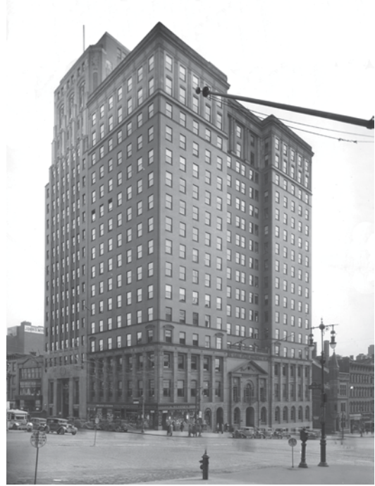
Fig. 7.5 In 1926, when the Albany State Bank directors decided to build a new 16 story office building, they asked their architect Henry Ives Cobb to keep the original 1803 façade with the result that it was jacked up and moved to its new location, to form the entryway. (Author’s collection)
