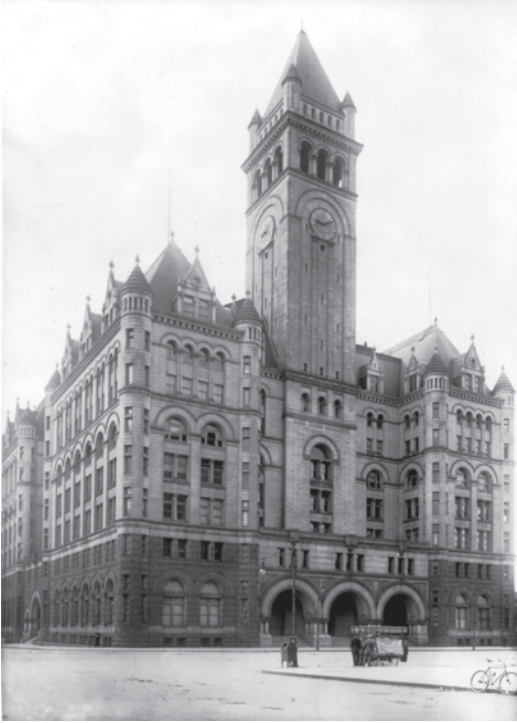
Fig. 2.25 On Pennsylvania Avenue in Washington, D.C., the Romanesque Old Post Office was threatened with demolition but preservationists led a campaign not only to save it, but other surplus public buildings. (Historic American Buildings Survey, Library of Congress)
