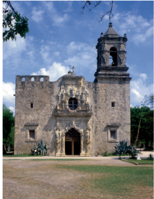
Fig. 1.29 In addition to the Alamo, the other four extant missions needed considerable repair and restoration. San Jose y San Miguel de Aguayo's dome and roof collapsed and the Daughters of the Republic of Texas worked with the Catholic Diocese to raise needed funds. (Author's photograph)
