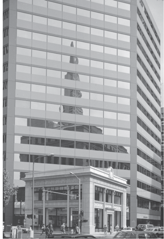
Fig. 2.26 In San Francisco, the White Investment Building was one of the first to be all but completely destroyed, despite the best efforts of the preservation community. Saving only the fronts gave rise to the term “facadism.” (Author’s photograph)
