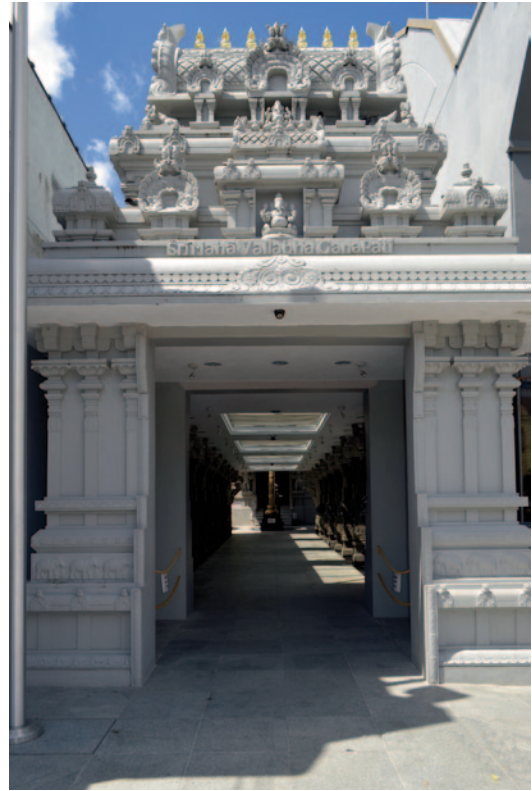
Fig. 8.15 The Maha Vallabha Ganapathi Devasthanam, in Flushing, Queens, is the oldest Hindu temple in the country, largely constructed of imported materials and assembled by artisans from India. (Author's photograph)
