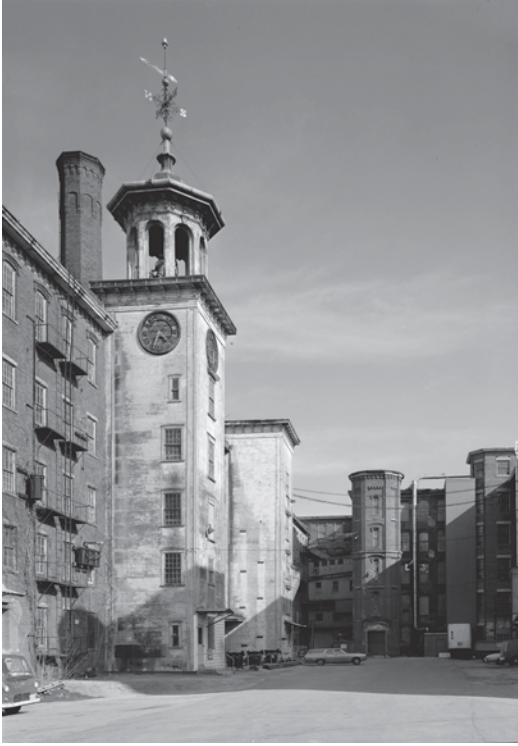
Fig. 4.4 Boott Mill Tower, one of the most notable elements on the skyline of Lowell's industrial waterfront, at the confluence of the Merrimack and the Concord Rivers. (Jack Boucher, photographer, Historic American Engineering Record , Library of Congress)
