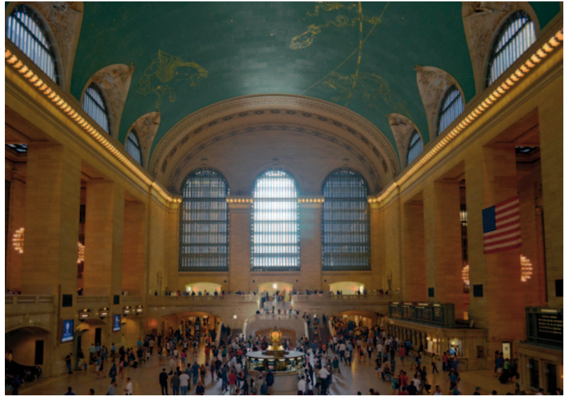
Fig. 3.12 The interior of the Grand Central Station is one of the most striking interior public spaces in the country, recently restored and rehabilitated with comparatively minor changes. (Author's photograph)
