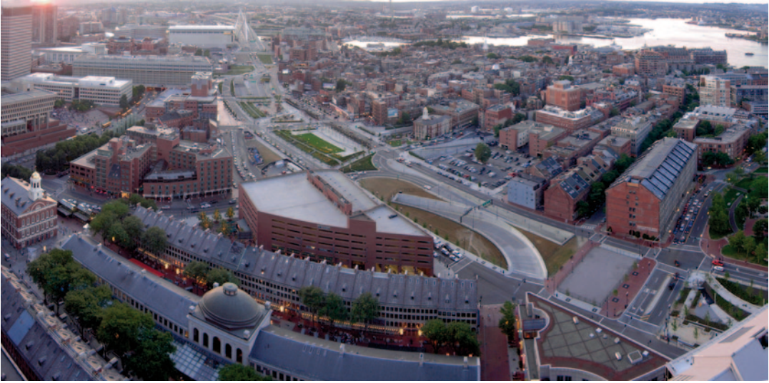
Fig. 6.13 Submerging the central arterial highway in Boston in a project that became known as “The Big Dig” began in 1991 and continued until 2008, a massive project. Existing buildings, subway lines, and highways had to
