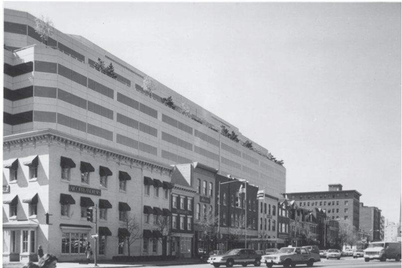
Fig. 7.10 Each of the buildings in Red Lion Row were deliberately “facadimized” to build a much larger structure that would generate rental income, with some doors and windows that are simply used as decoration. (Author’s photograph)
