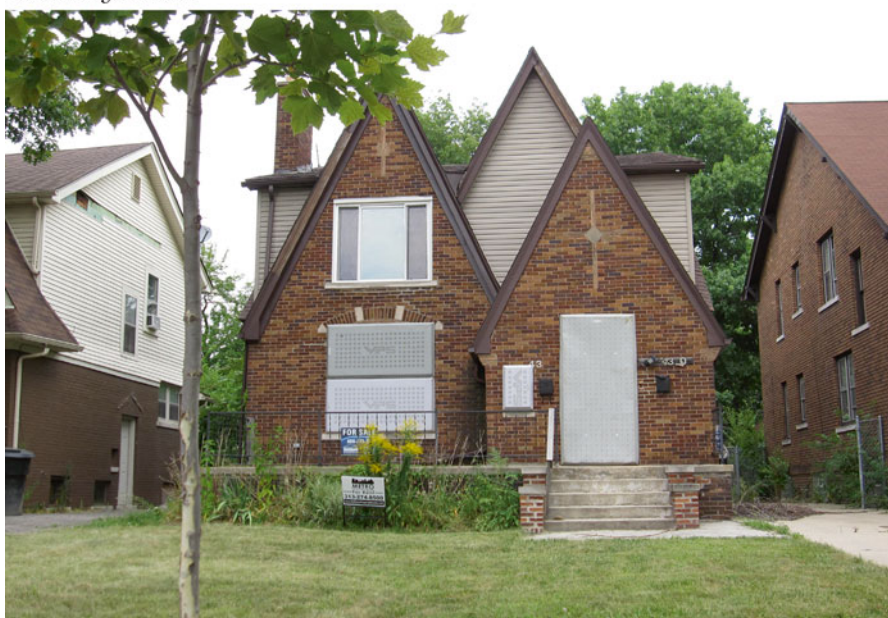
The investor who owns this house has secured it to prevent vandals from stripping out its plumbing and fixtures. Photo: Margaret Dewar
