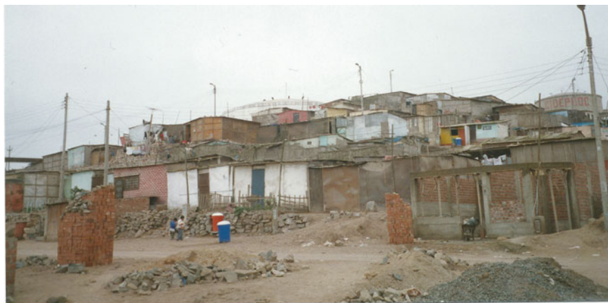
Photo: Diana Burgos-Vigna Very poor condition of recently built areas (called «asentamientos humanos» in spanish)
