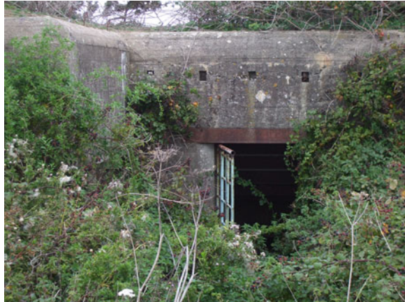
Fig. 3.7 Neglected bunker in Alderney, 2010 (© Gilly Carr)
