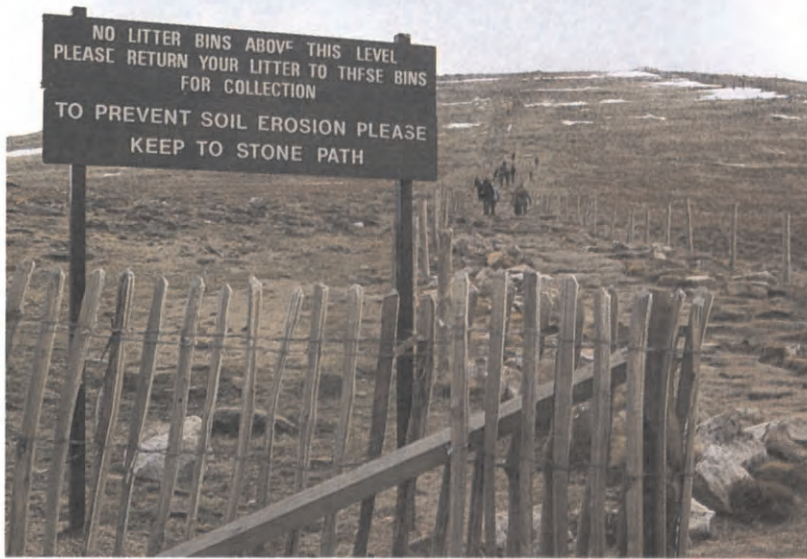
K Footpath erosion on the summit path to Cairn Gorm
