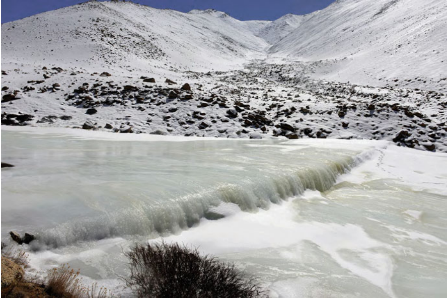
Fig. 9.6 Artificial glacier at 4,420 m (14,500 ft), located above the village of Igu, Ladakh. The masonry wall in this construction is completely submerged by ice (Photograph by M. Nüsser, February 25, 2014)
