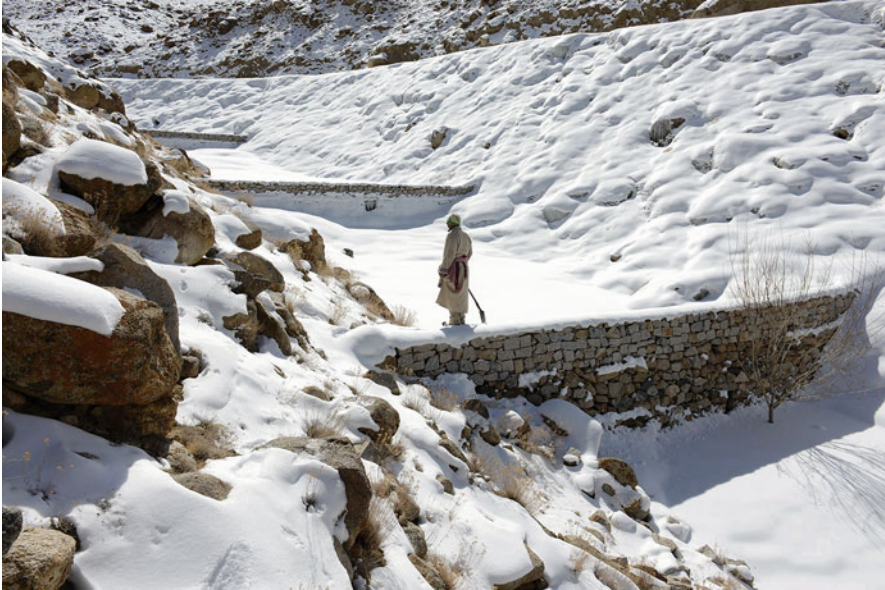
Fig. 9.5 Artificial glacier at 3,900 m (about 12,800 ft), located above the village of Nang, Ladakh. The cascade is composed of a series of loose masonry walls ranging in height from 2 to 3 m (6½ to 10 ft), which help freeze water for storage (Photograph by M. Nüsser, February 20, 2014)
