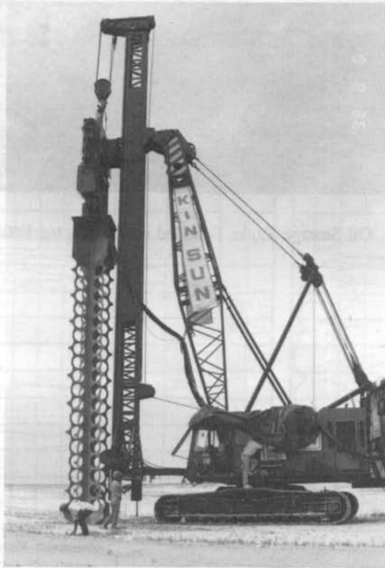
Fig. 3.23 The Resonance Compaction Equipment
