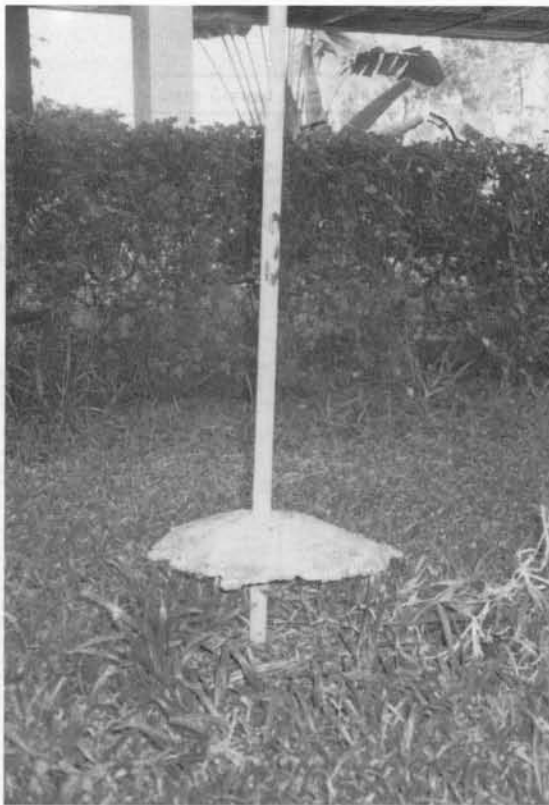
Fig. 1.8 Deep Settlement Marker Showing Compression of Soft Clay Layer
