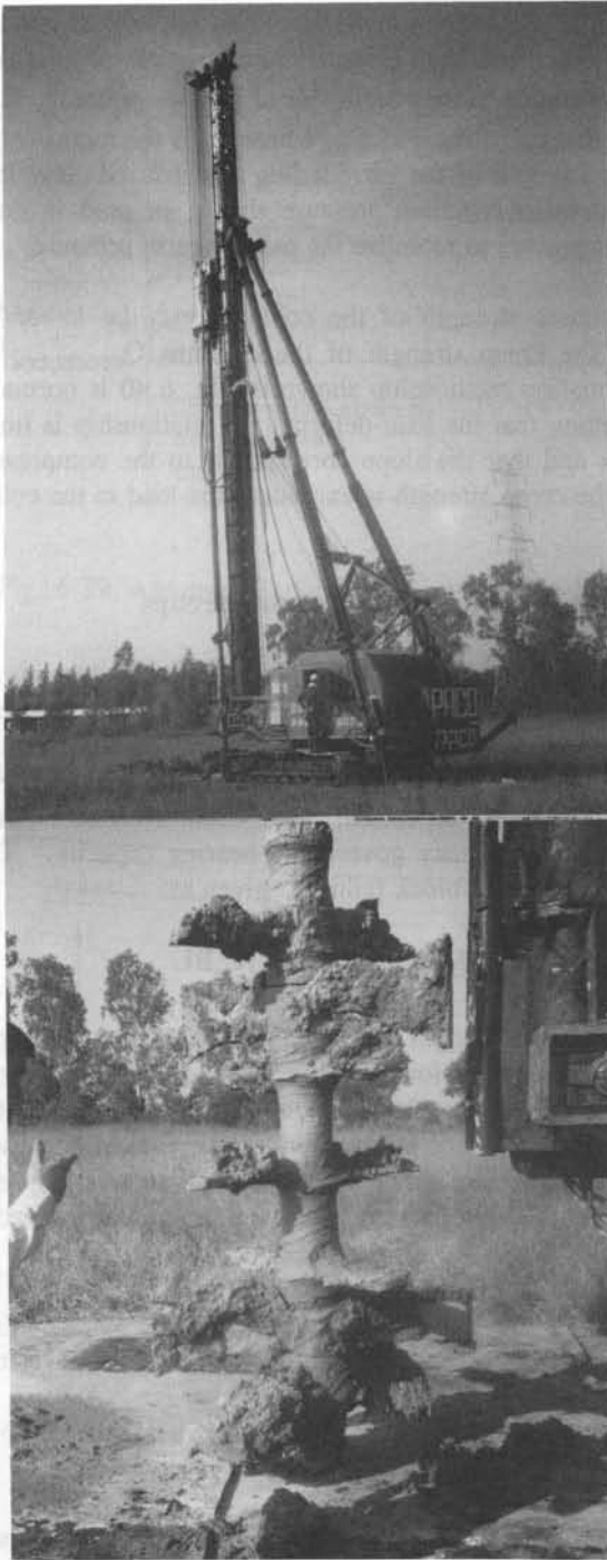
Fig. 6.38 Installation of Cement Piles by DMM Method
