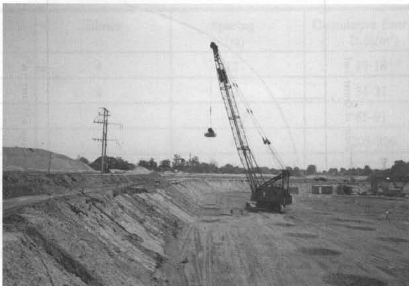
Fig. 3.42 Actual Application of Dynamic Compaction for Dam Rehabilitation in Thailand
