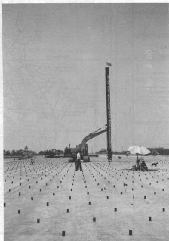
Fig. 4.47 PVD Installation
