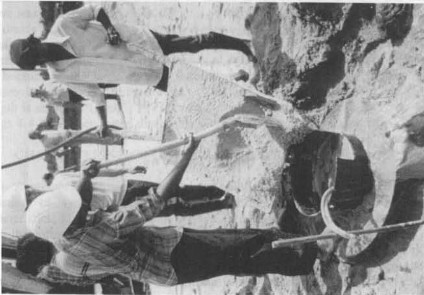
Fig. 4.4 Non-Displacement Sand Drains Using Water Jets
