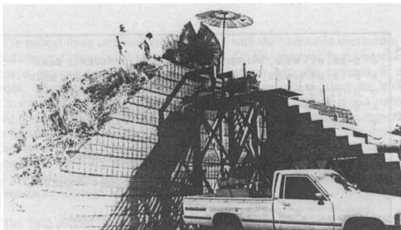
Fig. 7.35 Typical Set-Up of Field Pullout Test
