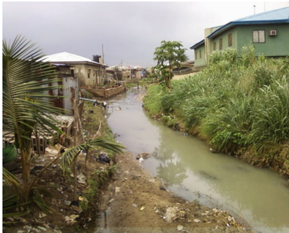
Fig. 8 A house at Ajiliti located on slopes very close to a stream
