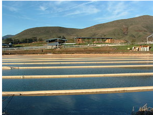
Fig. 6.13 Anaerobic lagoon and generators at the Cal Poly Dairy, USA 2003; 25 kW Power plant is fired using the biogas (photo by Kjkolb, From Wikipedia, Free encyclopedia)
