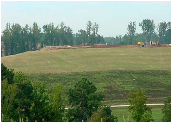
Grass and other plants cover the municipal solid waste landfill.
