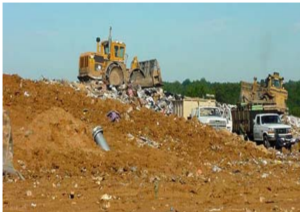
A bulldozer prepares
