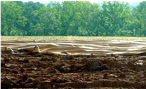
An experimental tarp provides daily cover of the landfill cells.
