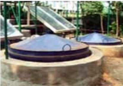
Fig. 9.7(a) Biogas Unit at BARC (Courtesy: Mahadevia, D)
