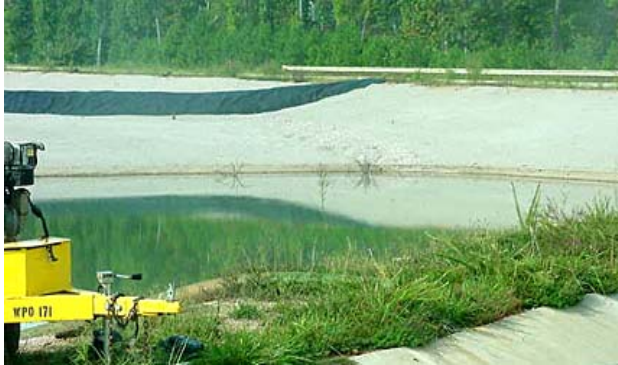
Collection pond catches storm water
