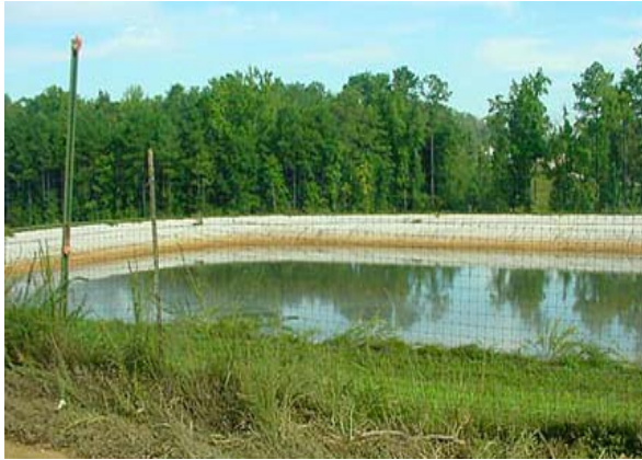
A leachate collection pond catches the contaminants that can get into water that goes through the trash in a landfill
