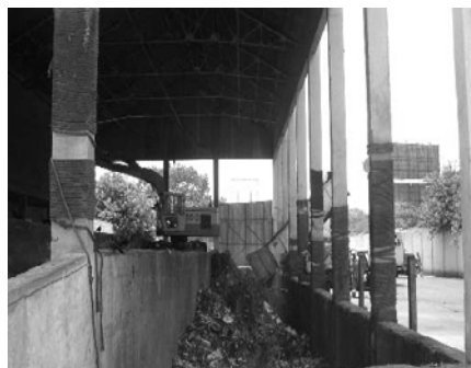
Fig. 9.2(d) Transfer station
