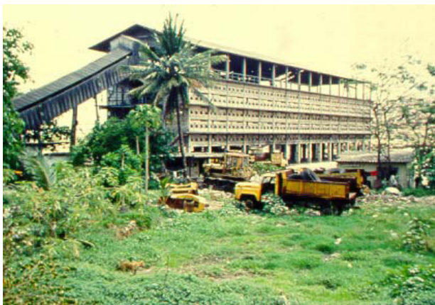
Fig. 5.10 Composting Plant in Bangkok, Thailand
