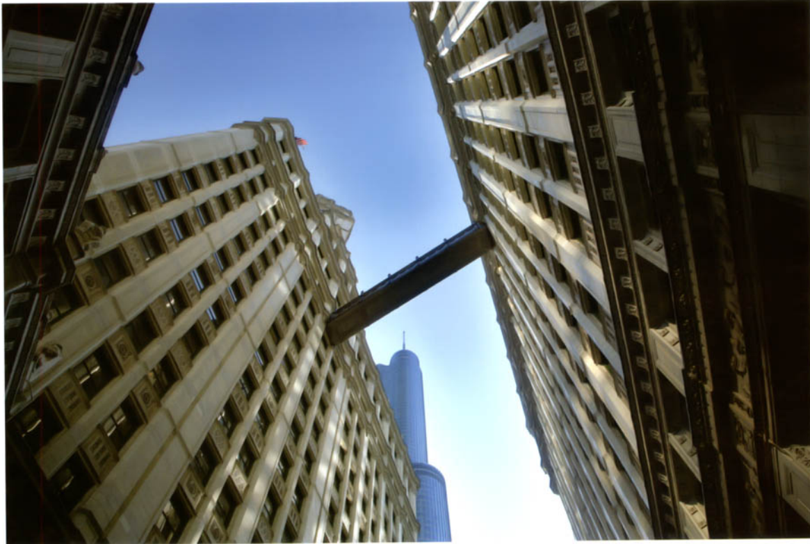
Example of Bridge Spanning Between Buildings
