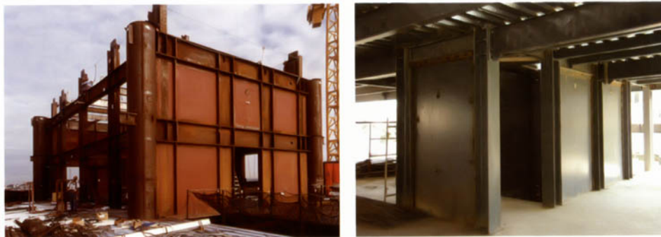
Special Steel Plate Shear Walls
