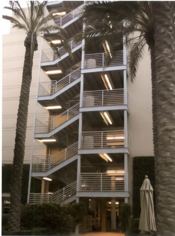
Example of Egress Stairway Not Part of Building Structure
