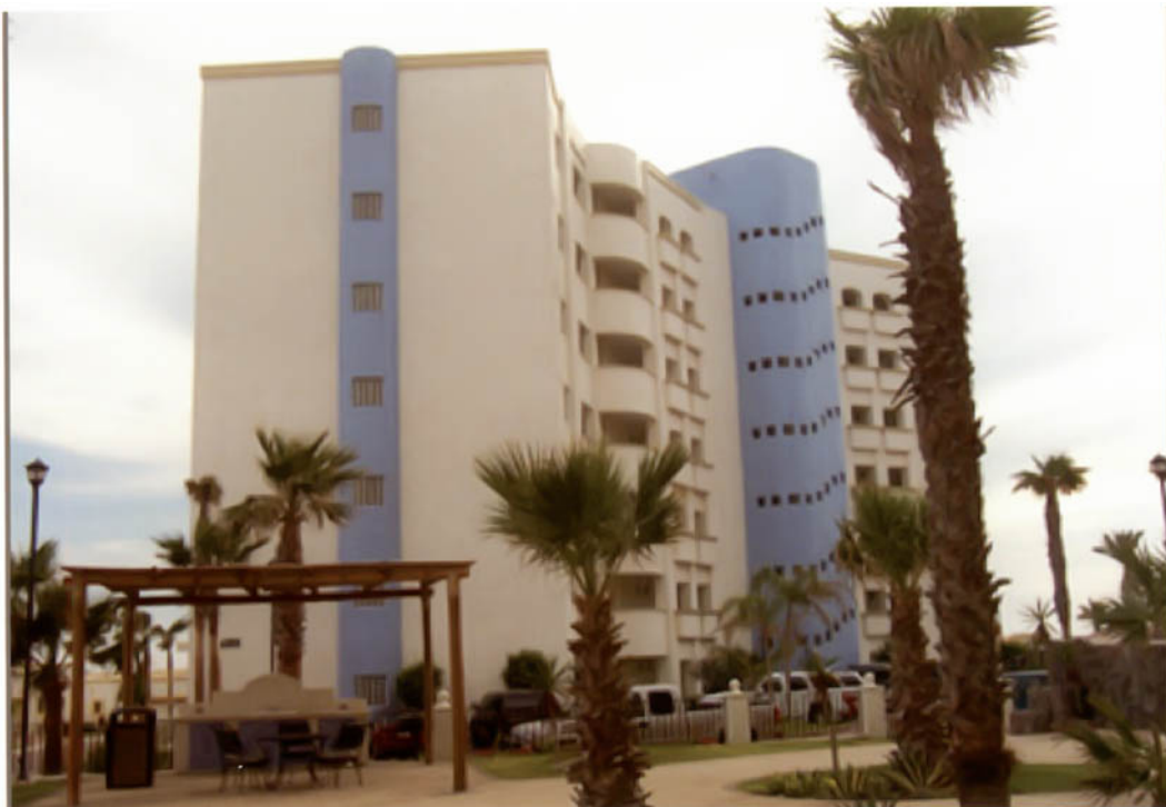
An AAC masonry hotel in Las Palmas, Mexico, where AAC masonry elements are used as structural members as well as cladding Courtesy: Autoclaved Aerated Concrete Products Association
