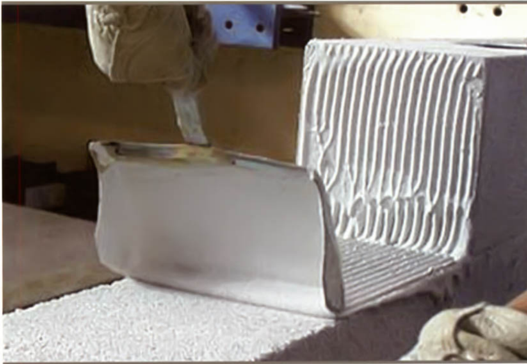
Laying AAC masonry units using thin-bed mortar and toothed trowel www.masonrymagazine.com
