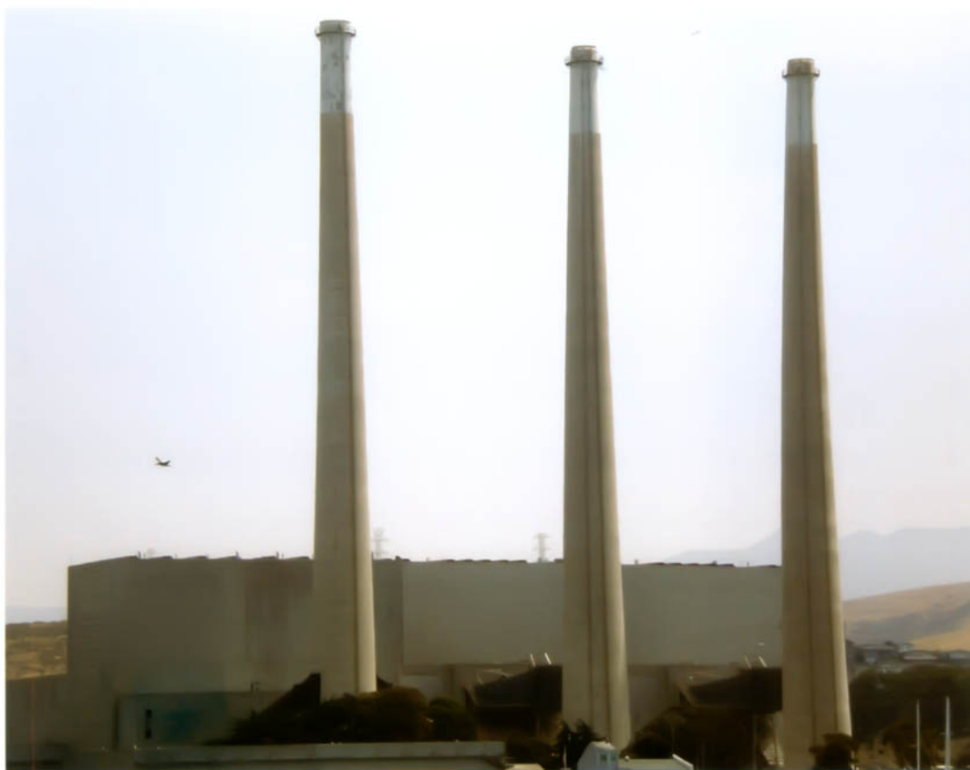
A new entry is added to Table 15.4-2 for concrete chimneys and stacks designed in accordance with ACI 307.
