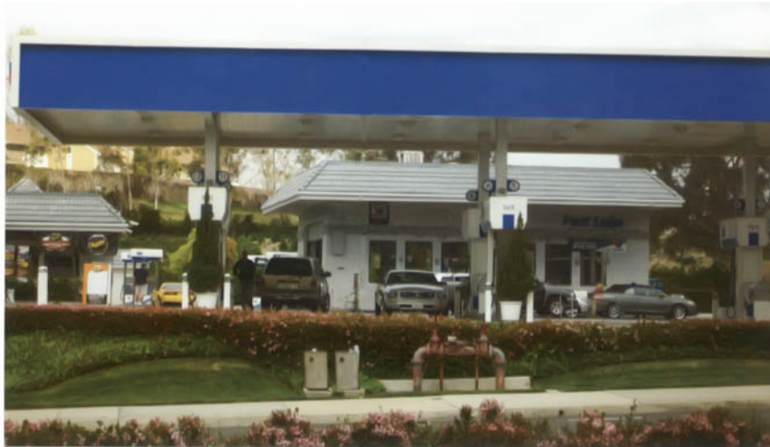
Gas station canopies are typically cantilevered column systems.
