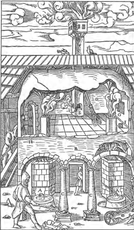
Fig. 1.1. Diagram of a dust chamber in the Ore Mountains (1556)[2], by courtesy of the VDI Commission Air Pollution Prevention
