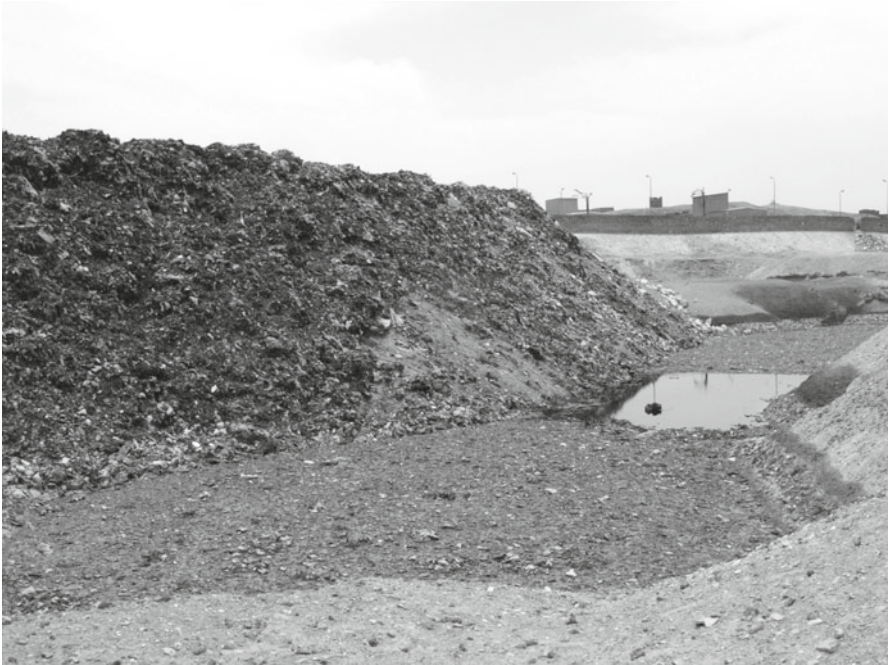
Fig. 7 Debris slopes marked with dummy excavations that have since filled with ground water seepage (photo: author)
