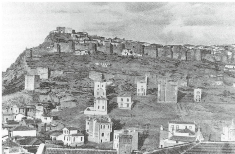
Fig. 7 The burned Hisarönü district in the early 1920s, with some new construction after Ankara became the capital. However, the scars of the fire are quite visible (Source Ankara Municipality, Ankara in Postcards)
