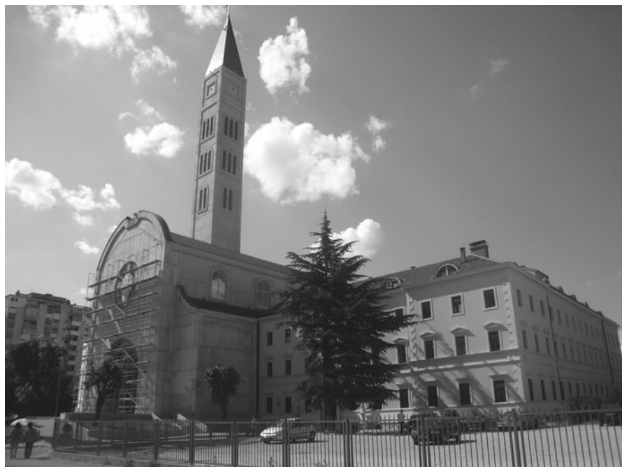
Fig. 5 Franciscan church, bell tower, and monastery complex after reconstruction (image: author, 2011)
