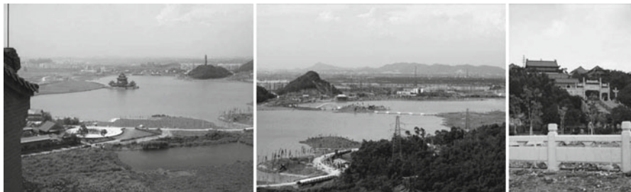
Fig. 9 Qingyun Lake and Baolin Temple under construction (photos: Andrew Dribin, Carl Wohit and Sarah Brady)
