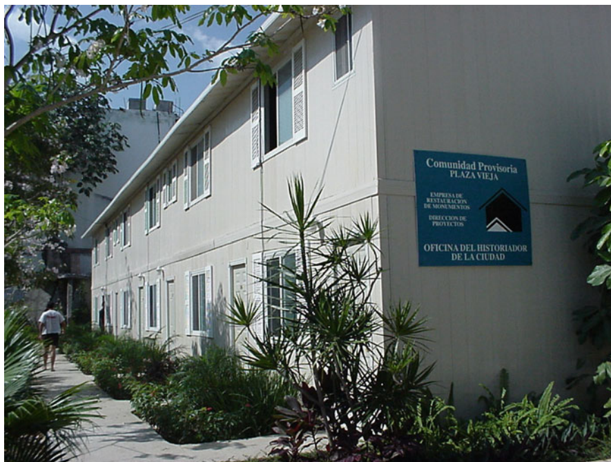
Fig. 7 Temporary pre-fab housing, one block from Plaza Vieja in Habana Vieja. These Canadian-built modular units are small but offer solid housing while locals await housing reassignment outside the neighborhood or else return to their remodeled home, done by the City Historian Office (photo: Scarpaci)
