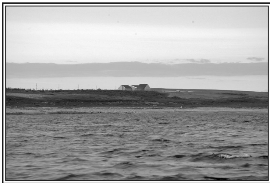
Fig. 14.11 Port au Choix National Historic Site Visitor Centre, which can be seen as a peak on the horizon for a distance of several kilometres as one travels the coast by road or water
