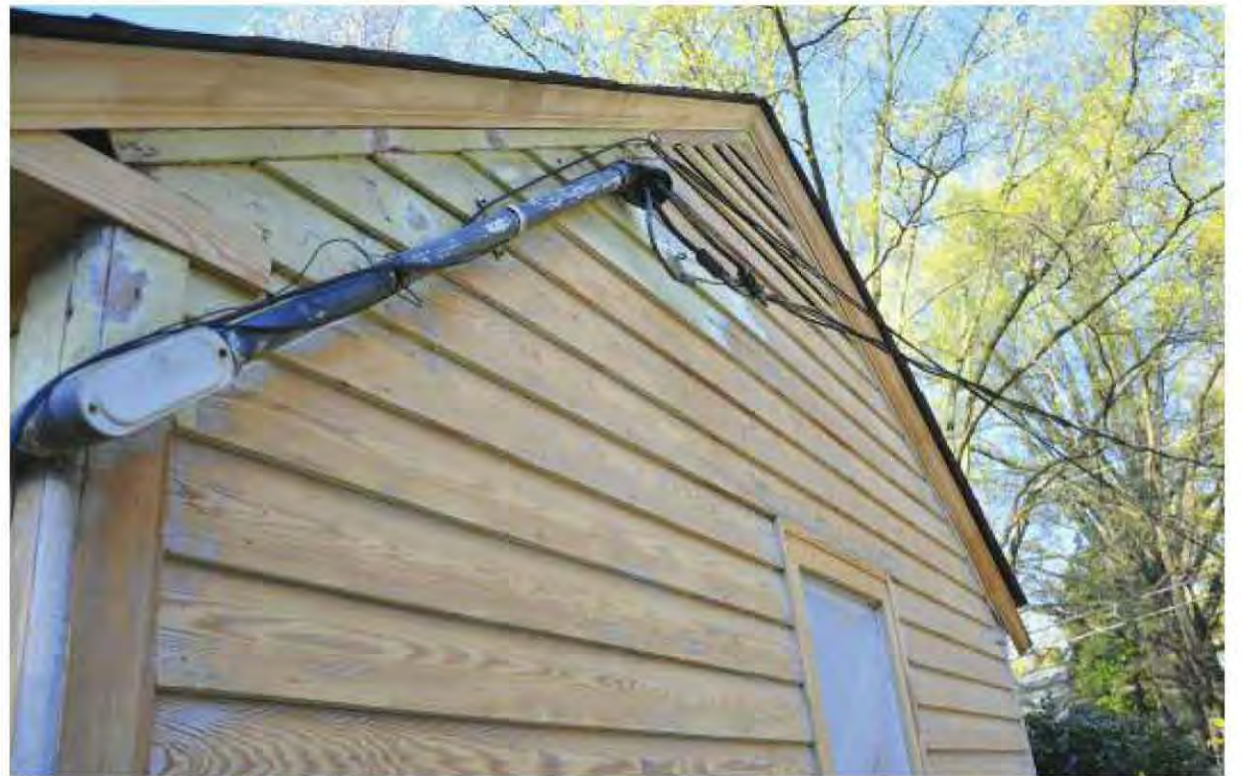
Fig. 14.2-3: Electricity comes to the home through an elevated weather-mast, through protective conduit to the meter and on to the circuitry panel. Generally speaking the homeowner is responsible for all maintenance beyond the meter, and the utility for everything on the other side.
