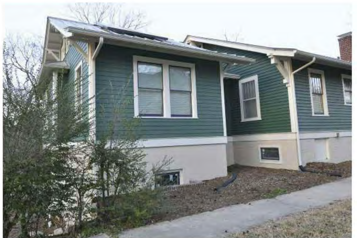
Fig 2.4-5: The addition to this 1920s bungalow was designed and constructed to complement the original house in style and massing, while differentiating with a roof break and window detail. The door connecting the old and new was purposely kept in place to preserve the original structure (consistent with SISR 10).
