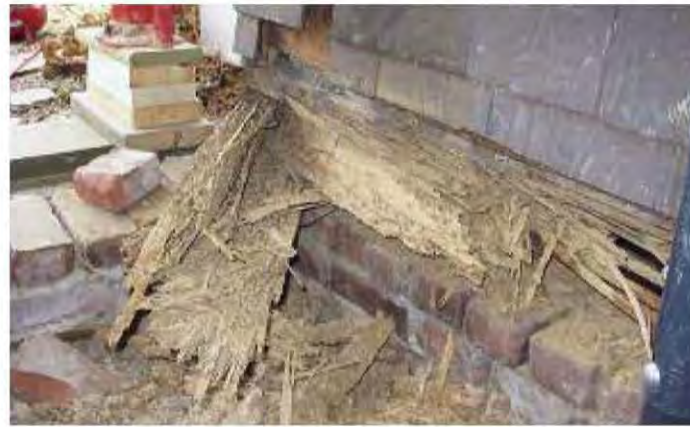
Fig. 9.21-22: Termites love a good, wet sill beam. Bottom, termites are attracted to beams saturated by water not from the ground, but from a leaky radiator. Inside, the girder, sillbeam and floorboards all show clear termite tunnels and stalactites.
