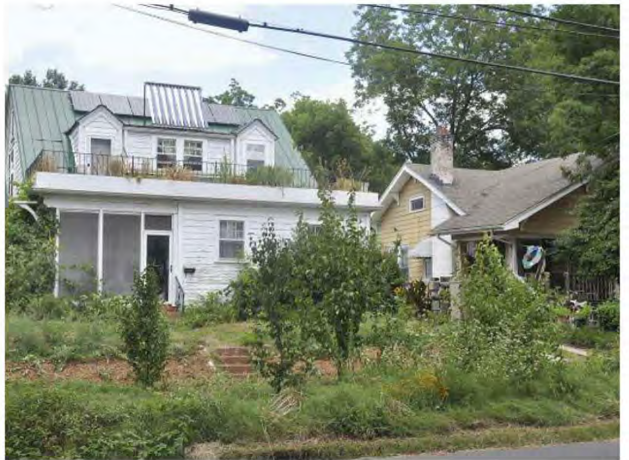
Fig. 14.23: This historic bungalow is one of the greenest old houses in my part of the US, featuring a range of technologies that take the home off the grid. The solar panels on the street façade, however, disqualified it from receiving tax credits. As this book went to press, this state's SHPO was reconsidering their position on roof panels, though even under the more lenient criteria being considered this particular design would still be considered too obtrusive to qualify.
