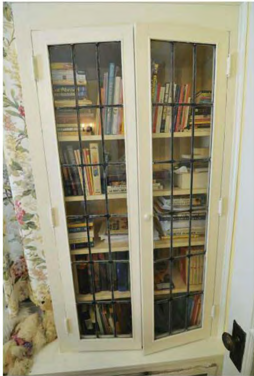
Fig. 6.27: Original built-ins should be preserved in place. The glass may be too valuable and fragile to move.
