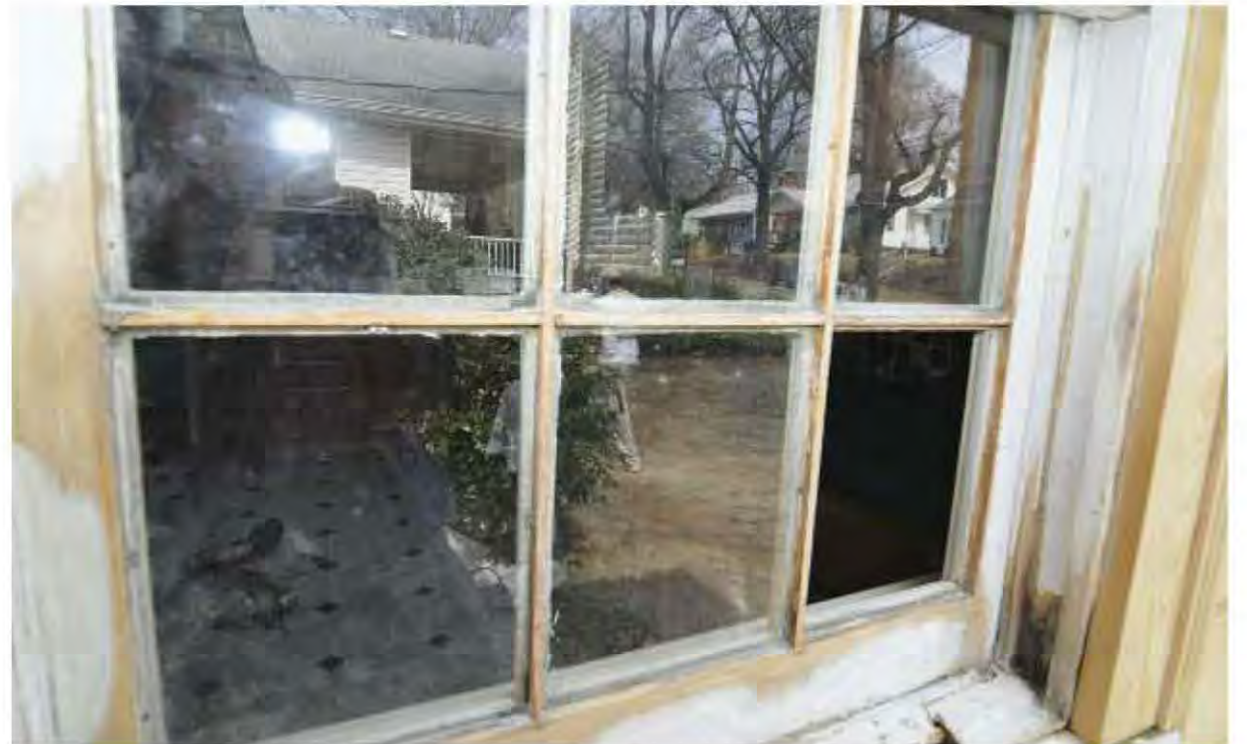
Fig. 11.18-19: When exterior window glazing falls into disrepair, reglazing is required. The old glazing is removed, the new glazing installed and a doughy putty is applied and cut at an angle to minimize the profile. Glazing is being installed at left, and new glazing is completed at right.
