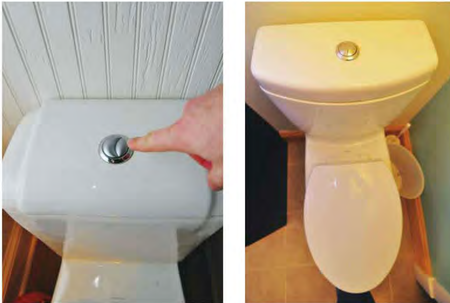
Fig. 4.15-16: A dual flush toilet has two buttons, allowing the user to choose how much water is necessary to clear the contents of the bowl. Sometimes a challenge to design cohesion, most efficient toilets tend to be very modern looking.
