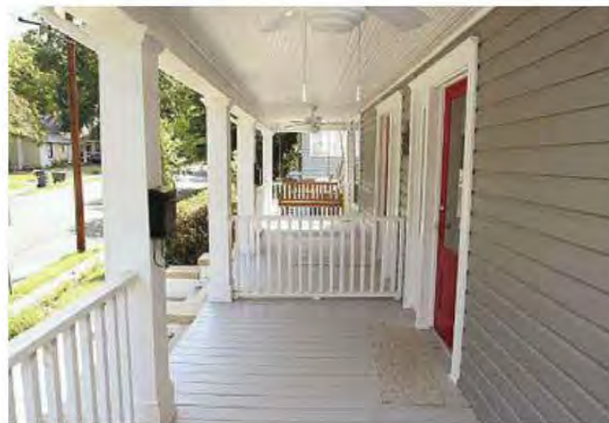
Fig. 8.27: A veranda is a roofed structure open to the exterior and structurally supported by columns.
