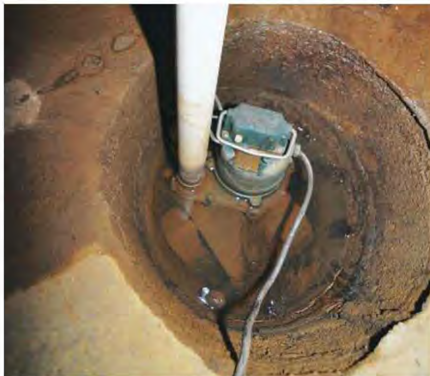
Fig. 9.13: A sump pump sits in a sump pit. Basements or crawl spaces are graded to direct water to this pit, where it is pumped to the exterior and away from the house.
