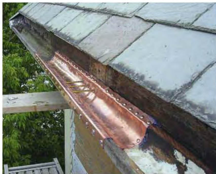
Fig. 8.21-22: Copper is molded to fit an original wood gutter form.
