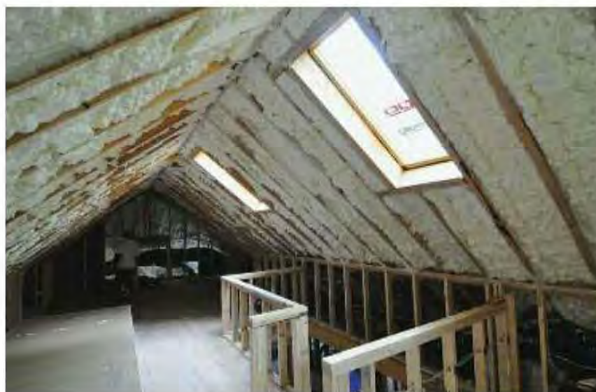
Fig. 7.21-23: Ceiling joists in the attic replaced with beefier floor joists. Rafters are sprayed with open cell foam in a sealed attic assembly. Skylights are placed on the north slope to let in light while restricting heat gain.
