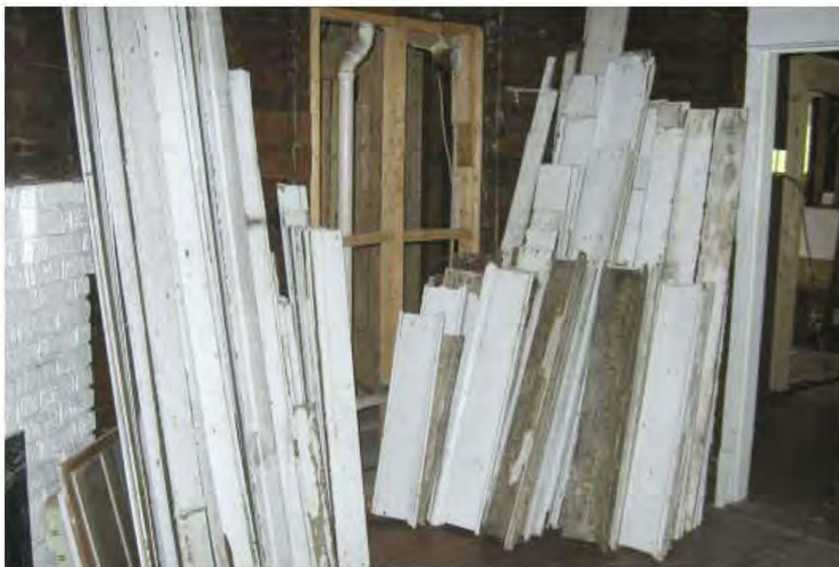
Fig. 6.25-26: If removed, trim should be carefully inventoried and stored for reuse.
