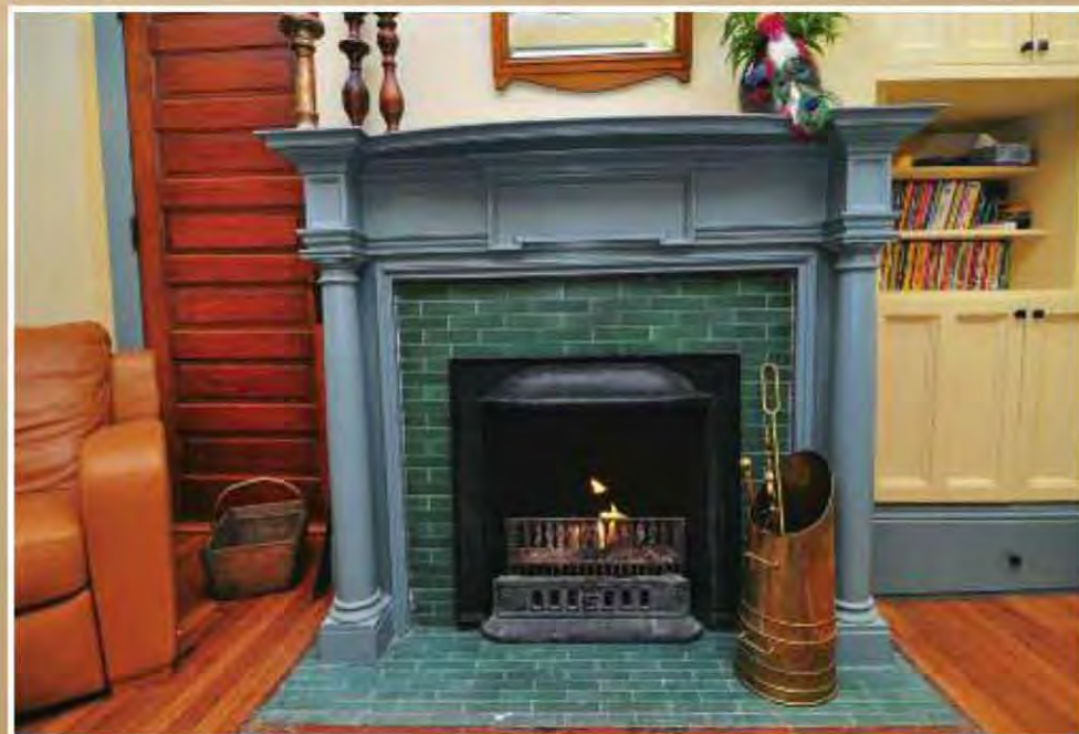
Fig. 6.9: The owners opened the cover and installed vented gas coal baskets, giving the appearance of coal burning. Vented chimneys vent harmful gases, making them preferred and superior to ventless alternatives.
