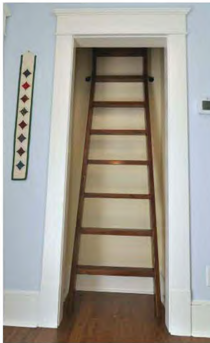
Fig. 7.4: Stairways may require too much space. Ladders can be used for access to an attic space, though they cannot be used for egress. Inspectors may require egress if the attic appears habitable.
