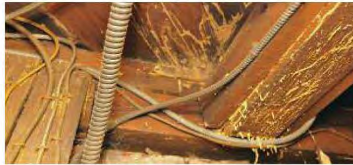
Fig. 9.21-22: Termites love a good, wet sill beam. Bottom, termites are attracted to beams saturated by water not from the ground, but from a leaky radiator. Inside, the girder, sillbeam and floorboards all show clear termite tunnels and stalactites.
