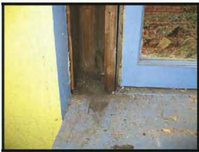
Fig. 11.26: Cranford House. Center, the counterweight cavity is opened, insulated, reinstalled and caulked airtight.
