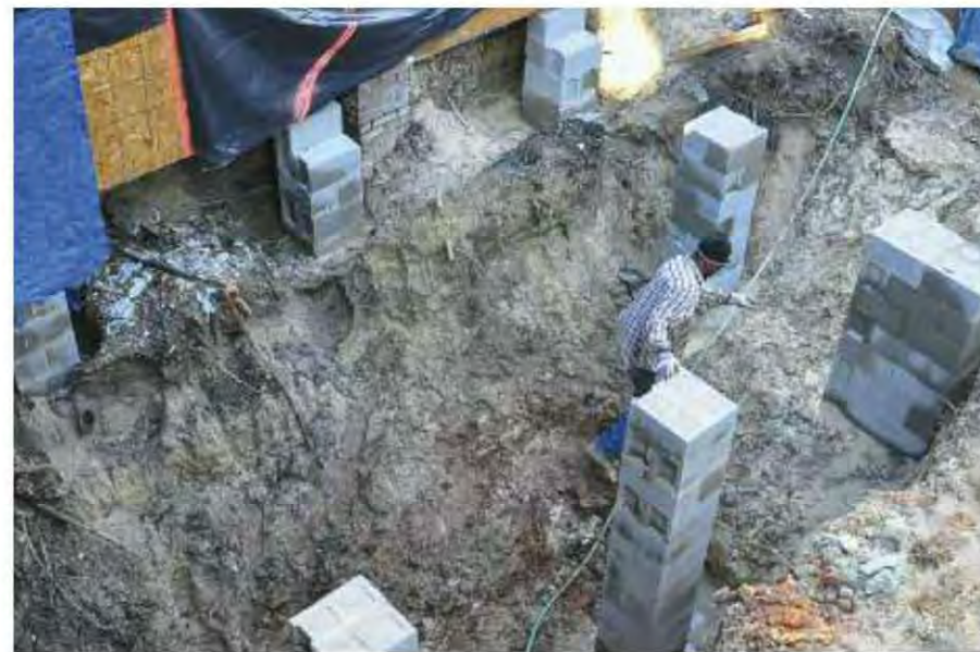
Fig. 9.4-6: Left, a new 24x24-inch footing is formed. Center, freestanding CMU block piers await framing for an addition to an historic home. Right, a continuous footing will support a load-bearing exterior wall.
