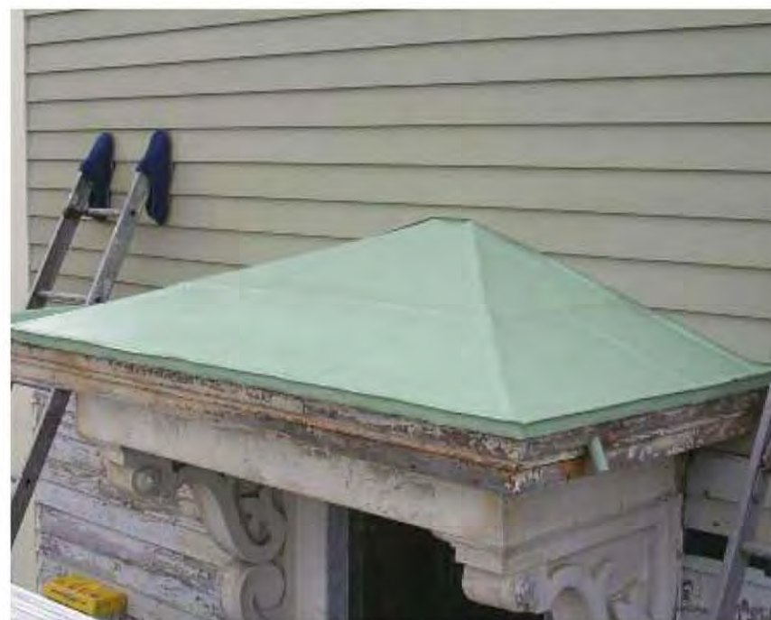
Fig. 8.14-17: Top left, roof decking is found to be in good shape. Top right, new felt and a copper standing seam roof is installed. Within a season copper will patina to a golden green. Bottom left and right, an entryway roof is redone.
