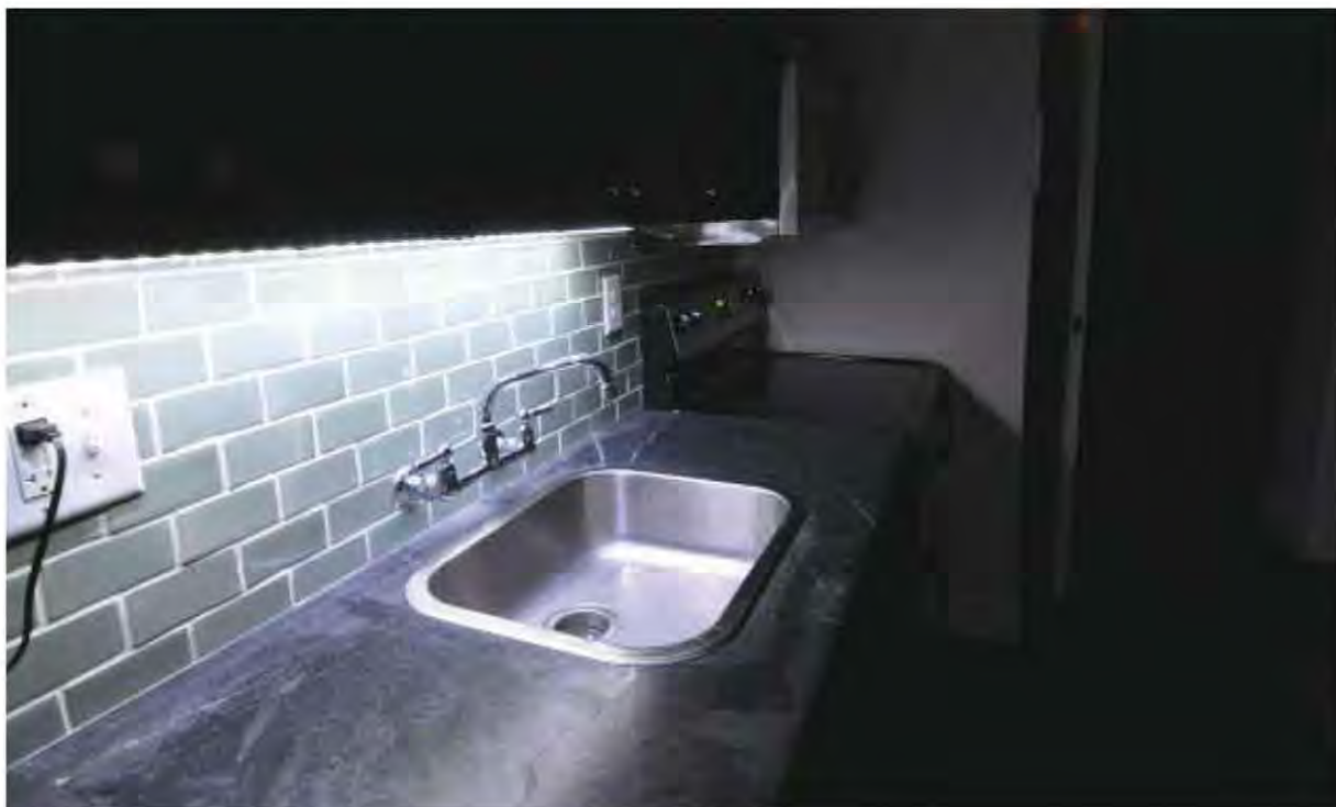
Fig. 5.8-9: Ambient LED under-cabinet lighting sets moods and softens the effect of harsher task lights.
