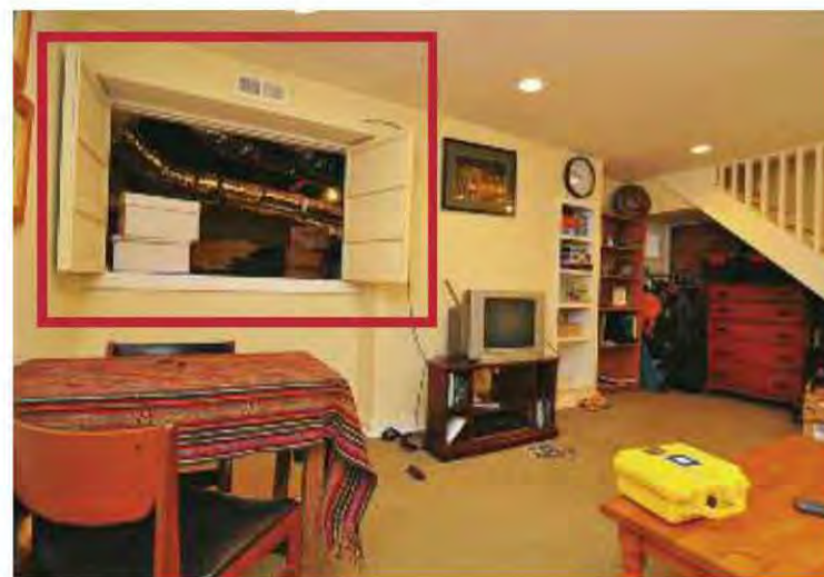
Fig. 10.12-14: Unlike a traditional crawl space, a sealed crawl space can be used for storage. Books, boxes and papers would nor- mally all be ruined by water in a tradi- tional crawl. Here, it's no different than putting them on a basement bookshelf. Bottom left, a close- up reveals the spray foam-insulated walls and polyethylene membrane on the floor.
