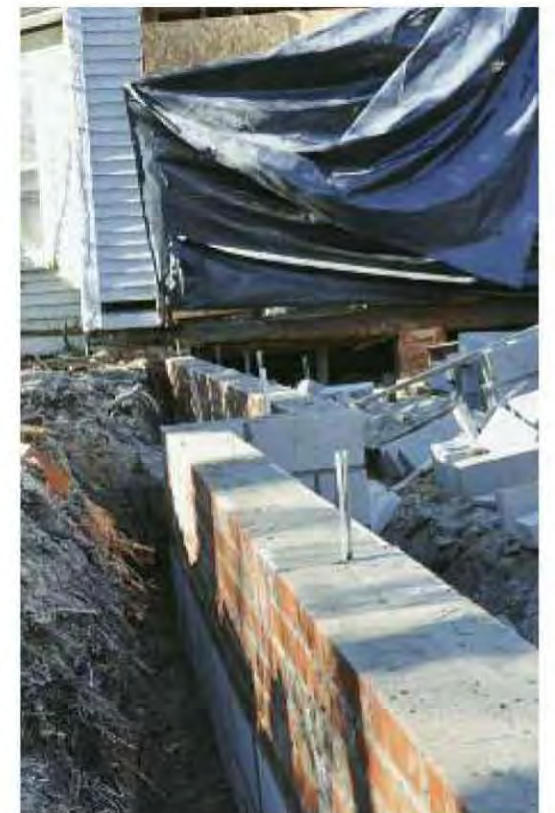
Fig. 9.4-6: Left, a new 24x24-inch footing is formed. Center, freestanding CMU block piers await framing for an addition to an historic home. Right, a continuous footing will support a load-bearing exterior wall.
