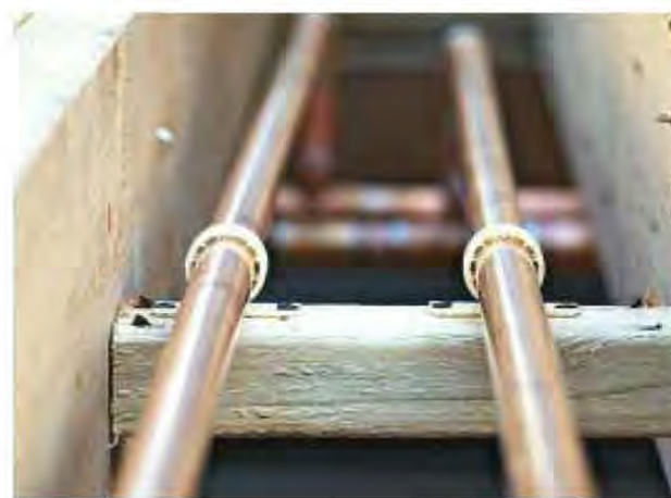
Fig. 12.2-3: Top, colored PEX with yellow gas line; bottom, copper.
