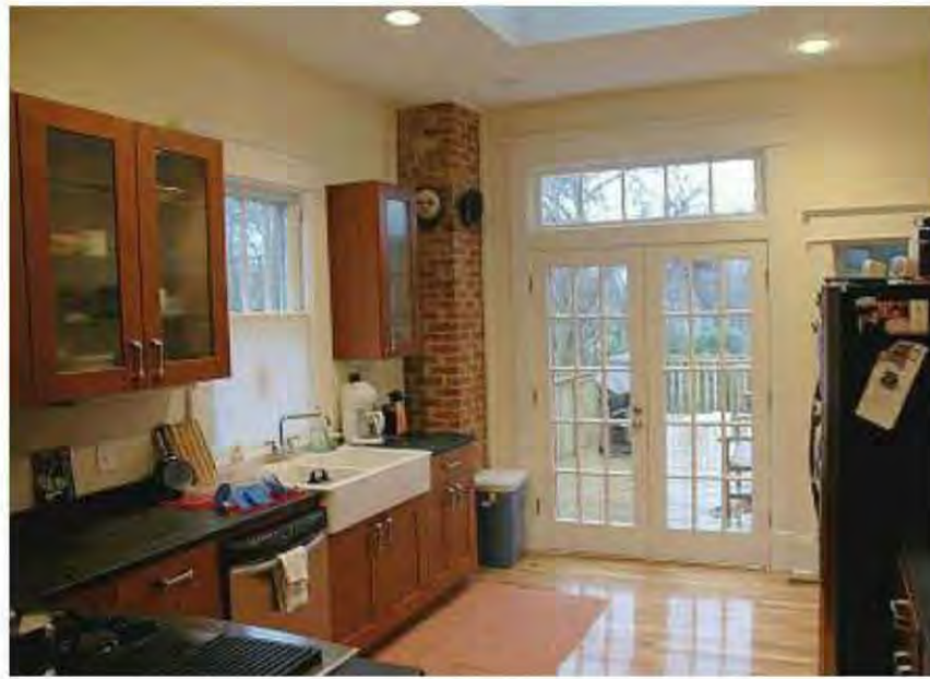
Fig. 5.30: A retired masonry chimney has been exposed, serving as a ghostmark of the home's previous systems and a nice architectural detail.
