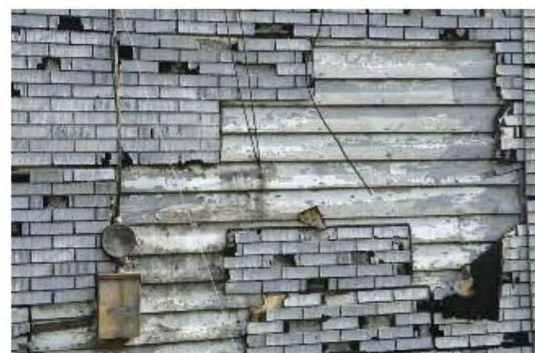
Fig. 8.6: A siding restoration reveals the damage vinyl siding installers do to original woodwork. The skirt board is destroyed, skirt sill detail deleted, window sills chopped and lintel detail deleted. Vinyl casing requires destruction of original woodwork. Artificial siding decreases door, window frame and cornerboard projections, eliminating shadow lines and creating a flat exterior. Good restorations aim to restore the craftsmanship.
