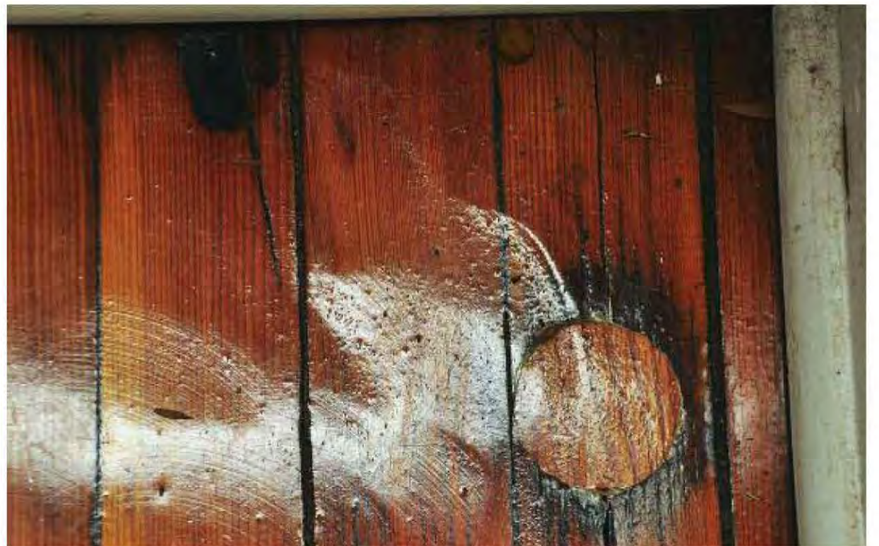
Fig. 13.19-21: Top, old radiators are sometimes kept in place as decoration, even after they are made nonfunctional. Center, a ghostmark wood patch indicates the placement of an old radiator pipe. Bottom, a new central system return claims a former closet, which is then uniquely turned into a nook for art display.
