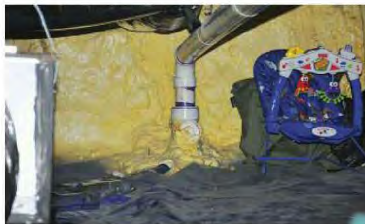
Fig. 10.12-14: Unlike a traditional crawl space, a sealed crawl space can be used for storage. Books, boxes and papers would nor- mally all be ruined by water in a tradi- tional crawl. Here, it's no different than putting them on a basement bookshelf. Bottom left, a close- up reveals the spray foam-insulated walls and polyethylene membrane on the floor.
