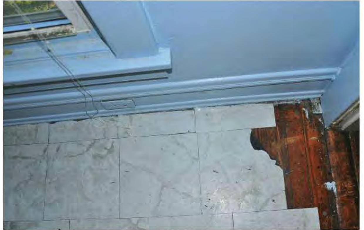
Fig. 6.17: A gorgeous wood floor lies under vinyl tile, the latter installed by someone who wrongly concluded the vinyl was easier to maintain than wood. As the photo shows, it was not.
