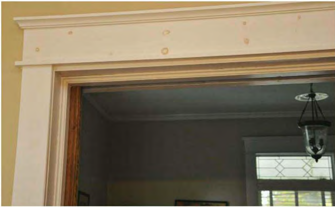
Fig. 6.21: Any interior trim should be select #1, clear and better grade wood free of knots with minimal imperfections. Knots will bleed through paint after a few years.
