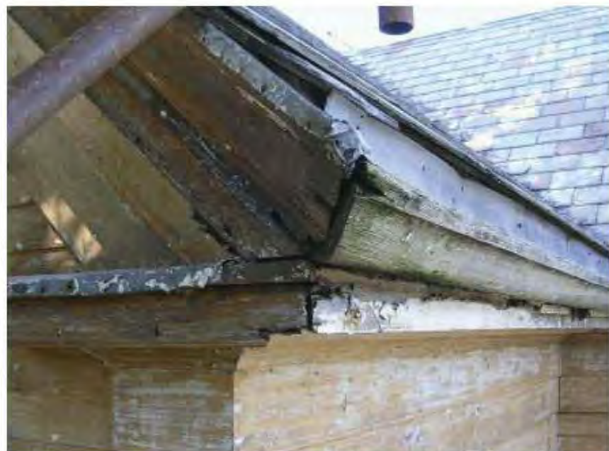
Fig. 8.10-12: A rotted return is repaired, flushed and painted.
