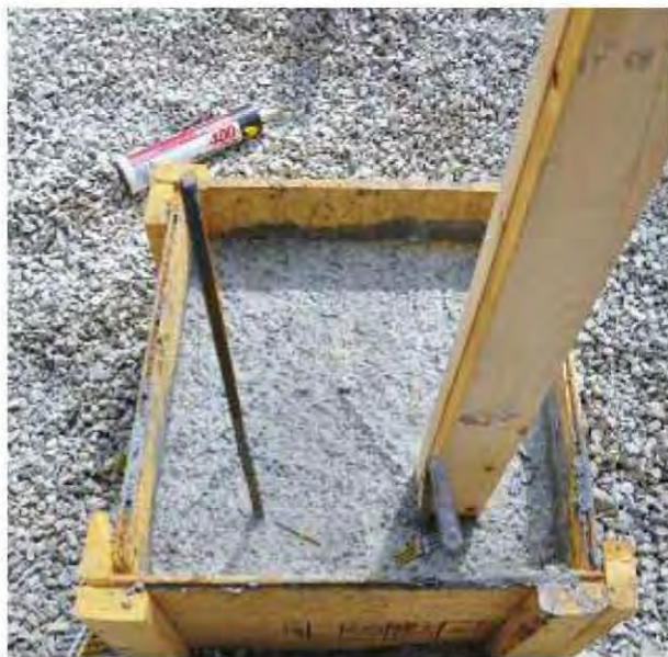
Fig. 9.4-6: Left, a new 24x24-inch footing is formed. Center, freestanding CMU block piers await framing for an addition to an historic home. Right, a continuous footing will support a load-bearing exterior wall.
