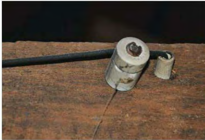
Fig. 14.20-22: Top, the porcelain knob and tube of the namesake wiring. Bottom left, a stud cavity has both knob and tube and BX armored cable. Bottom right, a gut job allows for easy rewiring with modern 14-2 Romex.
