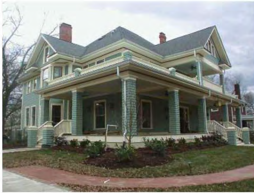
Fig. 11.24-25: Bussel House interior/ exterior. Top right, the addition of a non-descript 2 nd pane of glass to each individual sash is almost completely unnoticeable from either side of the window.
