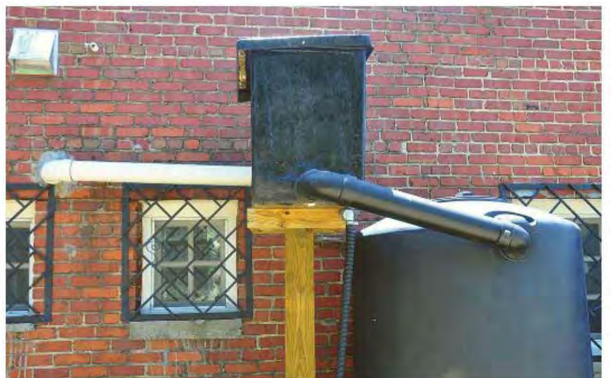
Fig. 12.15: A filter box catches debris before it enters the cistern.
