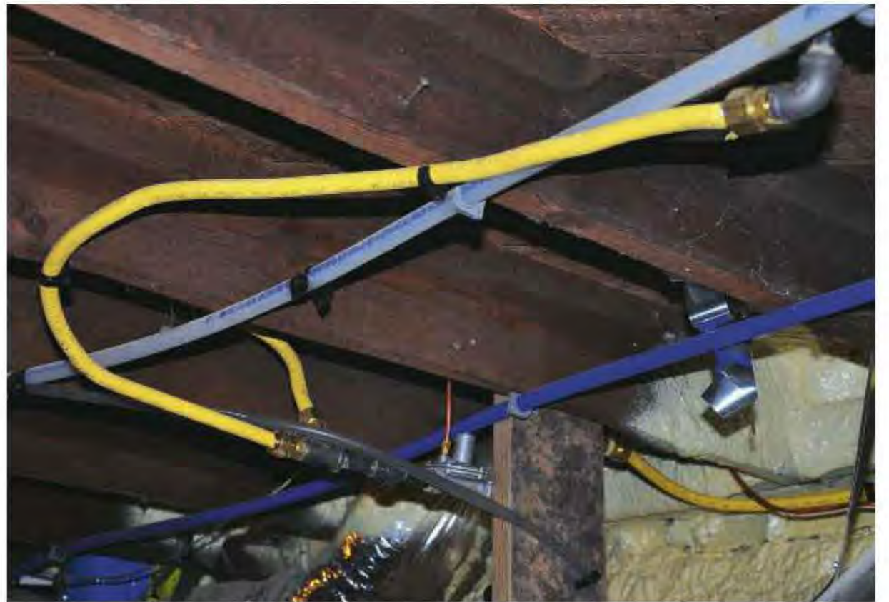
Fig. 12.2-3: Top, colored PEX with yellow gas line; bottom, copper.
