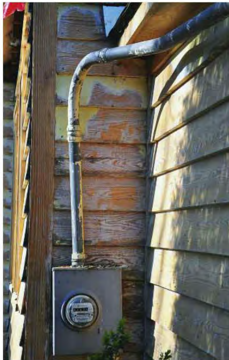
Fig. 14.2-3: Electricity comes to the home through an elevated weather-mast, through protective conduit to the meter and on to the circuitry panel. Generally speaking the homeowner is responsible for all maintenance beyond the meter, and the utility for everything on the other side.
