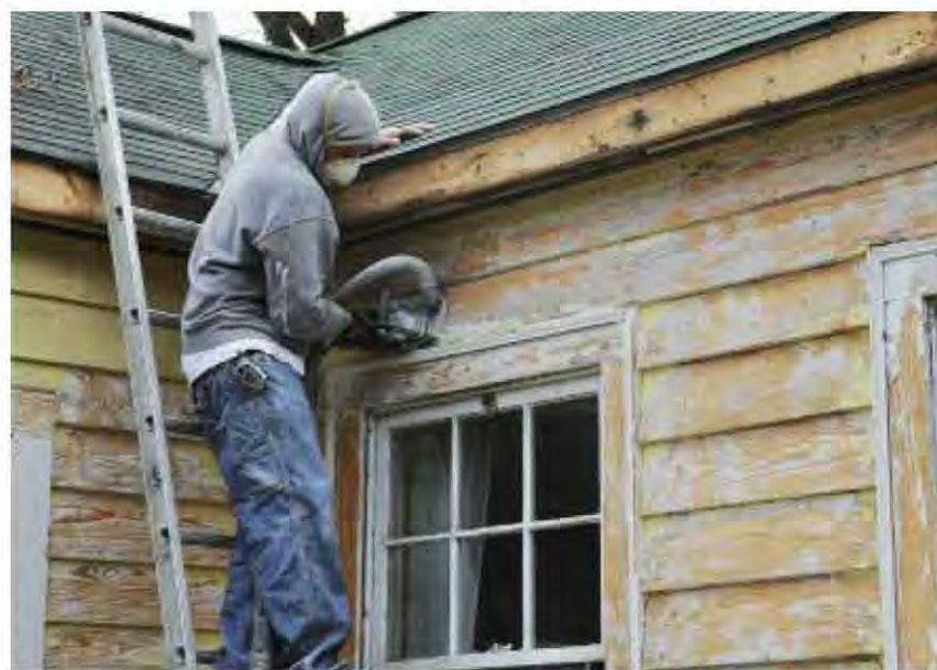
Fig. 8.37-38: Top, a simple test swabs a suspect area to detect lead. Within seconds, red means lead (pink too). Bottom, a paint shaver removes eight decades of paint in two passes, suctioning the debris into a HEPA-filter vacuum.
