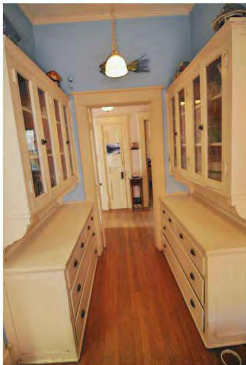
Fig. 5.31: A butler's pantry was once used for kitchen storage and food preparation. It features large original cabinetry, and a small eating nook. Such a room may risk being demolished for the sake of a larger kitchen.
