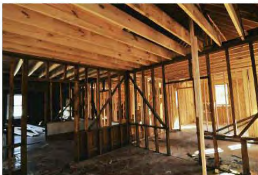
Fig. 7.21-23: Ceiling joists in the attic replaced with beefier floor joists. Rafters are sprayed with open cell foam in a sealed attic assembly. Skylights are placed on the north slope to let in light while restricting heat gain.
