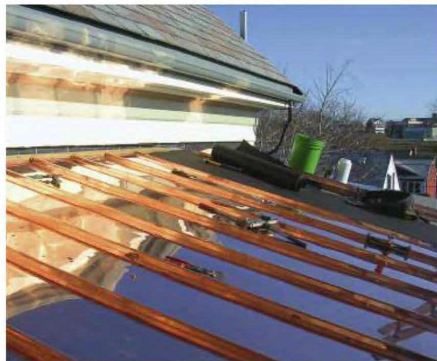
Fig. 8.14-17: Top left, roof decking is found to be in good shape. Top right, new felt and a copper standing seam roof is installed. Within a season copper will patina to a golden green. Bottom left and right, an entryway roof is redone.
