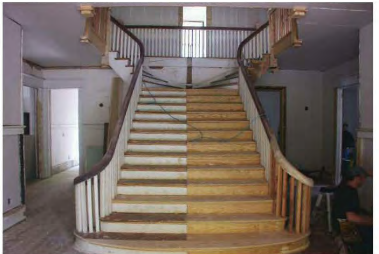
Fig 2.9-10: Center and bottom, a grand foyer staircase was split down the middle to partition a large home into two units. Exploratory demolition confirmed that the wall was not original, and suggested how to restore the original look.
