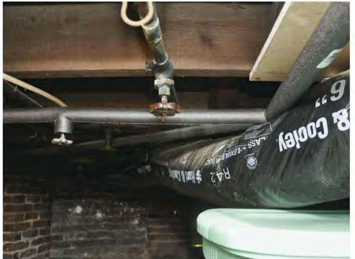
Fig. 12.20: Hot water pipe insulation is an inexpensive and simple upgrade.
