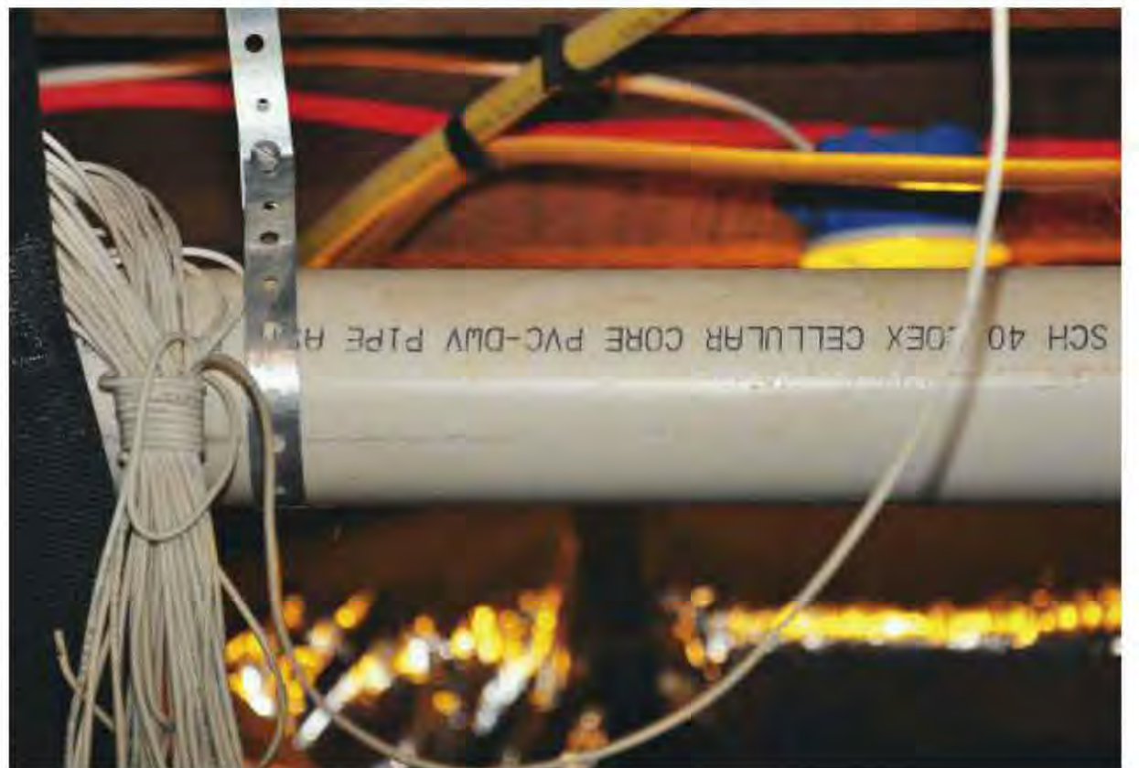
Fig. 12.5: PVC waste — the most commonly used residential pipe.
