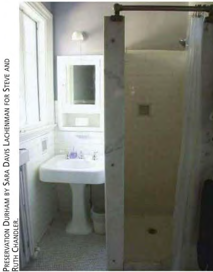
Fig. 4.1-2: A traditional restored bathroom features original double casement windows, hexagonal tile, pedestal sink, marble shower and a radiator. At right, a more modern aesthetic.
