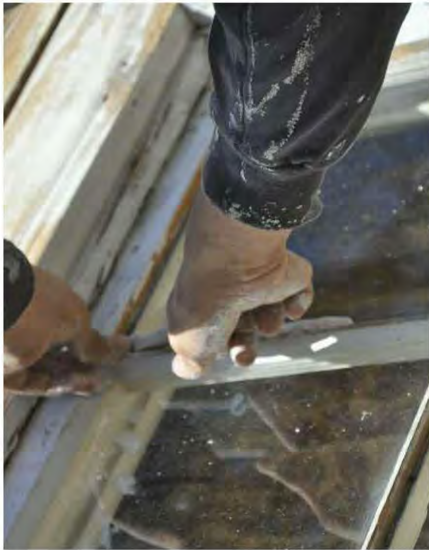
Fig. 11.18-19: When exterior window glazing falls into disrepair, reglazing is required. The old glazing is removed, the new glazing installed and a doughy putty is applied and cut at an angle to minimize the profile. Glazing is being installed at left, and new glazing is completed at right.
