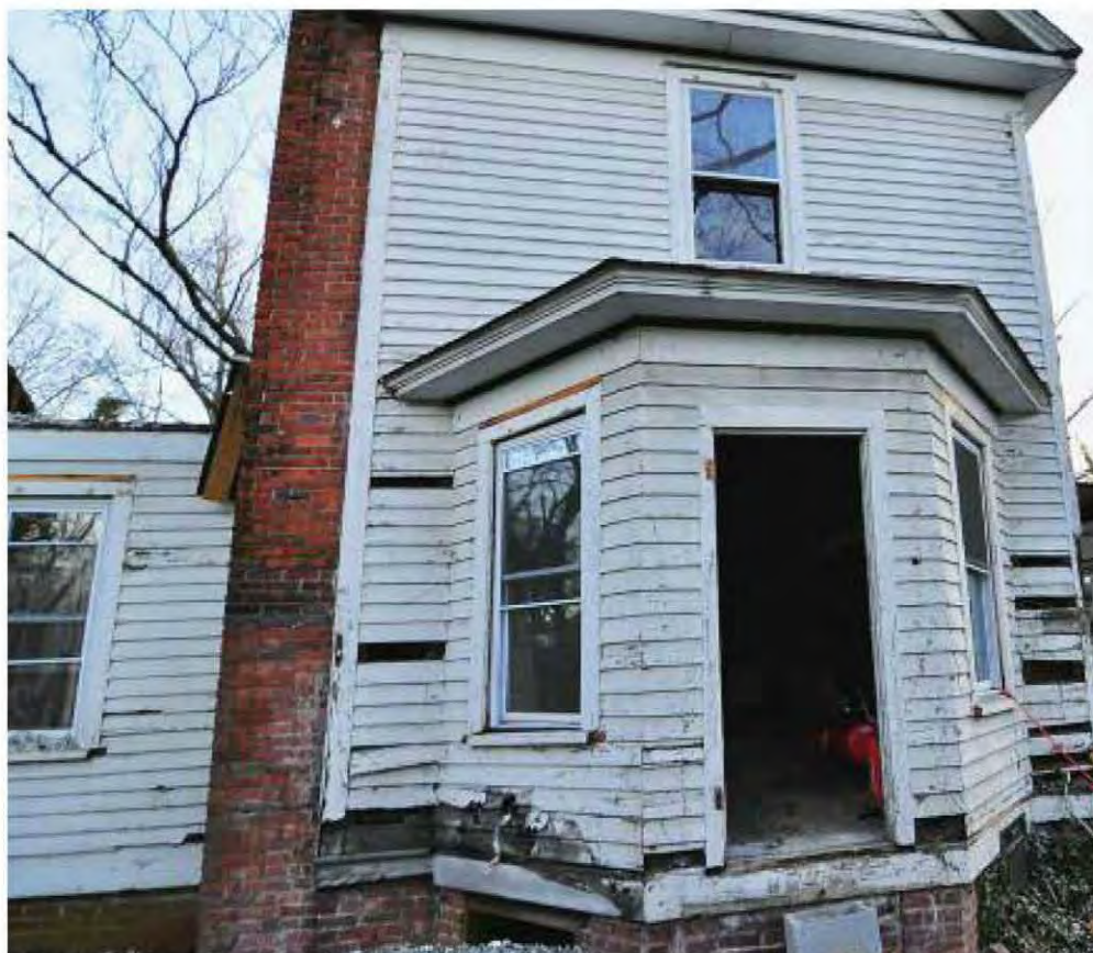
Fig. 8.6: A siding restoration reveals the damage vinyl siding installers do to original woodwork. The skirt board is destroyed, skirt sill detail deleted, window sills chopped and lintel detail deleted. Vinyl casing requires destruction of original woodwork. Artificial siding decreases door, window frame and cornerboard projections, eliminating shadow lines and creating a flat exterior. Good restorations aim to restore the craftsmanship.
