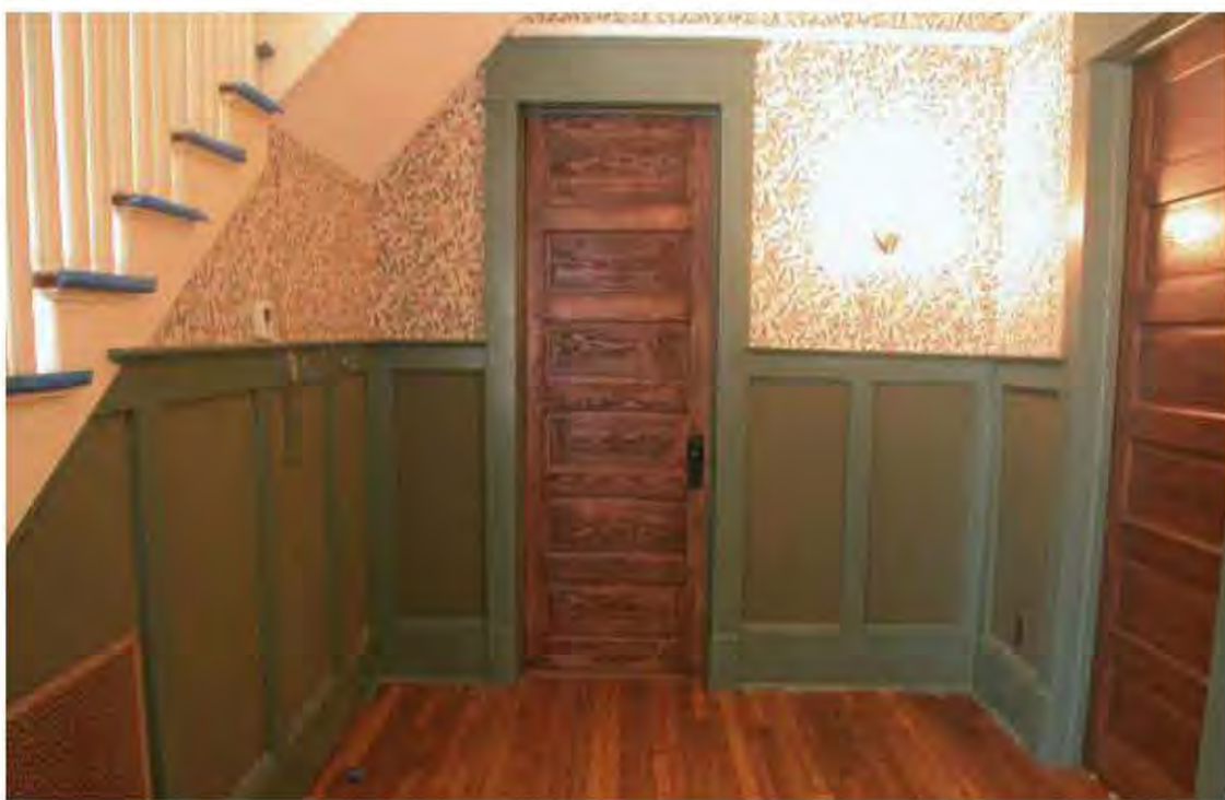
Fig. 6.20: The casing on this historic home requires 16 pieces, made from five different moldings: 5/4 plinth, 1x6 casing, 1x2 lintel base, 1x8 lintel and lintel crown. Old trim is grand in size and detail, while modern trim lacks an emphasis on quality, revealed by its nickname, speedbase.
