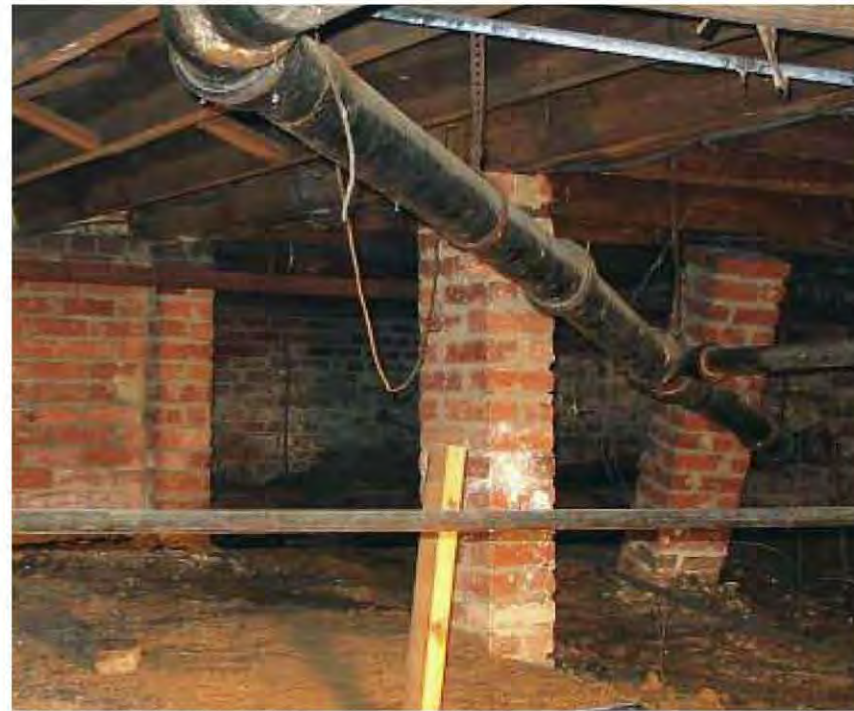
Fig. 9.2-3: Top, a pier and curtain wall. The piers bear the weight, and the curtain is not load-bearing, though in practice this house has settled and does bear on the curtain wall. Bottom, two freestanding piers bear interior girders; the pier in the background has failed and must be reconstructed.
