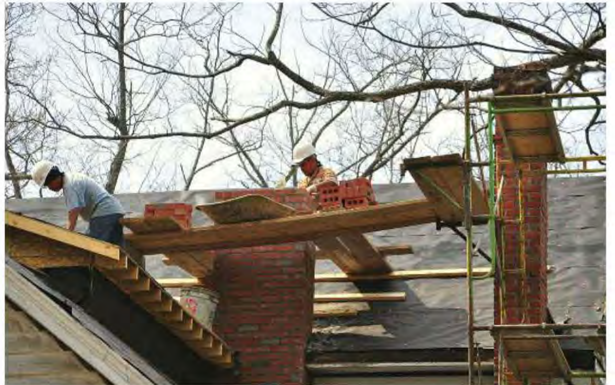
Fig. 8.24: A chimney being reconstructed.
