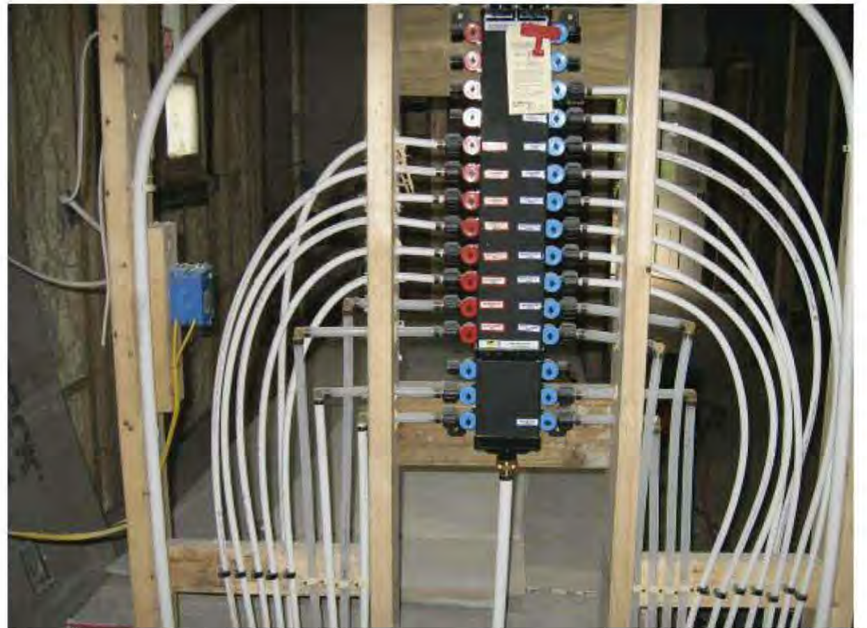
Fig. 12.21: A manifold plumbing system — \frac{3}{8} -inch supply lines mean hot water gets there faster.
