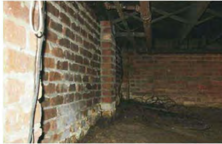
Fig. 9.2-3: Top, a pier and curtain wall. The piers bear the weight, and the curtain is not load-bearing, though in practice this house has settled and does bear on the curtain wall. Bottom, two freestanding piers bear interior girders; the pier in the background has failed and must be reconstructed.
