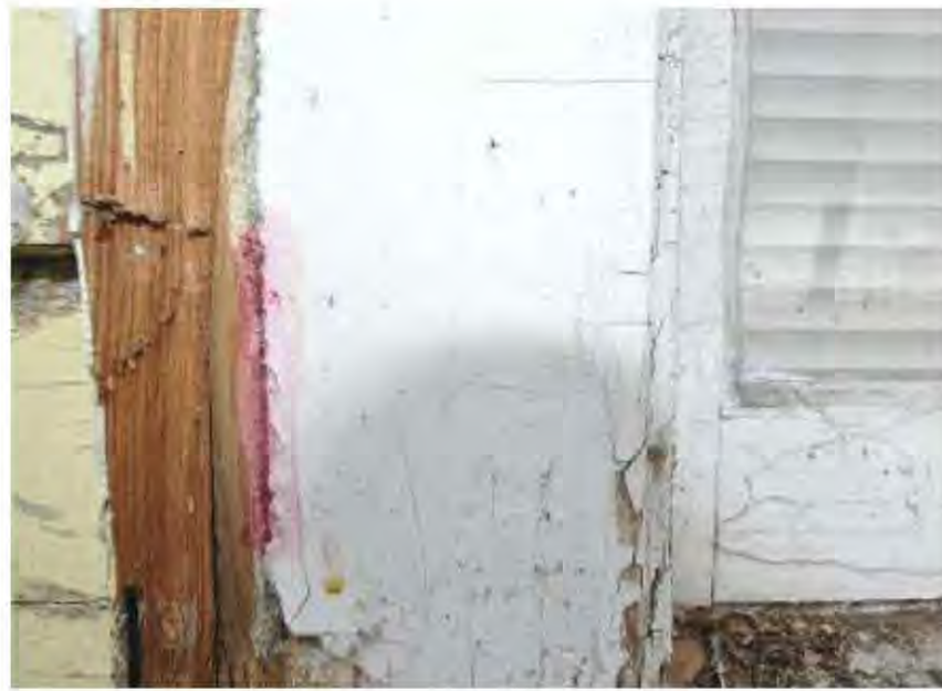
Fig. 8.37-38: Top, a simple test swabs a suspect area to detect lead. Within seconds, red means lead (pink too). Bottom, a paint shaver removes eight decades of paint in two passes, suctioning the debris into a HEPA-filter vacuum.
