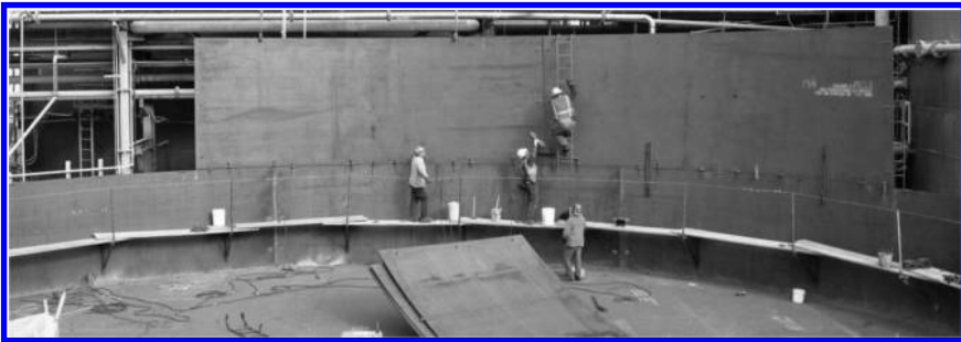
Erection of second shell course in progress.
