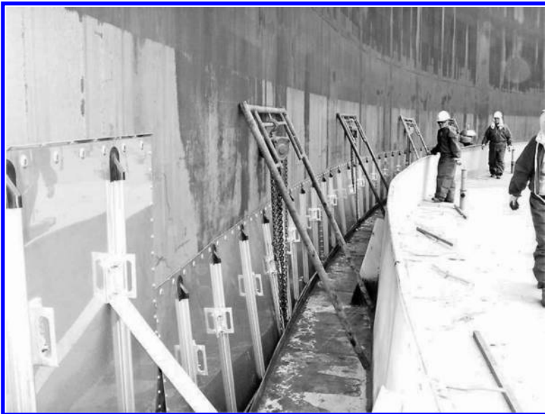
Shoe plate attachment works.
