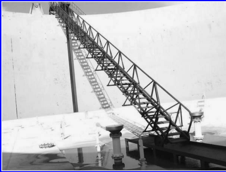
Rolling ladder and antirotation device.
