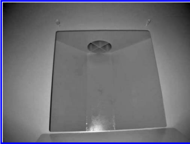
Tank bottom sump.
