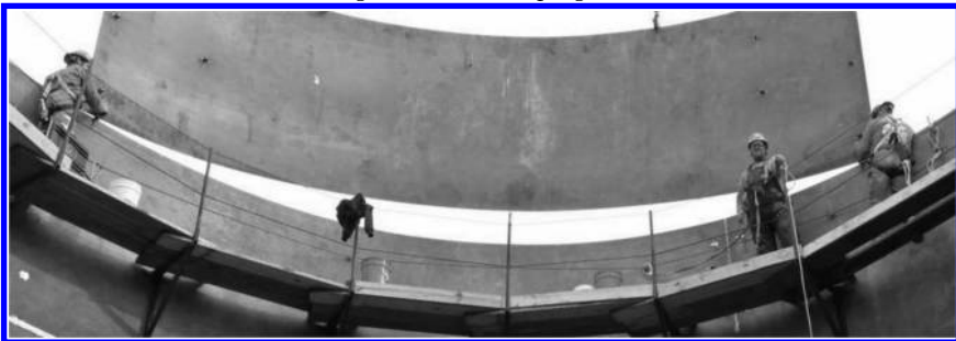
Erection of shell at higher elevation in progress (view from inside).
