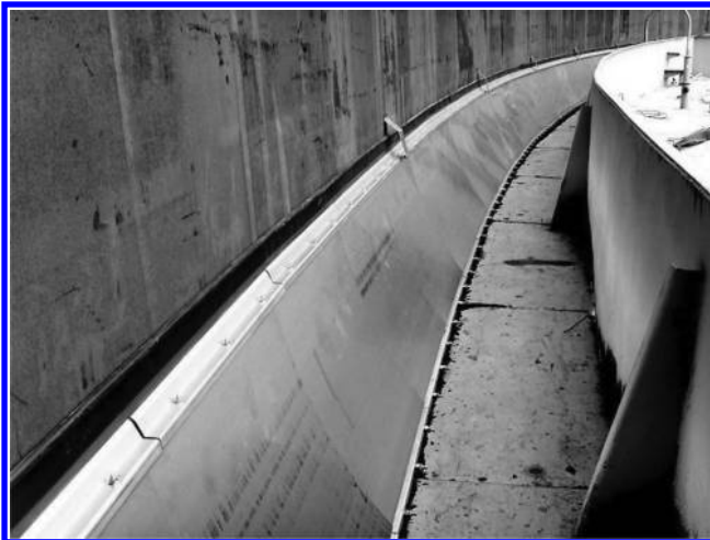
Secondary seal system.
