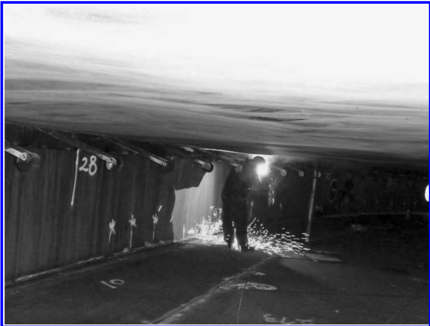
Installation works of shoe arm and counterweight arm.
