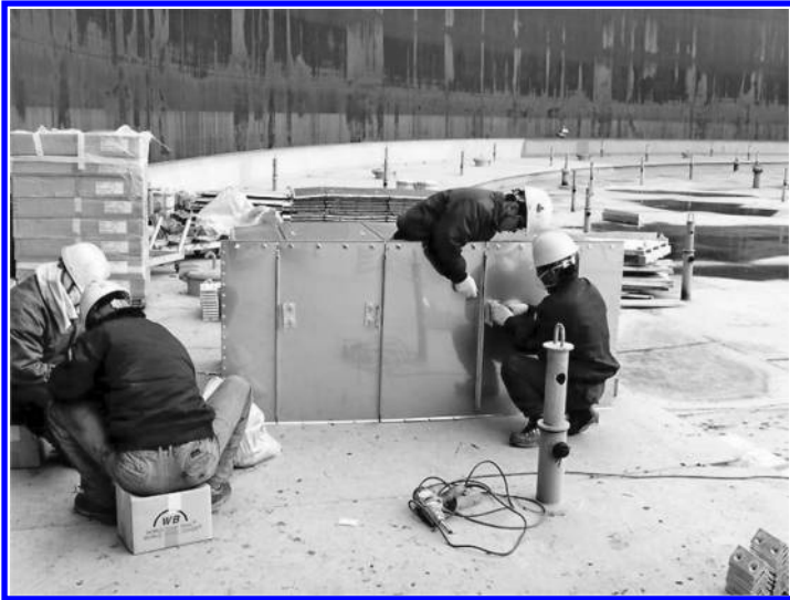
Preparation works for attaching shoe plate.
