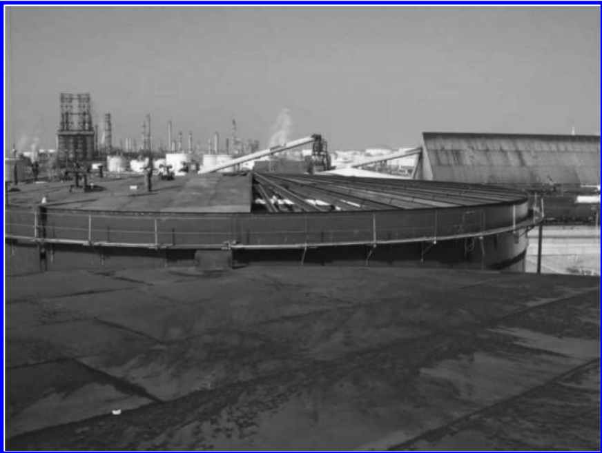
Supported roof partially completed.
