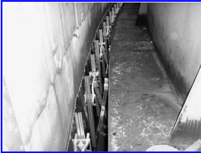
Installed shoe arm and counterweight arm.
