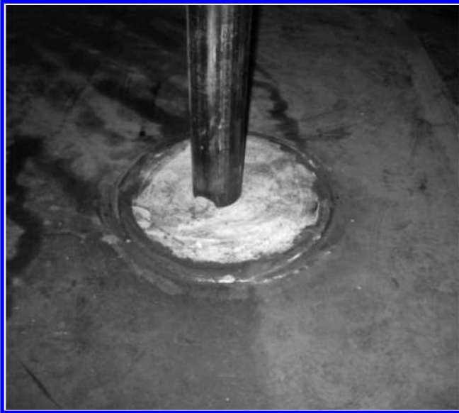
Reinforcing pad for roof leg.
