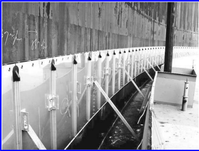
Shoe plates after installation.
