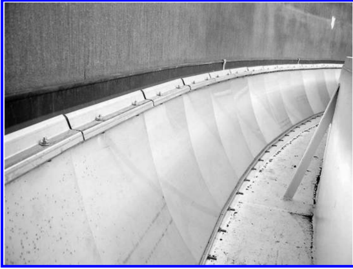
Pantograph-type mechanical shoe seal.
