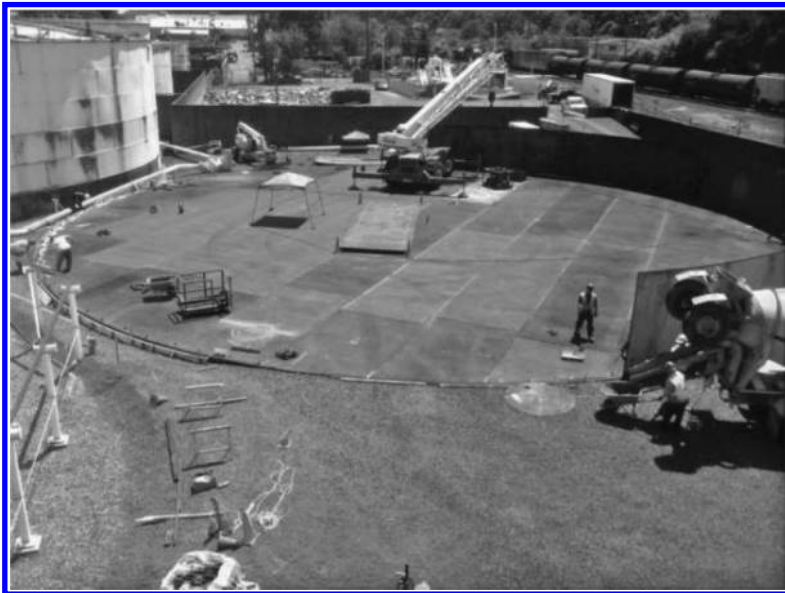
Erection of first shell course in progress.
