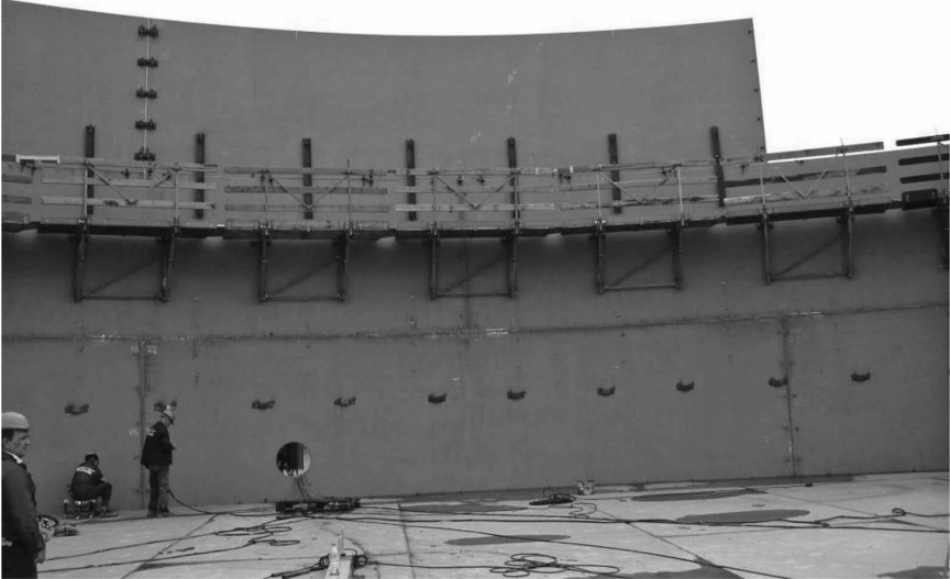
Third shell course erection in progress (view from inside).
