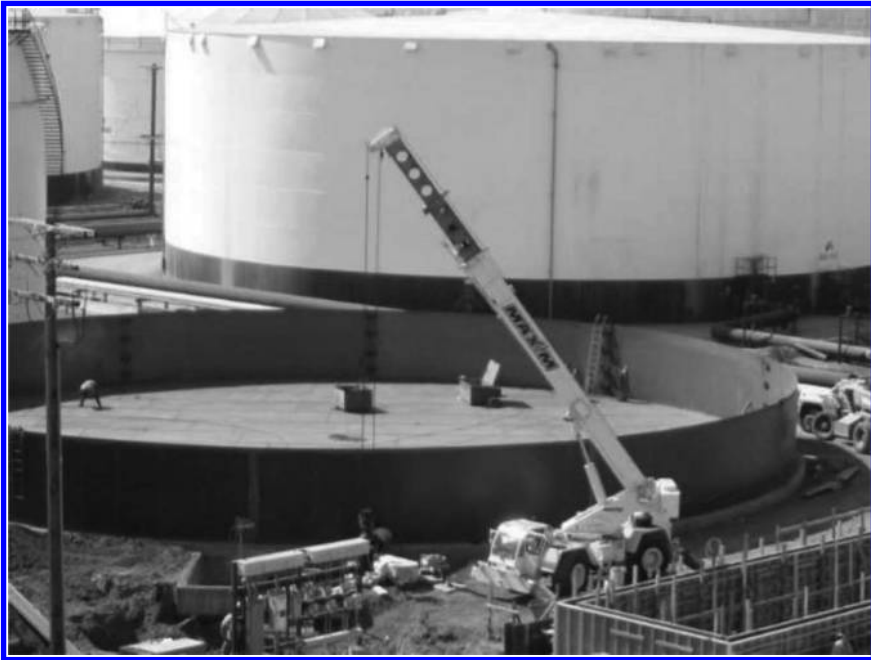
Erection of first shell course in progress (nearly complete).
