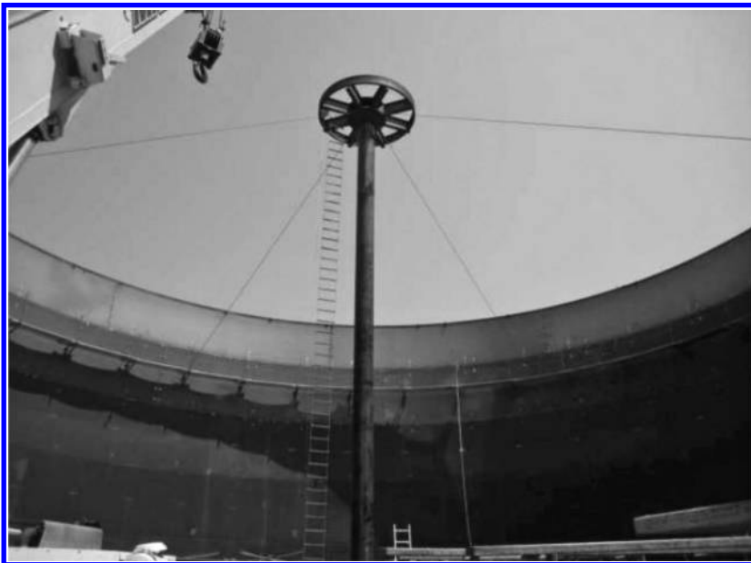
Roof construction: bull wheel and center column in progress.
