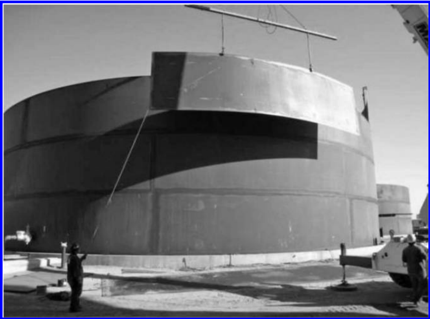
Fourth shell course erection in progress (view from outside).
