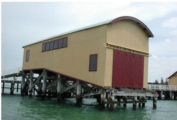
Fig. 7.4 Queenscliff new pier lifeboat shed
