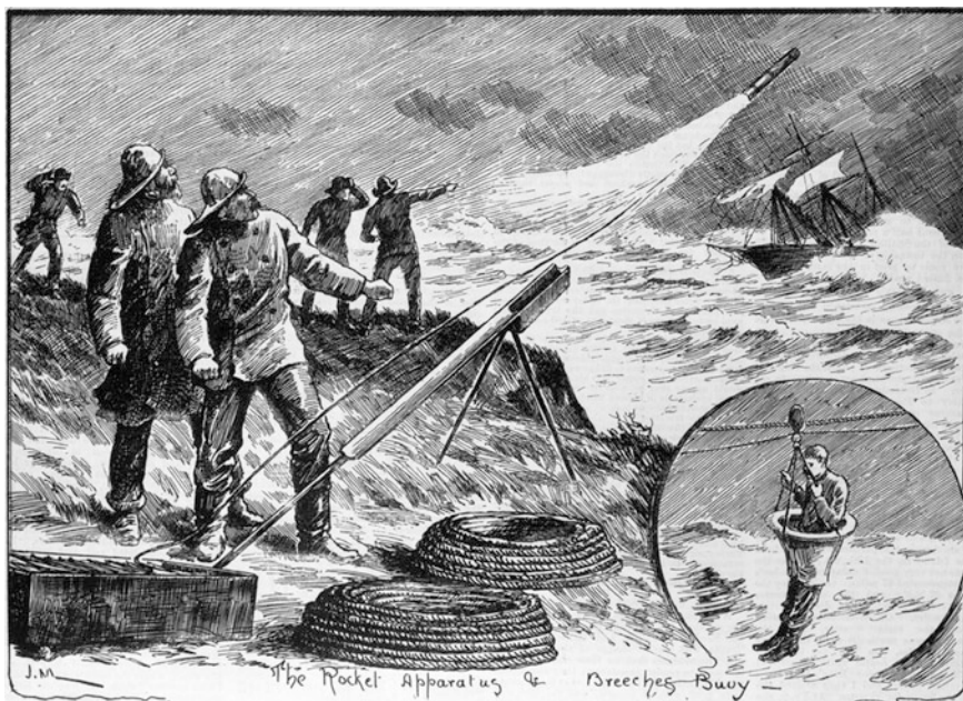
Fig. 4.5 Deploying a breaches buoy lifeline via a lifesaving rocket at Pt Nepean (Image Macfarlane 1892, SLV Collection)
