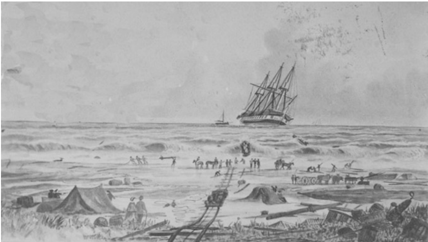
Fig. 5.4 Salvors at work on Sussex . Note the use of tramway and corduroy road to the wreck (Image after Roberts & Co 1872, SLV collection)
