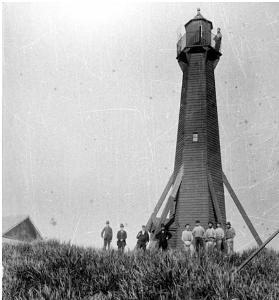
Fig. 6.3 Pt Lonsdale timber light tower c. 1867, previously located at Shortlands Bluff ( Photograph PH4560, C. Nettleton, QHM collection)
