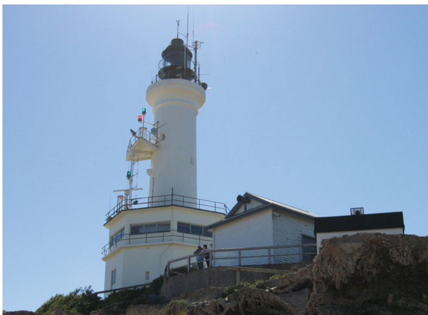
Fig. 6.6 Pt Lonsdale Lighthouse and lookout station, fog horn shed and scend shed
