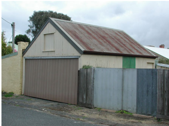
Fig. 7.17 Former morgue in Andrews St, Queenscliff
