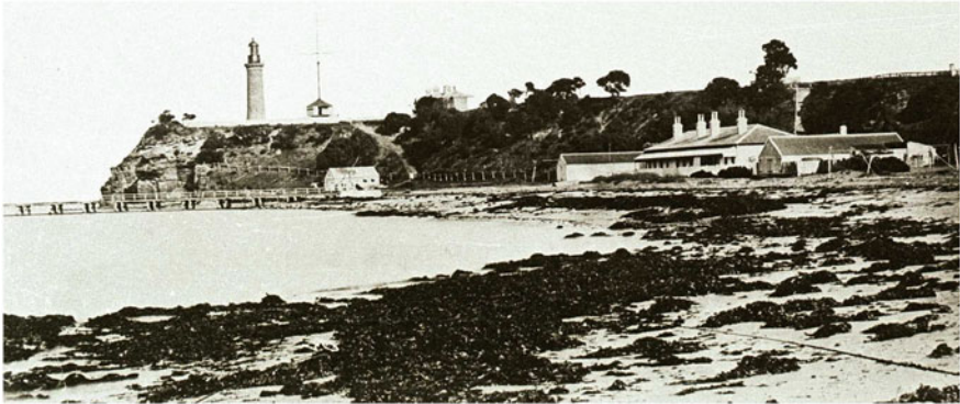
Fig. 3.9 Pilots Reserve buildings and Pier c.1882 ( Photograph PH24 Queenscliff Historical Society)
