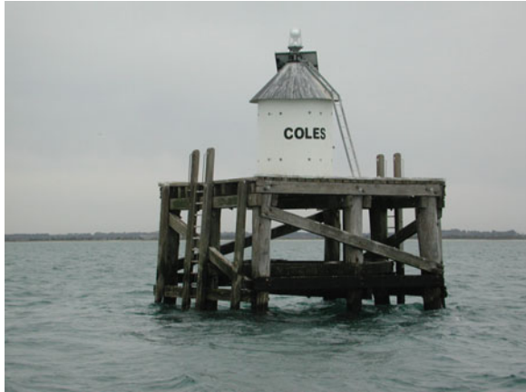
Fig. 6.15 Unmanned pile light—Coles Channel Pile Light beacon (also known as White Lady)
