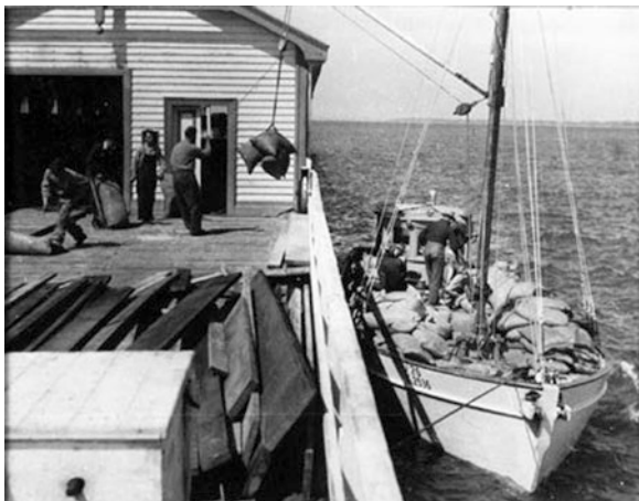
Fig. 5.2 Unloading sugar from the Time shipwreck (Photograph PH3440, QHM collection)
