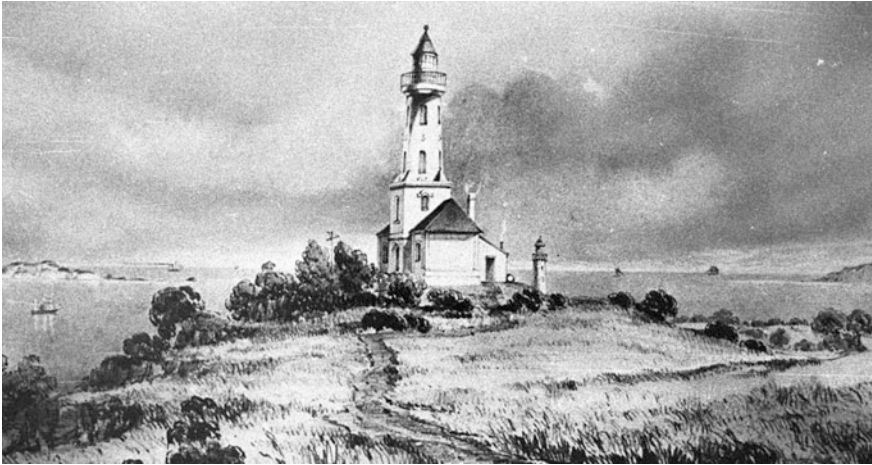
Fig. 6.1 Original Shortlands Bluff Lighthouse in 1857. Note the Shortlands Bluff Low Light Timber Tower to the right (Image PH1, QHM Collection)
