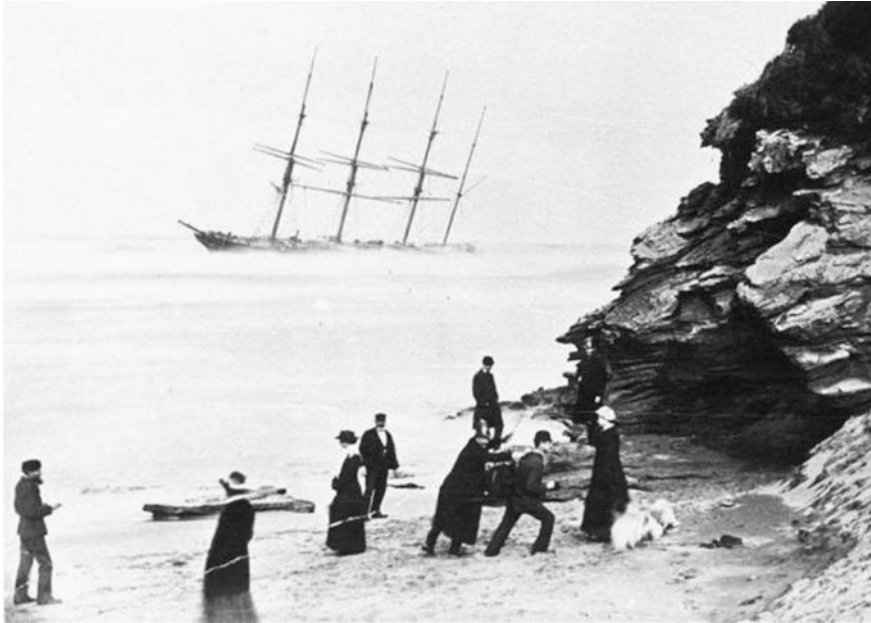
Fig. 4.9 Wreck of George Roper (1883). Note the policeman beating a looter in the foreground (Photograph PH2801, QHM Collection)
