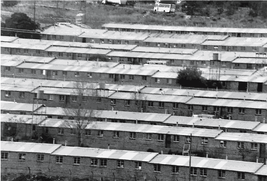
Photo 8.3. Hostel for seasonal workers in Soweto (Source: Jürgens).
