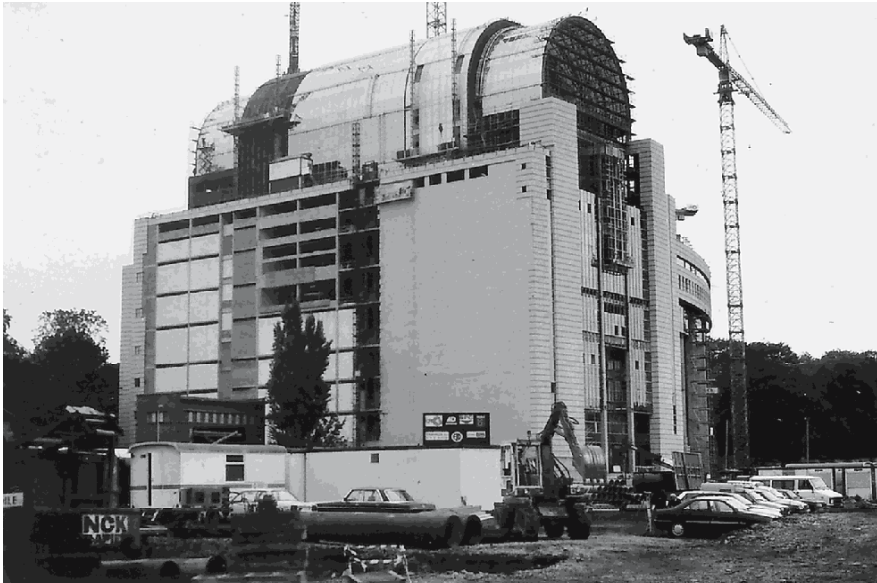
Photo 10.3 Centre Internationale du Congrès with dome-shaped roof of its parliament-like hall
