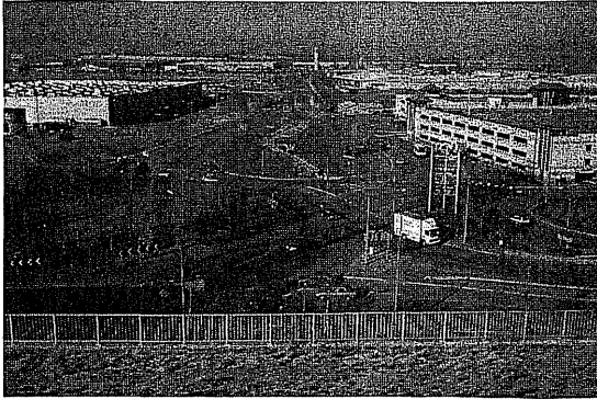
3 Building in a quarry displays the worst features of the landscape and architecture (Lakeside, Thurrock, east of London).
