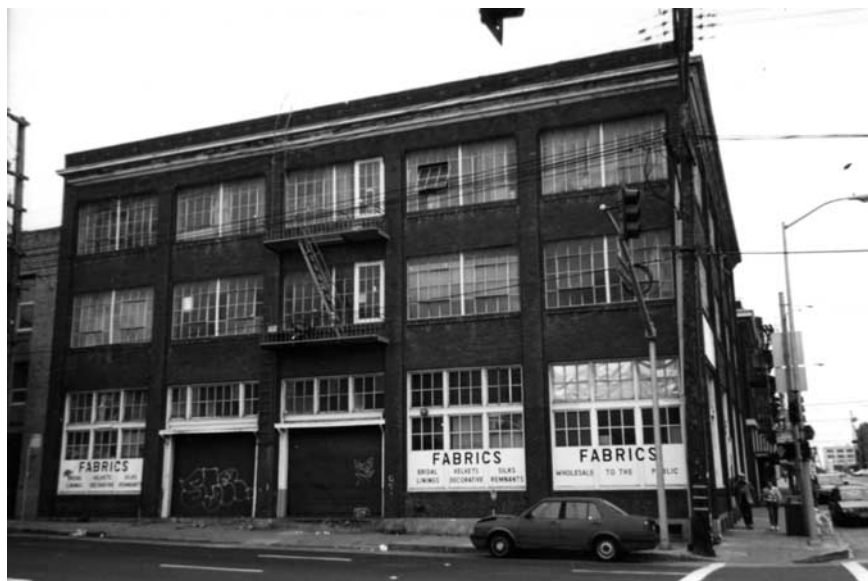
Figure 7.9 Fabric clearance store, circa 2001, Third and Bryant Streets (now a digital art gallery).
