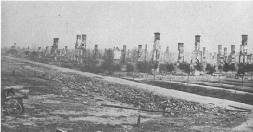
Figure 5.11. Photo of Gävle after the fire of 1869. Great fires were recurrent events in the history of Swedish towns, and an important prerequisite of the regulation plans. Source: Gävle kommuns centralarkiv, Gävle.
