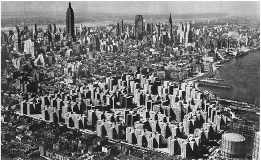
2.11. This view of the completed project, from the southeast, demonstrates the unprecedented innovation of Met Life’s intervention in the old cityscape and the immensity of the project in comparison with the city around it. By Thomas Airviews, in the Collection of the New-York Historical Society.
