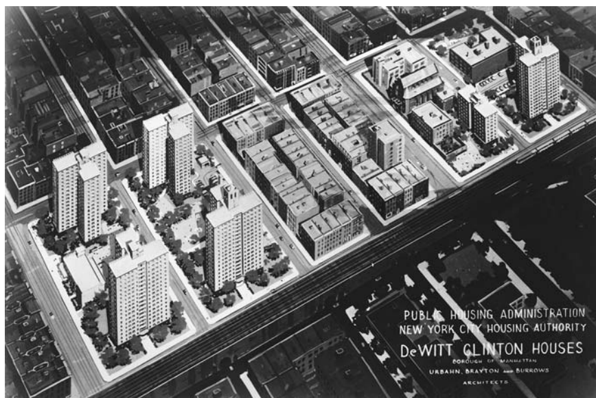
7.8. DeWitt Clinton Houses as it was eventually constructed on two separate slivers of available land. (The two blocks at left and the two towers at upper right make up the project.) One of the authority's first vest-pocket projects, it respected the street grid but still looked to supply light and air to residents with tower-in-the-park designs. New York World-Telegram Photograph Collection, Library of Congress.
