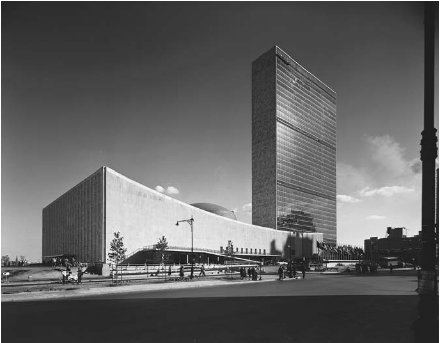
1.3. The General Assembly Hall and Secretariat from the northwest. Ezra Stoller specialized in capturing the clean lines and austere shapes of modern architecture. His photos, which frame buildings as works of art, give the viewer a good sense of the way that modern structures like the Secretariat and General Assembly Hall were understood by both their creators and the public as symbols of newness, freed from all historic and spatial context. Ezra Stoller © Esto.
