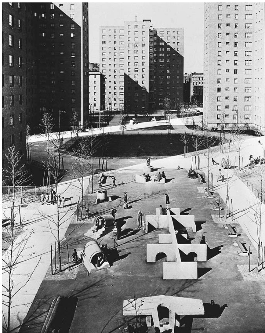
6.4. The James Weldon Johnson Houses in East Harlem during the 1950s. When they went up in the late 1940s, the Johnson Houses were a prime example of NYCHA's traditional red-brick modernism and laid out in the cruciform shape the authority had been using since the 1930s. Only a few years later, these designs would be phased out for more advanced variations on the slab form, which offered less ground coverage and greater cost savings. New York City Housing Authority Records, La Guardia and Wagner Archives.
