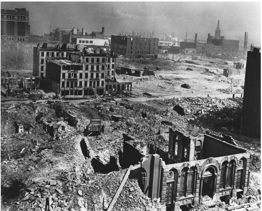
2.8. The remains of the Gas House District during clearance for Stuyvesant Town in 1945. Observers often likened clearance sites to images they had seen of bombed cities during World War II, which had ended only months earlier. New York World-Telegram Photograph Collection, Library of Congress.
