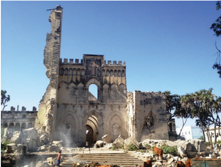
Fig. 6.3 Remnants of a church in Mogadishu. Photograph taken by M.I., 2011
