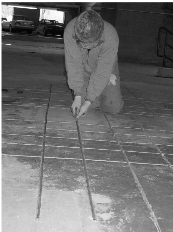
Figure 1.9 Installation of near-surface-mounted (NSM) strips. (Courtesy of Structural Group.)
