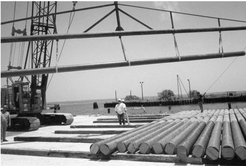
Figure 1.7 FRP piles. (Courtesy of Lancaster Composites.)
