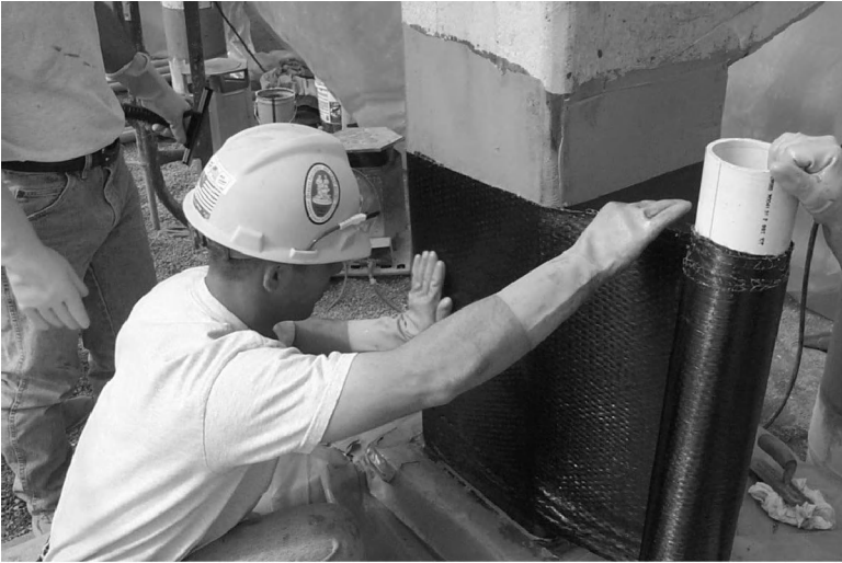
Figure 1.11 Installation of FRP wrap. (Courtesy of Sika Corporation.)
