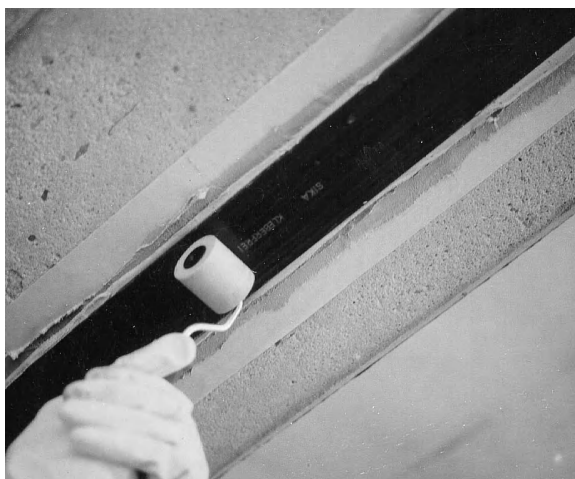
Figure 1.8 Installation of a precured FRP strip. (Courtesy of Sika Corporation.)
