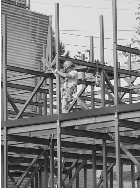
Figure 15.3 Stick-built light-frame pultruded structure. (Courtesy of Strongwell.)
