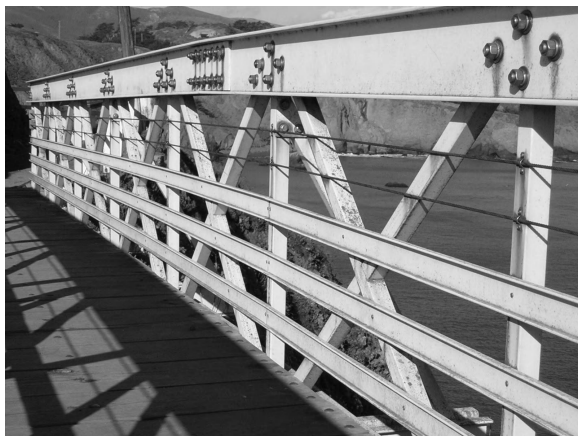
Figure 15.2 Connection details on the Point Bonita bridge.
