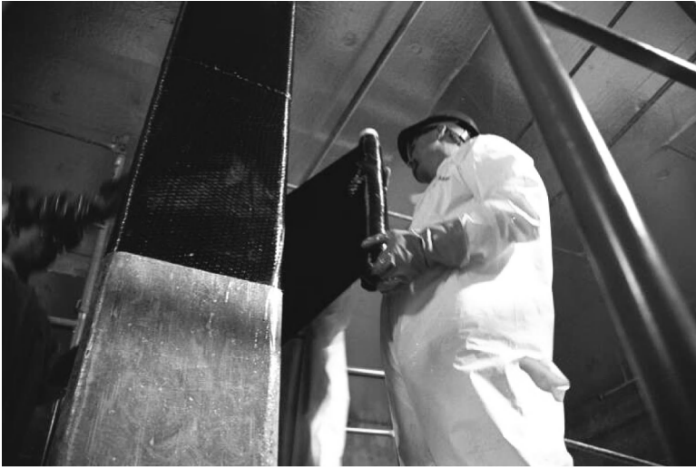
Figure 11.2 FRP wrapping of a rectangular column. (Courtesy of Structural Group.)
