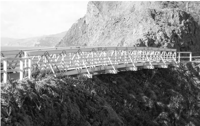
Figure 15.1 FRP bridge at Point Bonita, California.
