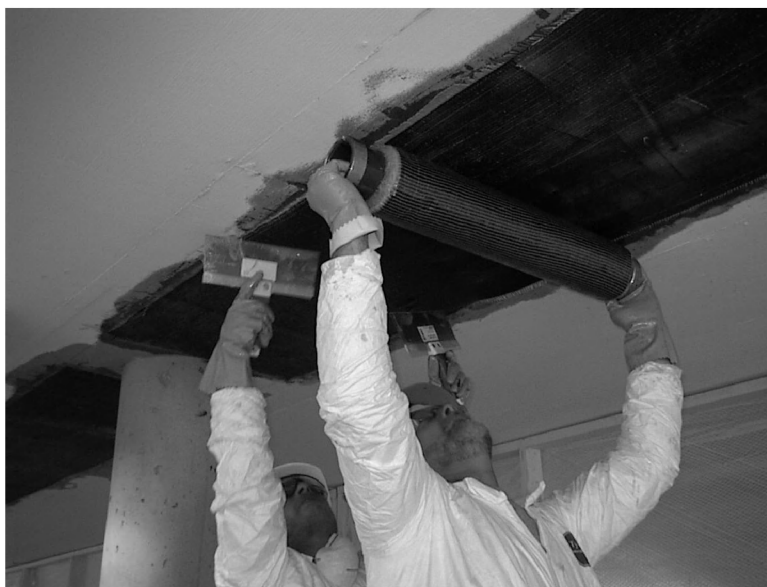
Figure 1.10 Installation of a carbon fiber fabric sheet. (Courtesy of Fyfe Company.)
