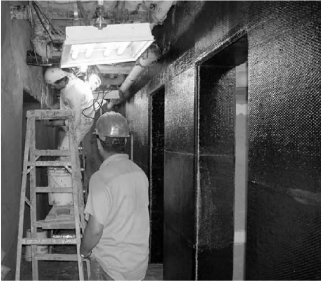
Figure 1.13 FRP fabrics for building shear wall retrofit. (Courtesy of Racquel Hagen.)
