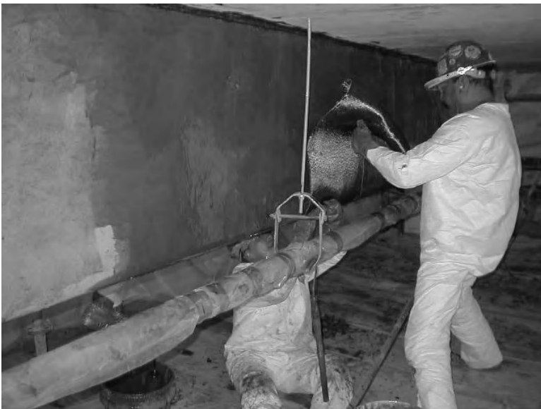
Figure 10.1 FRP Shear strengthening of a beam. (Courtesy of Structural Group.)
