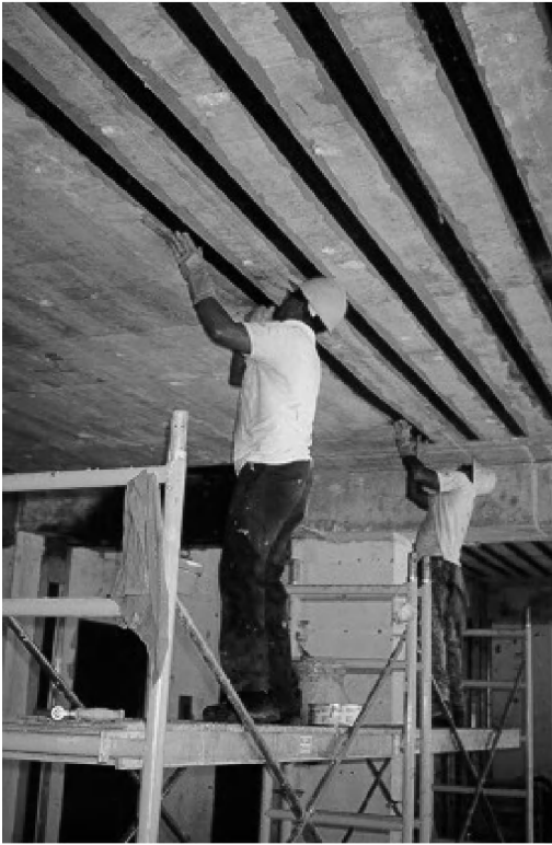
Figure 9.2 Flexural strengthening of a reinforced concrete slab. (Courtesy of Sika Corporation.)
