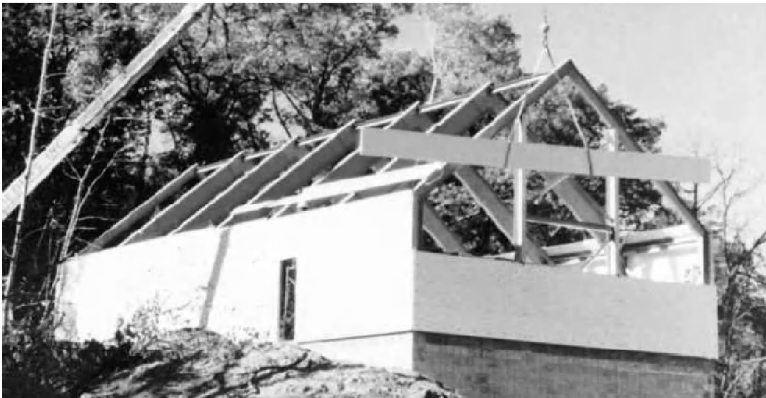
Figure 1.15 FRP gable frame structure under construction. (Courtesy of Strongwell.)
