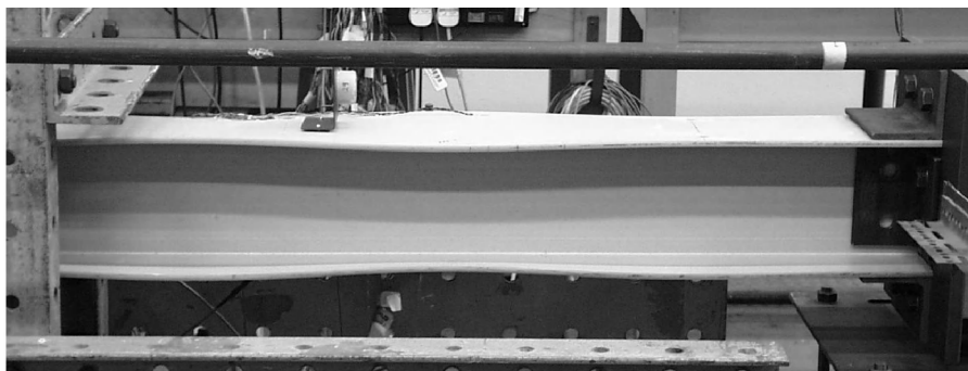
Figure 14.4 Local compression flange buckling in both flanges of a wide-flange pultruded profile subjected to axial load. (Courtesy of J. T. Mottram.)
