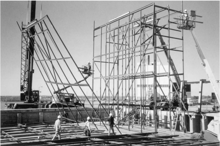
Figure 1.17 Stick-built cooling tower under construction. (Courtesy of Strongwell.)
