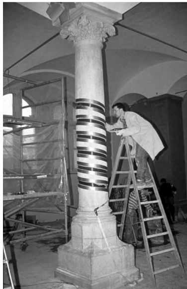
Figure 11.3 FRP confinement with a precured spiral-wound FRP strip. (Courtesy of Urs Meier.)
