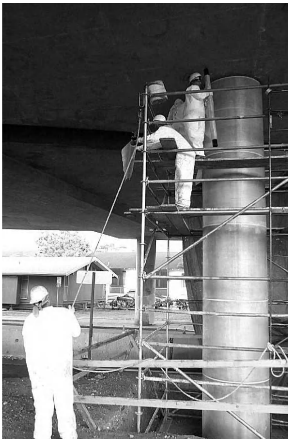
Figure 11.1 FRP system applied to a circular RC column. (Courtesy of Fyfe Company.)
