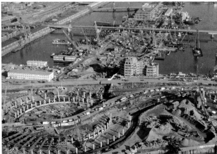
Figure 7.3 Aerial view of London Docklands Development.
