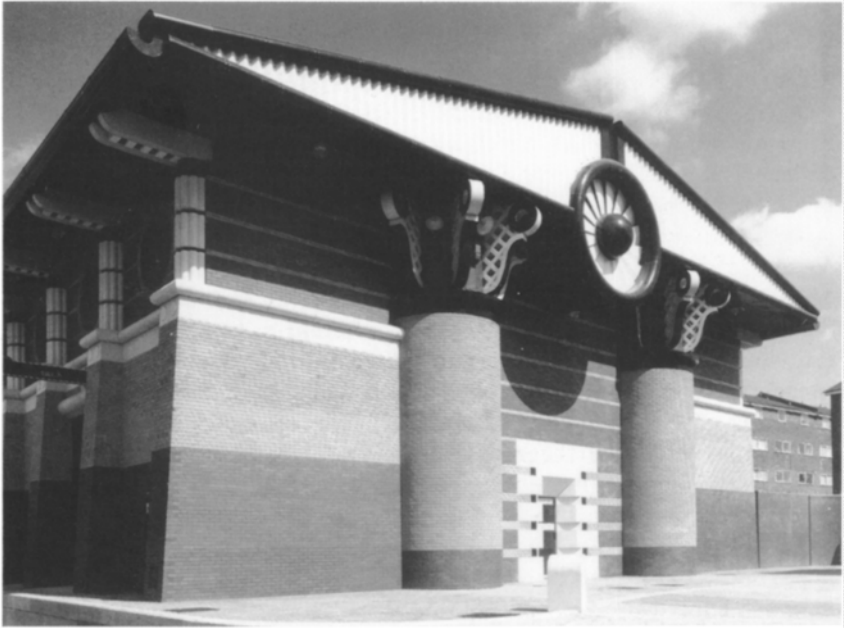
Figure 15.2 John Outram's Dockland Pumping Station, Isle of Dogs, London.
