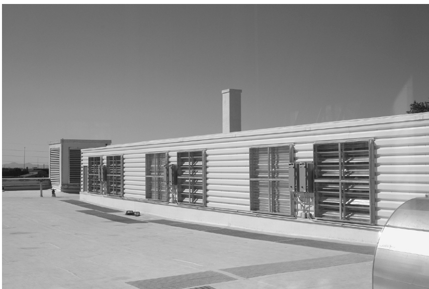
Figure 3.29. (a) The rotary fan at the top of the atrium of the Big D Construction office improves the thermal qualities of the building. (b) The automated relief air louvers work with the main mechanical systems to increase nighttime flush opportunities.
