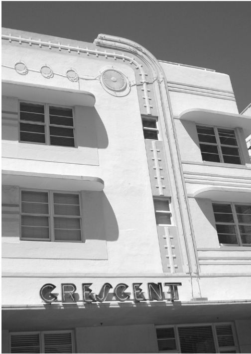
Figure 3.12. Sculptural form or even simple projecting shading devices were used to control sunlight. Windows could also be recessed to provide partial shading. Shown here are (a) the Crescent Hotel and (b) the Carlyle Hotel in Miami, Florida.
