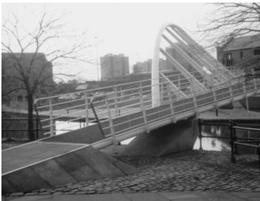
Figure 9.6 A new bridge across the Leeds-Liverpool canal, grant-aided by CMDC
