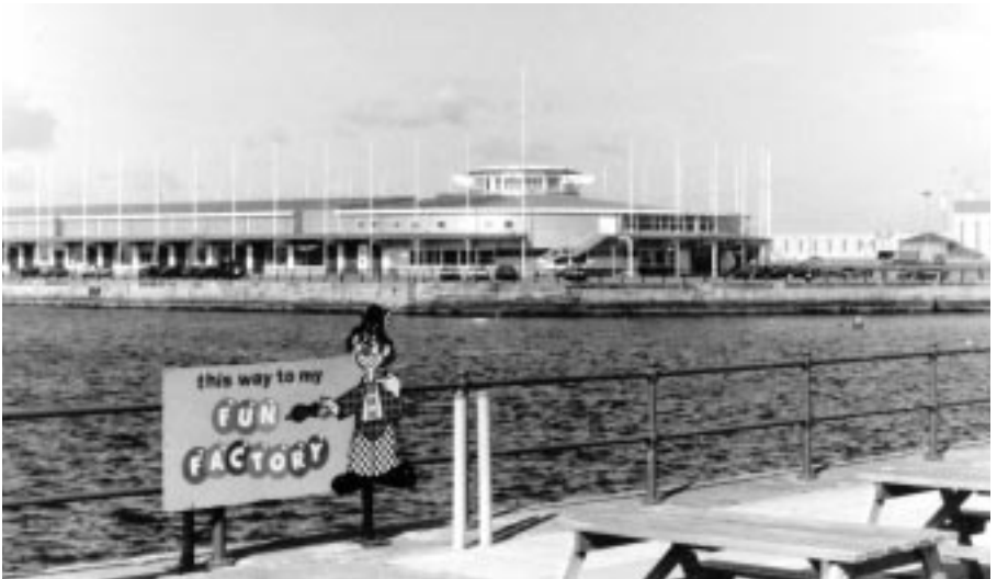
Figure 6.3 Jackson’s Landing – factory shopping development at Hartlepool Marina
