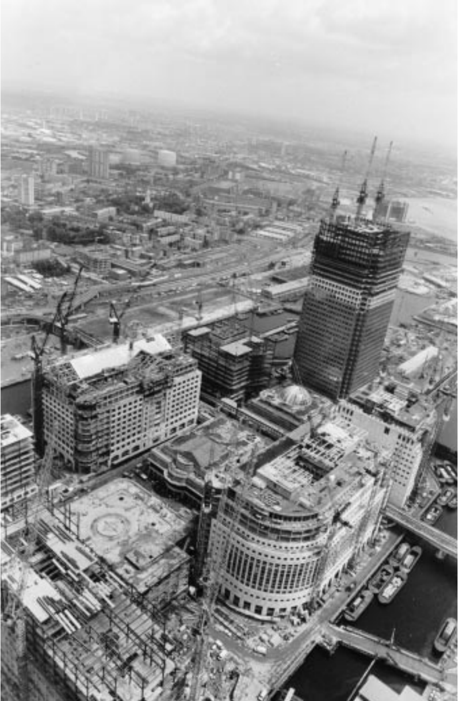
Figure 2.1 Canary Wharf under construction
