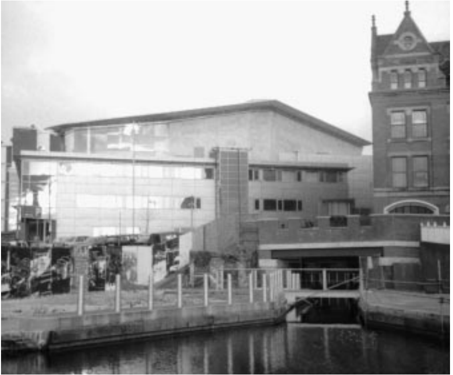
Figure 9.4 Riverside entrance to Bridgewater Hall, achieved by redirecting the canal
