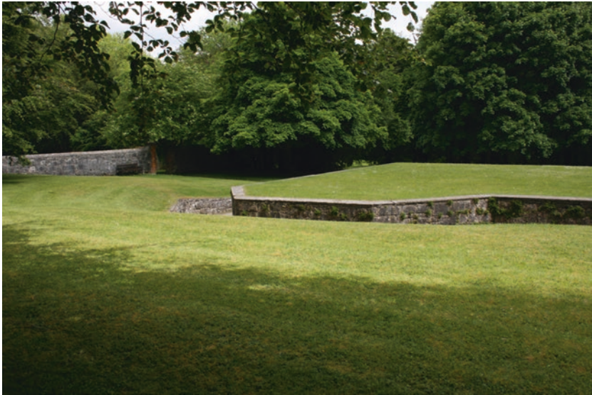
Fig. 2.3 The foundations of Coole Park, all that remains of the house today. Image credit: the author
