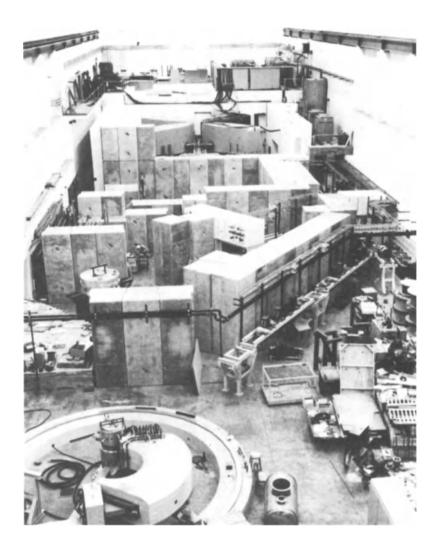
Fig. 5. Photograph taken in March, 1975 of the experimental areas looking south showing the magnetic spectrograph in the foreground, the 64 inch scattering chamber, and the main cyclotron in the background. The injector cyclotron is under the roof beams south of the main cyclotron, and the preinjector is behind the east wall in the separate ion-source room. The isotope production cave is underground outside the west wall.
