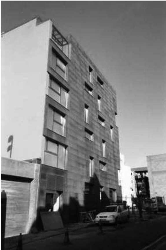
Plate 1. L1 20. (Rust-coloured façade, not discernible in a black-and-white photo)*. *Photo 1: L1 20 from log sheet: Flats and shop development for G. Gazzano and Sons, Farringdon Rd. Taken at 13:20 in late October 2004 this photo prompted discussion of how some modern architecture works sympathetically with the old.
