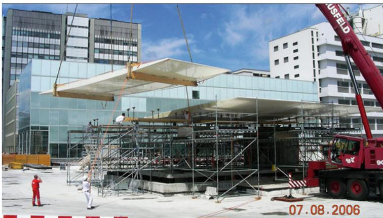
**Fig. 1.6** Roof assembly at construction site
