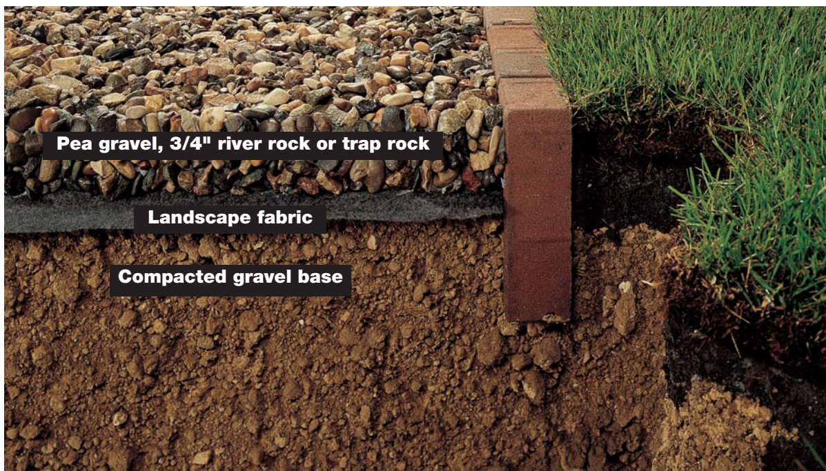
A thick layer of gravel set onto landscape fabric and a compacted gravel base makes an efficient and easily renewed floor.
