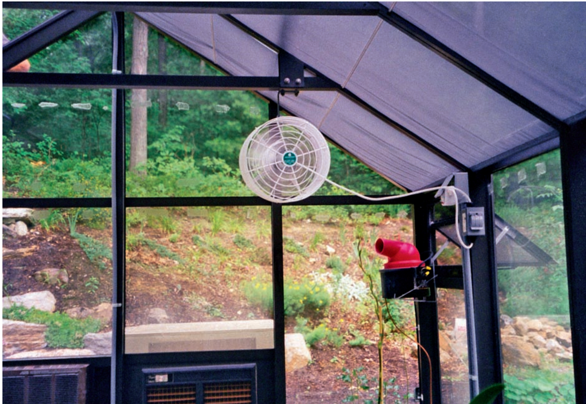
Roof shades, along with vents, help prevent a greenhouse from overheating in direct sunlight. Here, a combination of circulating fans and cloth shades mounted on the interior of the south-facing glass helps protect plants.
