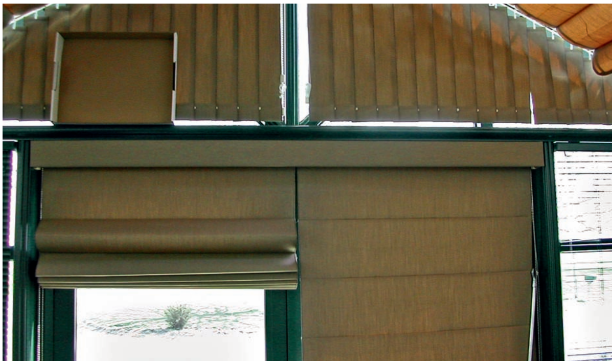
Louvered and roll-up shades help to block the sun in this greenhouse.
