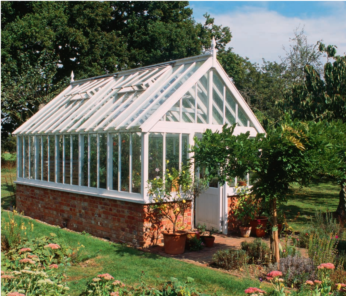
A greenhouse is composed of several major systems that perform important functions. When planning your greenhouse, you'll need to make choices about each system, which include the foundation, floor, frame, glazing, ventilation, watering, heat, storage and more.
