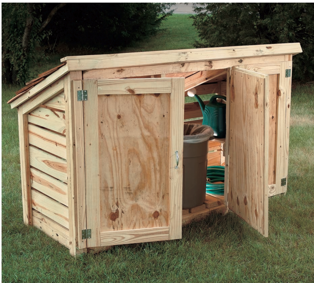
This utility shed is so small it's practically portable, but it succeeds in design because it has classic shed features, like the slightly sloping shed-style roof.
