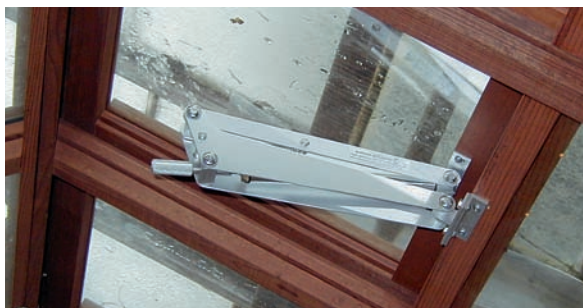
Automatic openers sense heat build-up and open vents.
