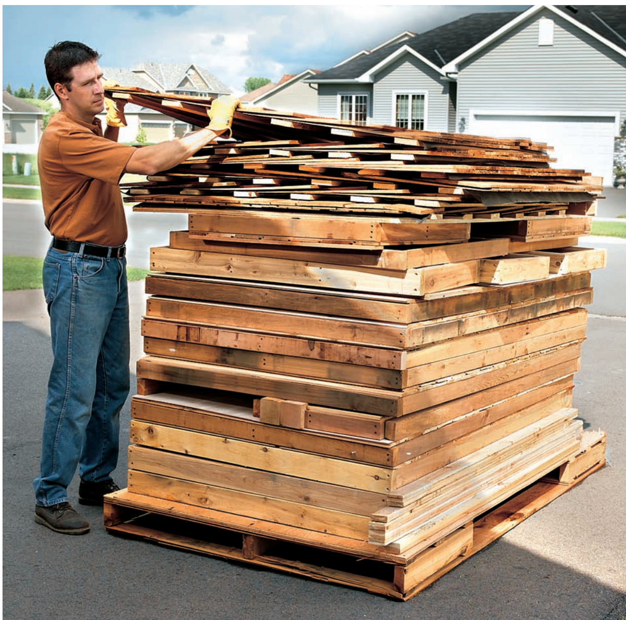
Some shed kits, such as this panelized cedar shed kit, are delivered directly to your house partially assembled and packed on pallets.
