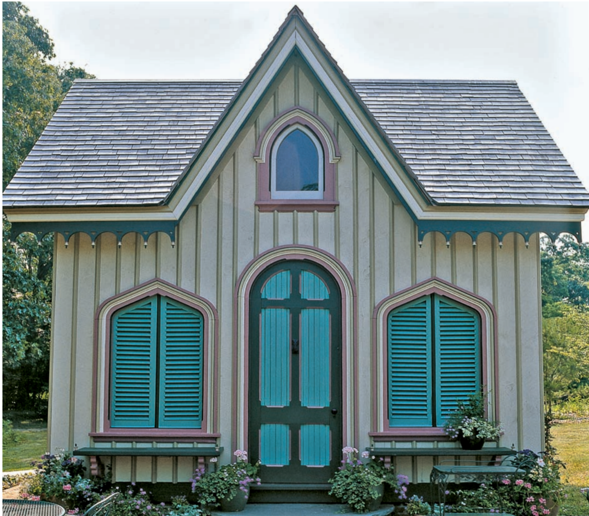
Kit sheds usually come with prehung doors and windows that are easy to install; they are typically major elements of the shed design.
