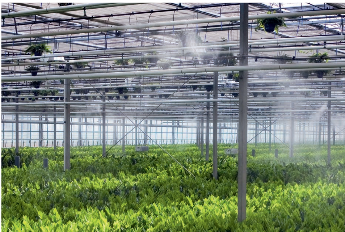
Misting systems restore the ambient humidity that is released when greenhouse vents open during the heat of the day. A humidistat monitors moisture levels and controls the misting system.
