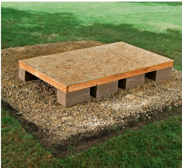
Landscape blocks or pavers can be bonded together with construction adhesive and stacked on a well-drained, sturdy base to create a raised foundation for building a shed.
