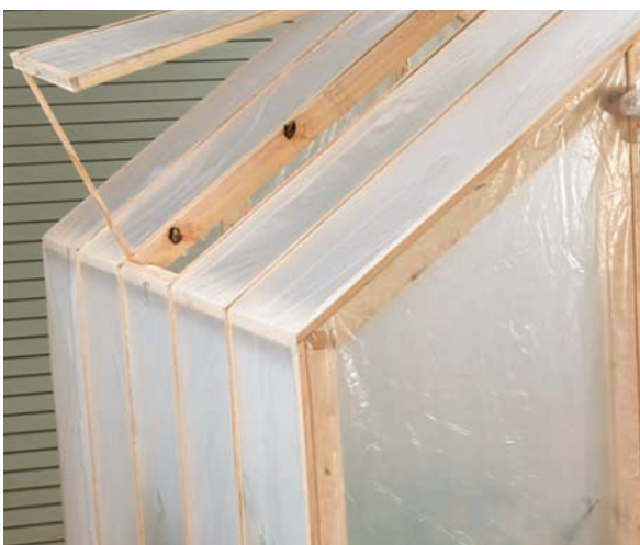
A wood frame with plastic glazing
