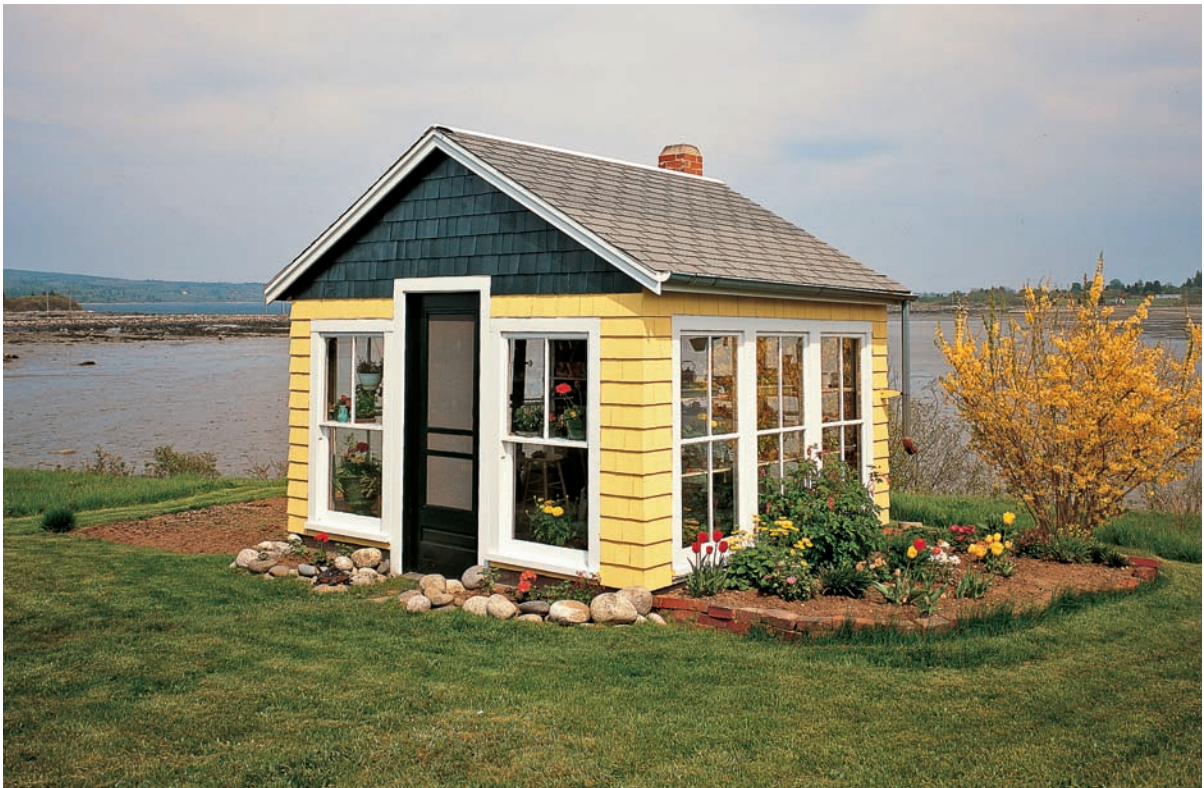
Because its floor plan is less than 100 square feet (9.2 sq.m) in area, this shed did not need a building permit (and fee) to be built. Exact thresholds between size and permit requirements are established by your municipality.
