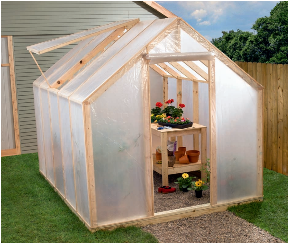
A wood-frame greenhouse with sheet-plastic cover is an inexpensive, semipermanent gardening structure that can be used as a potting area as well as a protective greenhouse.
