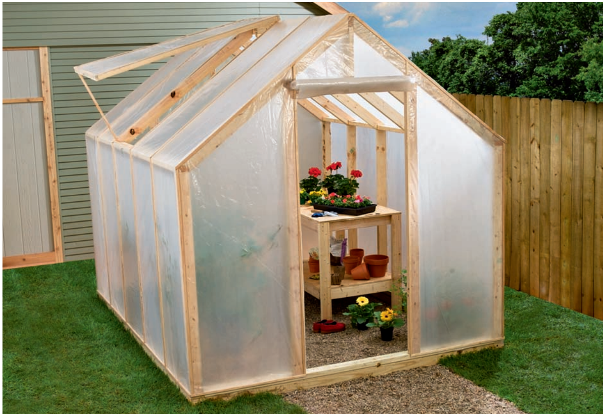
An A-frame greenhouse is easy to design and build yourself with just some wood and sheet plastic. See page 114.
