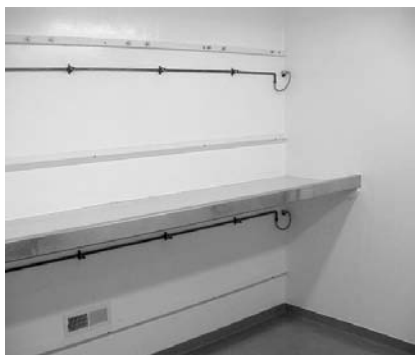
Figure 9.1 Nonhuman primate animal room. Floors and walls are made of nonporous materials that are readily sanitized. Watering systems are typically automatic.
