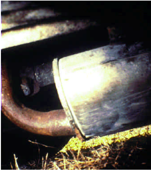
FIGURE 9.57 The tailpipe was bent up to fit into the hole.
