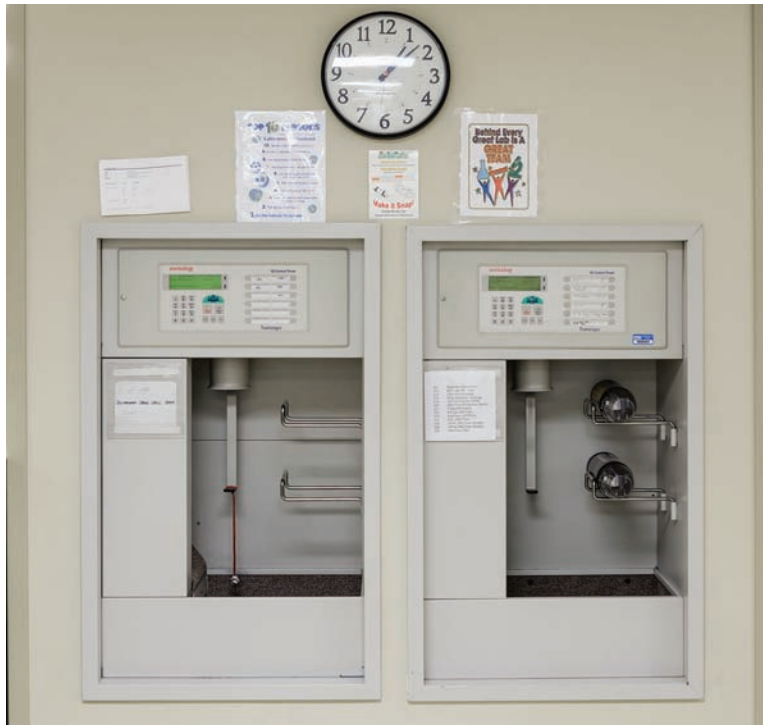
FIGURE 16-5 Pneumatic tube systems carry samples within a network of tubes.
